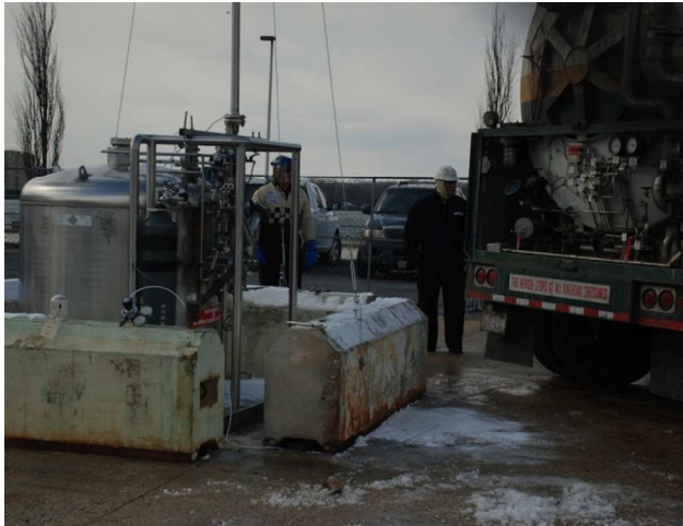
Figure 2. 1000-liter liquid hydrogen dewar at NRL being fueled by a commercial vendor.
