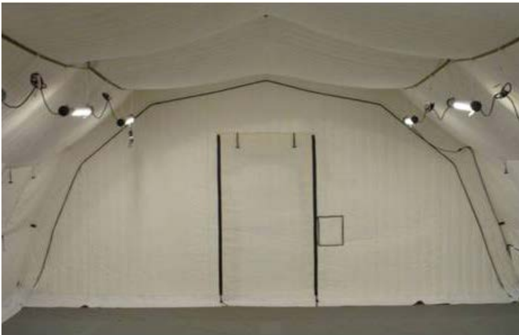
Figure 2-3. HDT global airbeam shelter with nonwoven composite insulation (Thinsulate™) liner.
