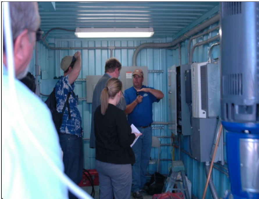
ARO Personnel viewing the Wash System in operation and Pump Station
