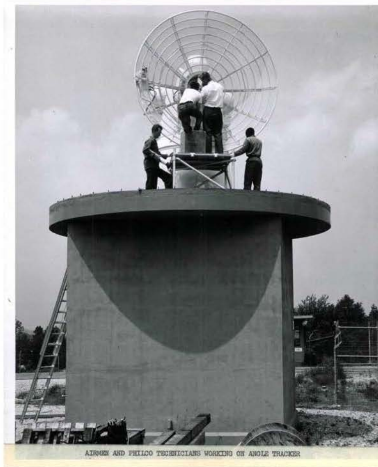
Historic View of Airmen and Philco Technicians Working on Angle Tracker Antenna (NBAFS 1961)
