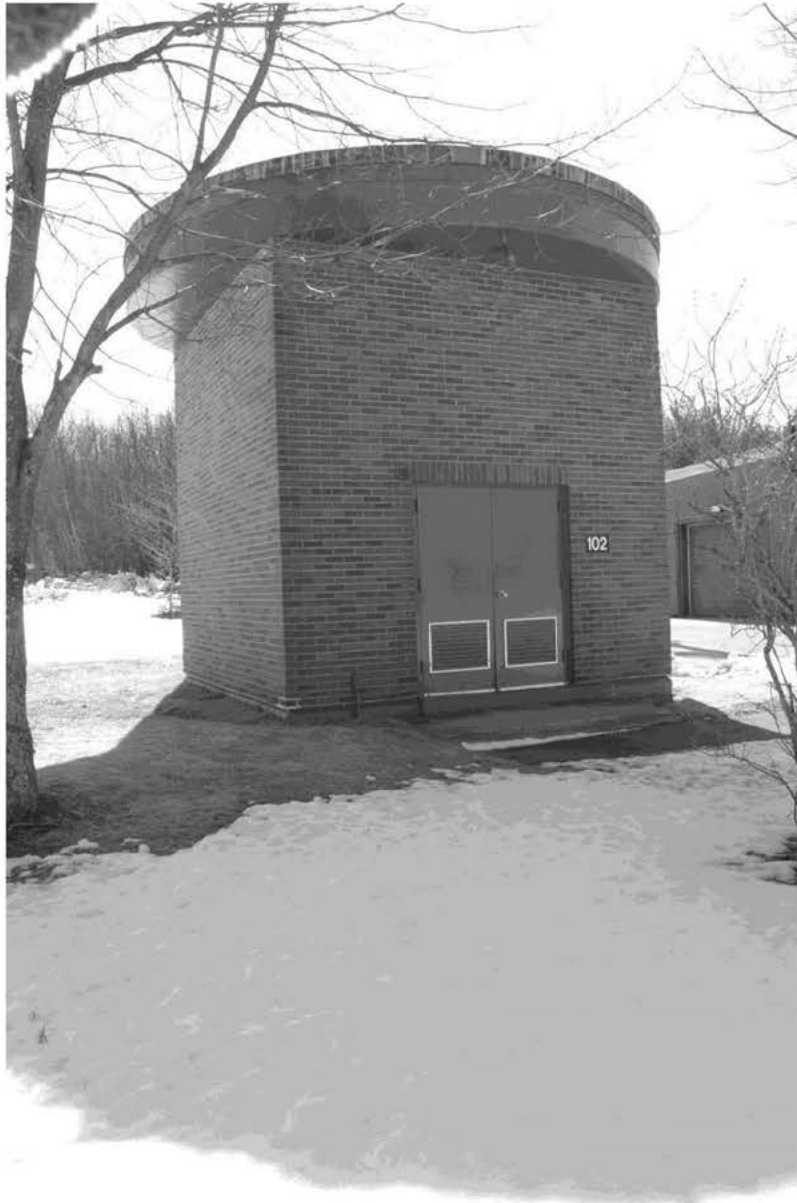
NH-51-B-1 BUILDING 102, LOOKING SOUTHWEST.
