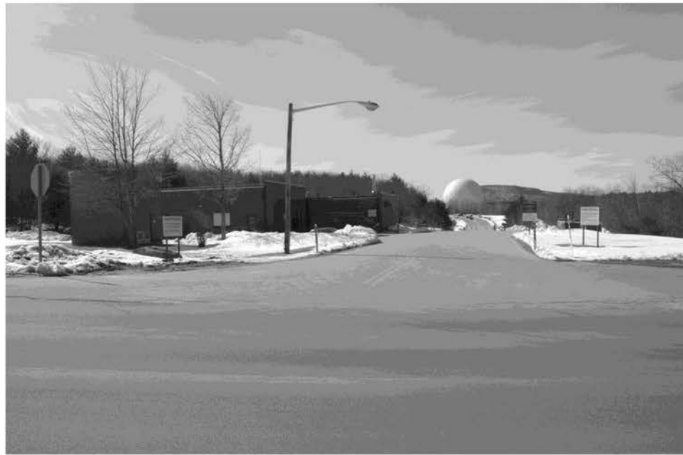
NH-51-B-3 BUILDINGS 102 AND 103, LOOKING WEST.
