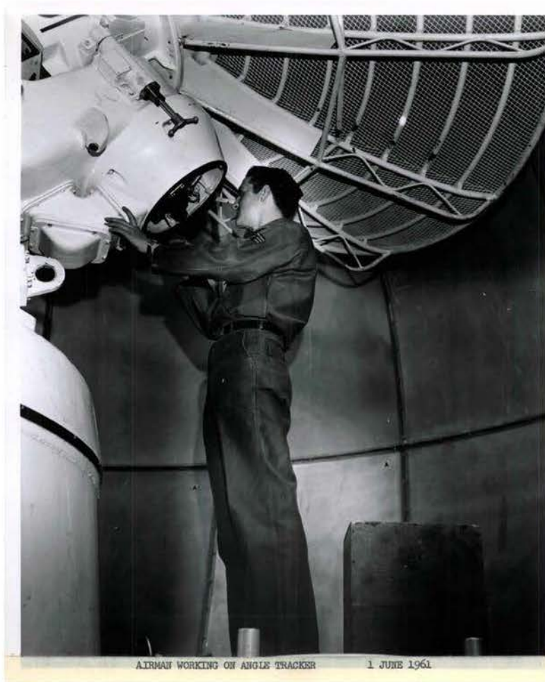
Historic View of Airman Working on Angle Tracker Antenna (NBAFS 1961)
