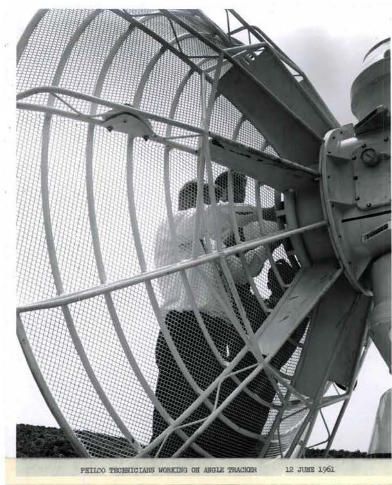
Historic View of Philco Technicians Working on Angle Tracker Antenna (NBAFS 1961)
