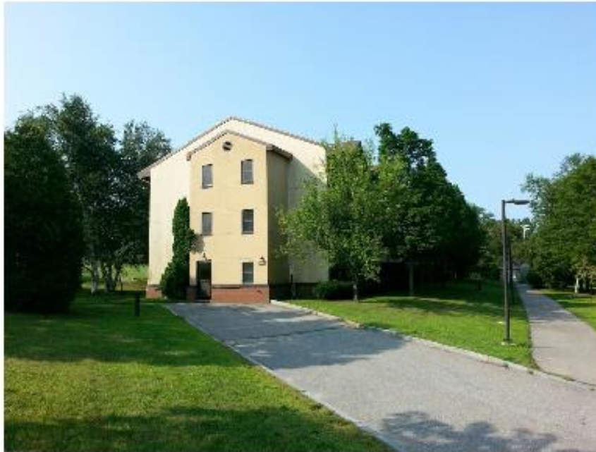
Building 1510 – View from East
