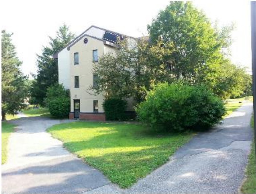
Building 1511 – View from West
