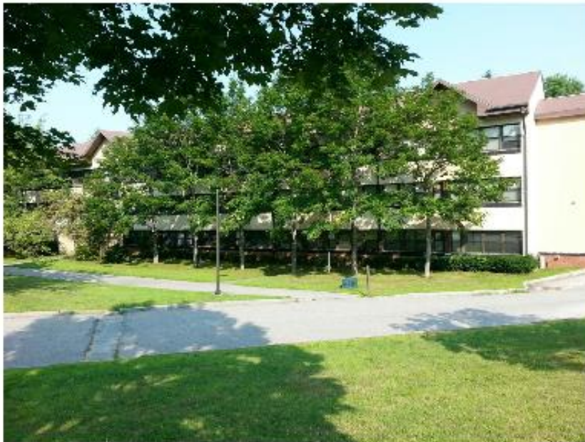
Building 1511 – View from Southeast
