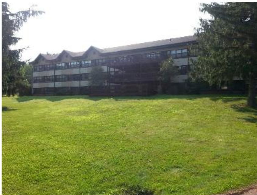
Building 1511 – View from North
