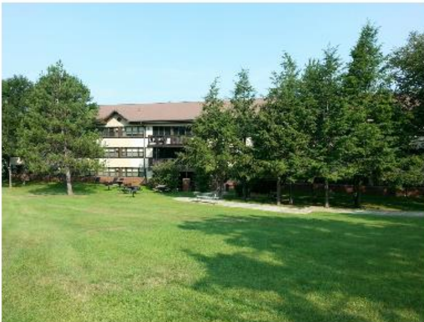
Building 1510 – View from South
