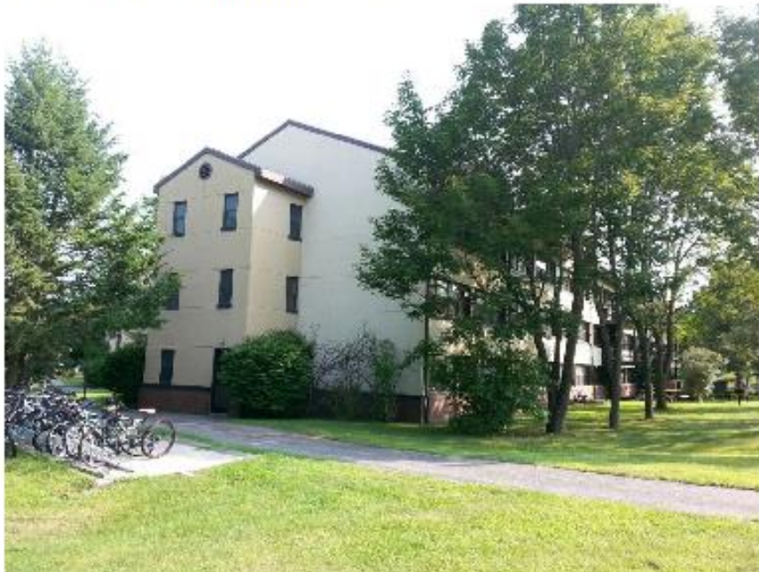
Building 1510 – View from West
