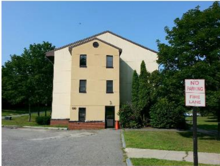
Building 1511 – View from East
