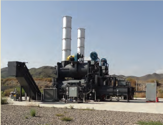
Photo 1 - Two 8-Ton Capacity Incinerators at FOB Salerno
