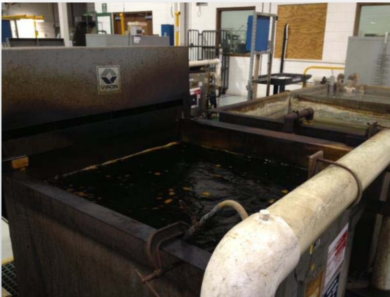
Tank E-2 – Shop 62722
