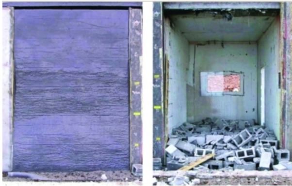
Fig. 3. The coated wall does not suffer any serious damage while the uncoated wall is broken completely exposing the interior.
