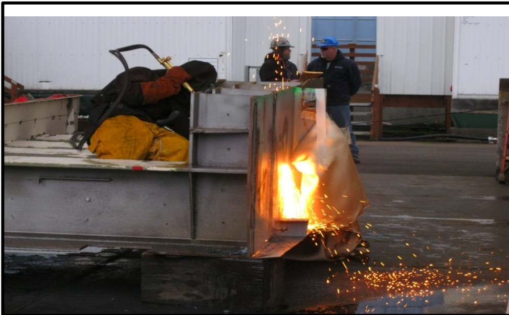
Figure 7: Ex-CGN-9 Deck Section. Photograph by Danny Schroedle.
