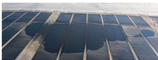
Figure-17: Site II (NAS Patuxent River) water ponding.
