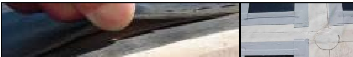
Figure-13: Bonding failure (left) and tape solution (right) between PVL and PVC at Site I (Luke AFB).
