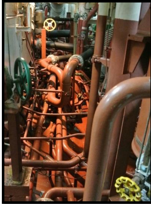
Figure 1 - Complex, space constrained fleet piping
