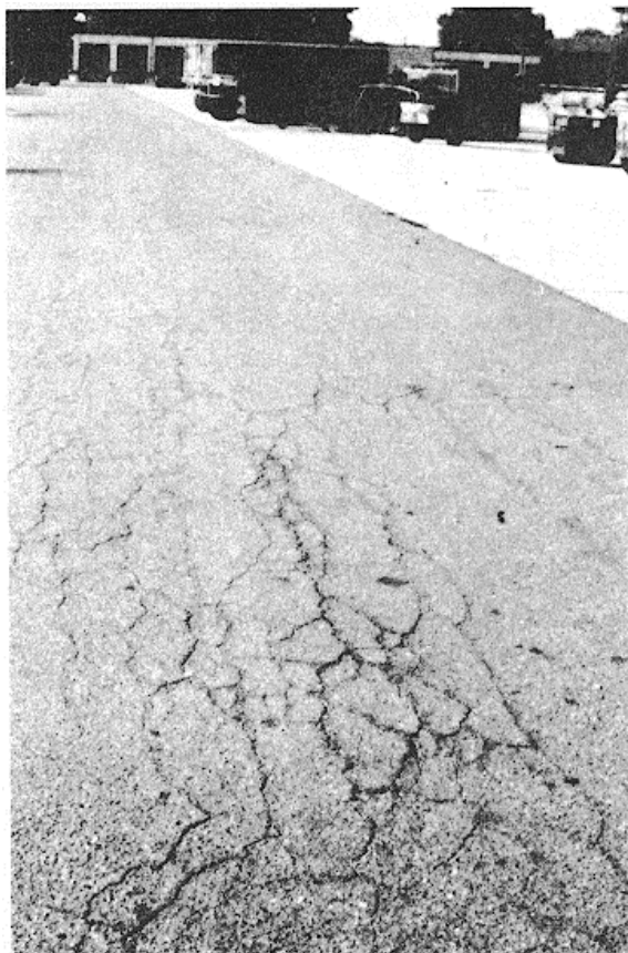
Figure 2 - Medium Severity Alligator Cracking
