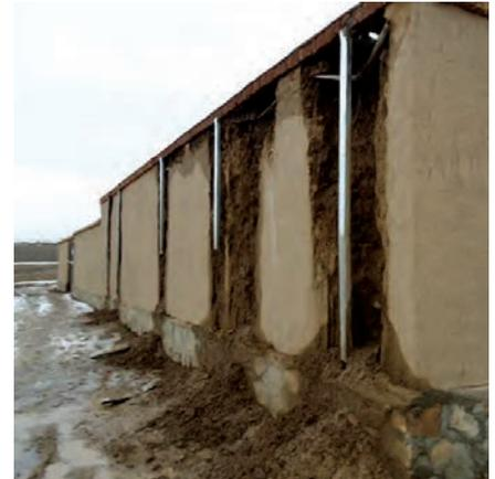
**Defective materials and construction methods**, as well as poor planning and oversight, were responsible for the exterior deterioration of the dry-fire range, which was caused by water penetration and required that the facilities be rebuilt. (NPTC photo)
