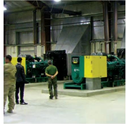
**SIGAR's inspection found that generators,** like those pictured, were improperly connected to a transformer, causing damage to two transformers. (SIGAR photo by Brian Flynn)
