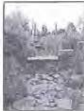
A rain garden manages runoff from impervious surfaces such as roofs and paved areas.
