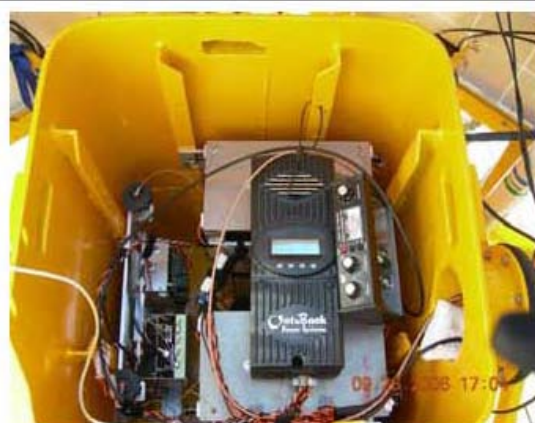
Figure 2: Inside view of the electronics box for the bistatic transmitter buoy.
