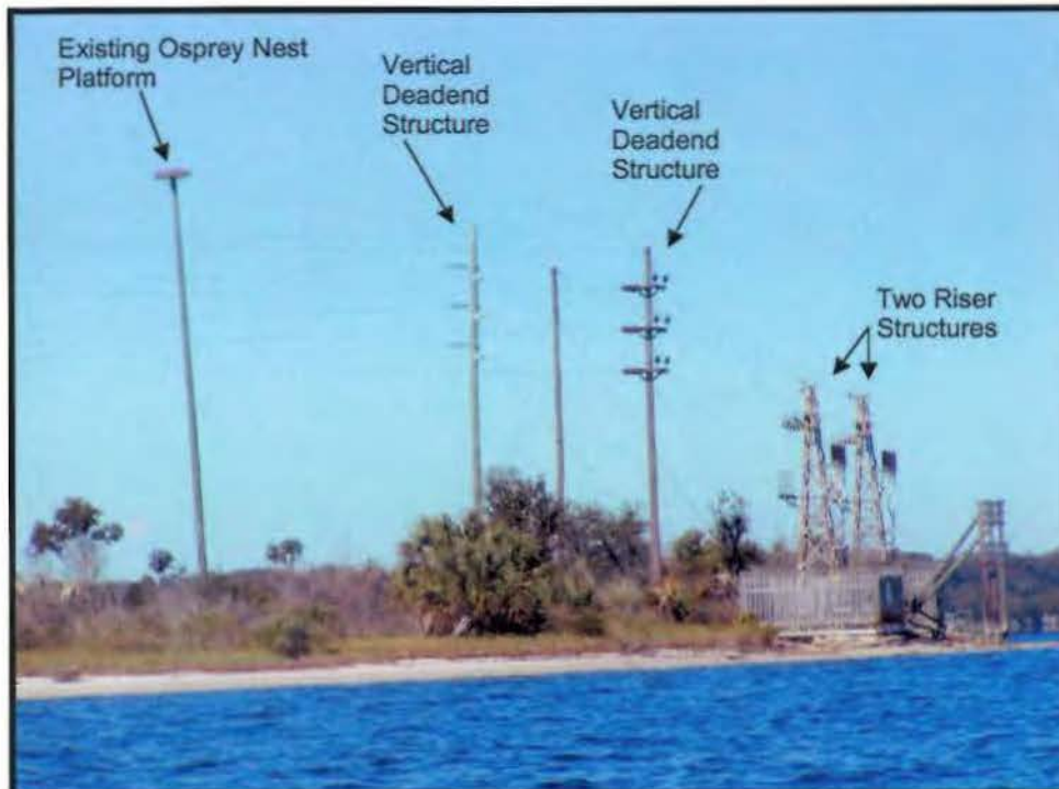
Photo 3 Existing 46kV Transmission Line, Associated Equipment Structures, and Osprey Nesting Platform at Military Point (Location #2 on Map 1)
