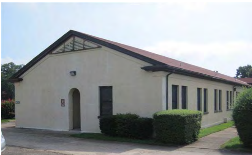
Maxwell facility # 902 is proposed for demolition
