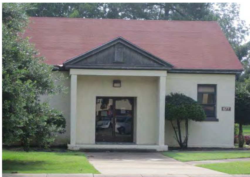
Maxwell facility #677 is proposed for demolition
