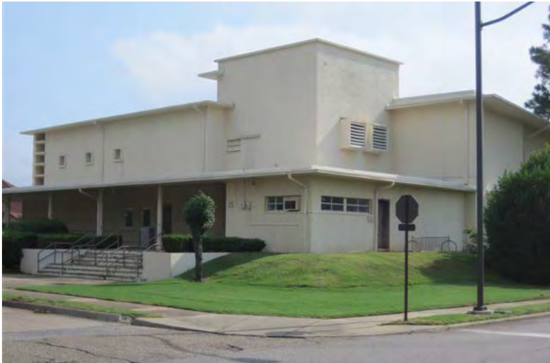
Maxwell Facility #26, Base Theater Proposed for Demolition
