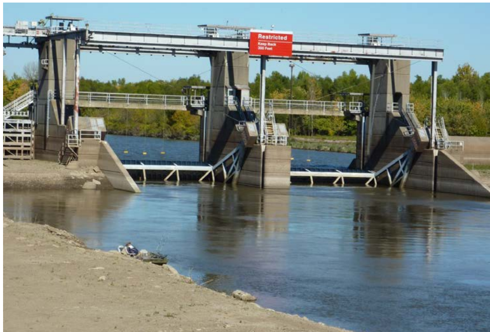
Figure 7. Site of third field test, Kaskaskia Lock and Dam, Illinois.
