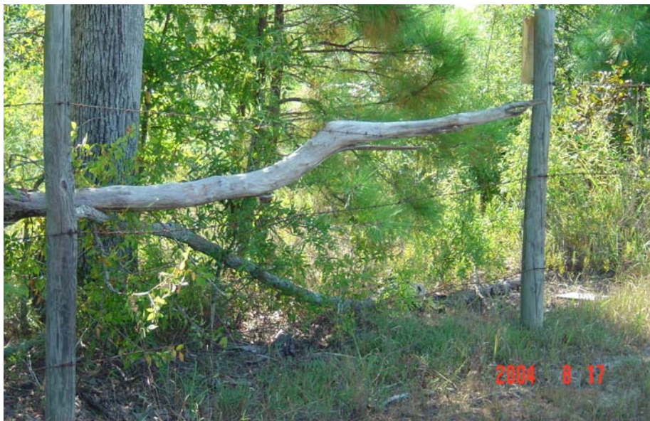
Photo 4: Corroded Perimeter Fence
