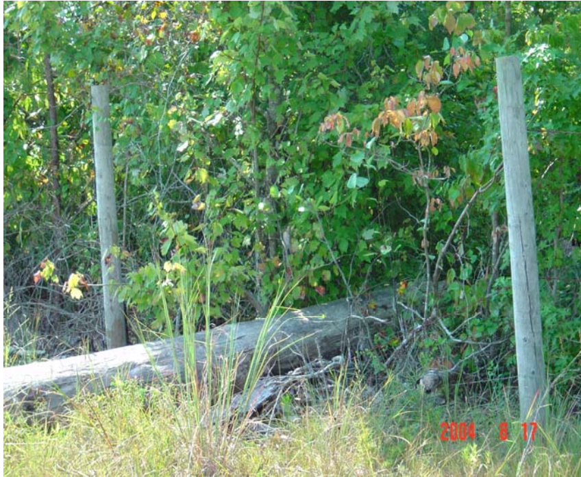
Photo 5: Damaged Perimeter Fencing Section
