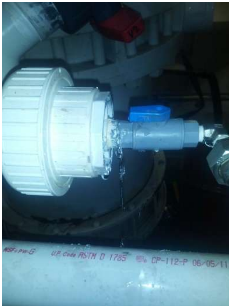
Figure 11. Cracked nipple on the p3SFS leading to the drip sampler.
