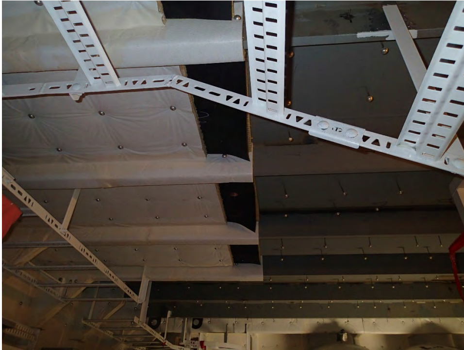
Sally Ride Aux Machinery Overhead
