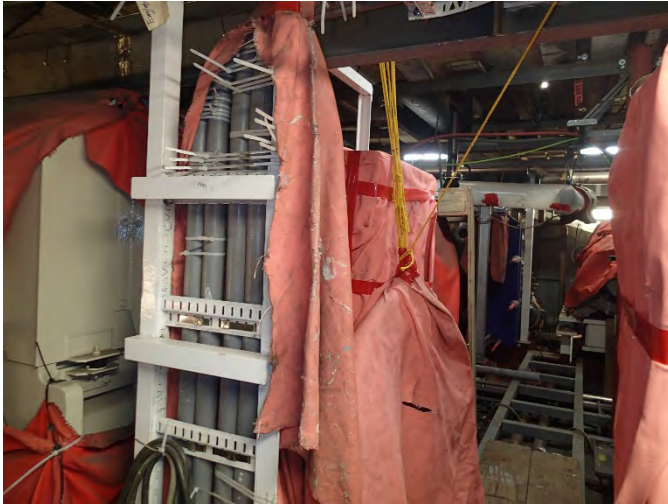
Sally Ride 23 October 2014 No2 Generator
