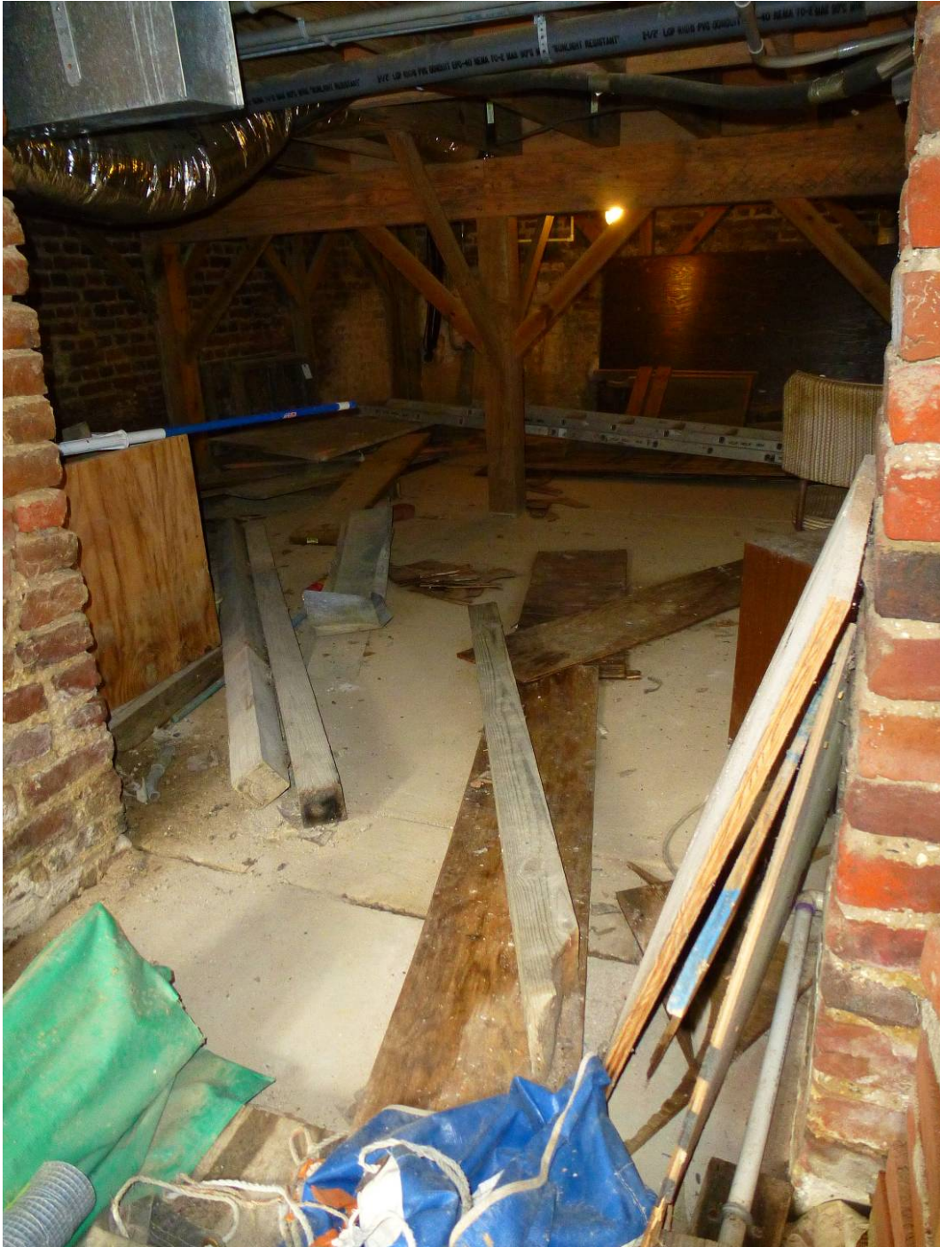
Figure 155. Newer wood support members in the cellar (ERDC-CERL, 2012).
