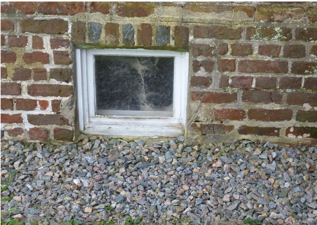
Figure 114. Single-pane cellar window (ERDC-CERL, 2012).
