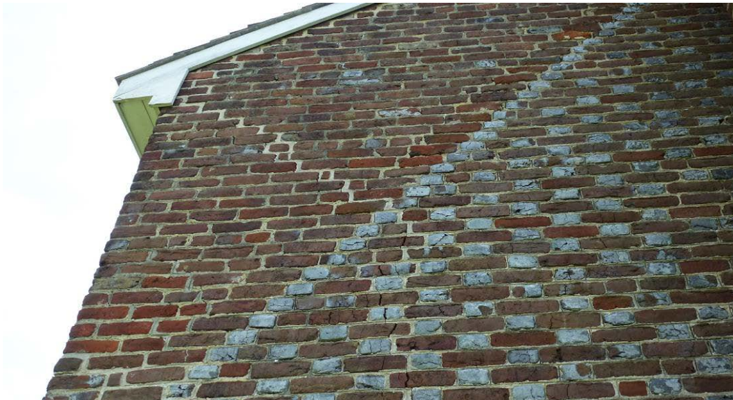
Figure 52. The ca. 1730 all-glazed brick header is still evident below the strikingly different 1893 brickwork (ERDC-CERL, 2012).
