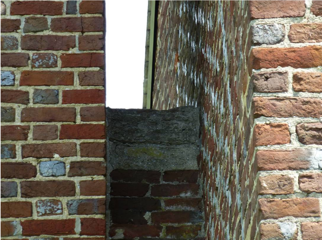
Figure 72. Connection between the chimney and main block (ERDC-CERL, 2012).
