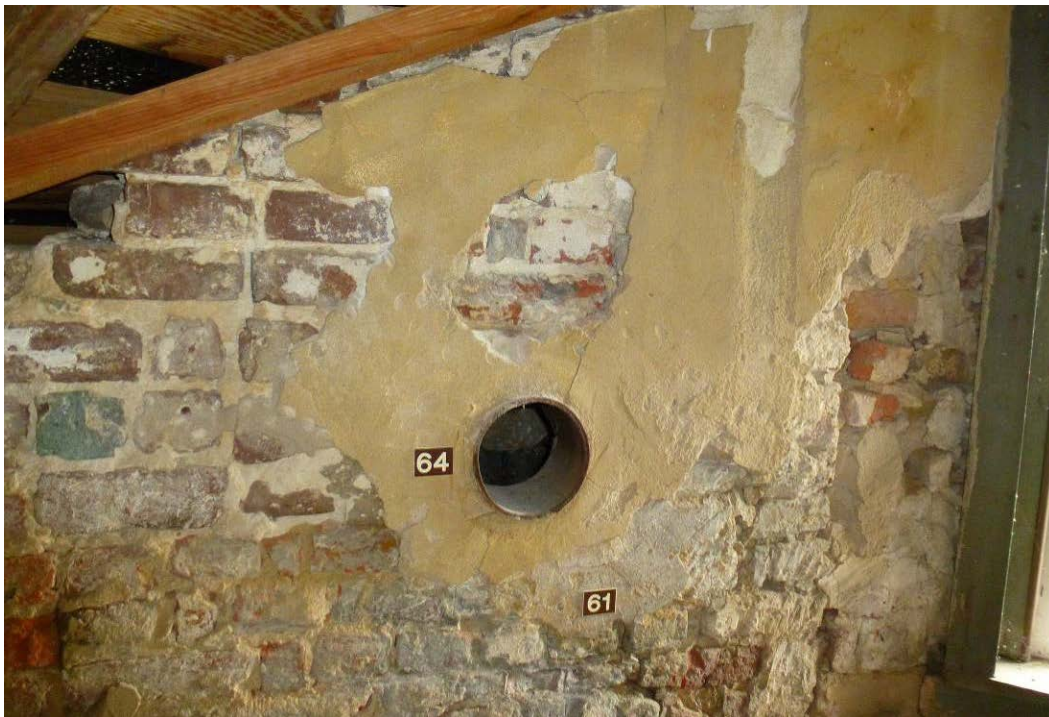
Figure 142. Stove thimble that was added in 1893 in the shed room (rear chamber) addition (ERDC-CERL, 2012).
