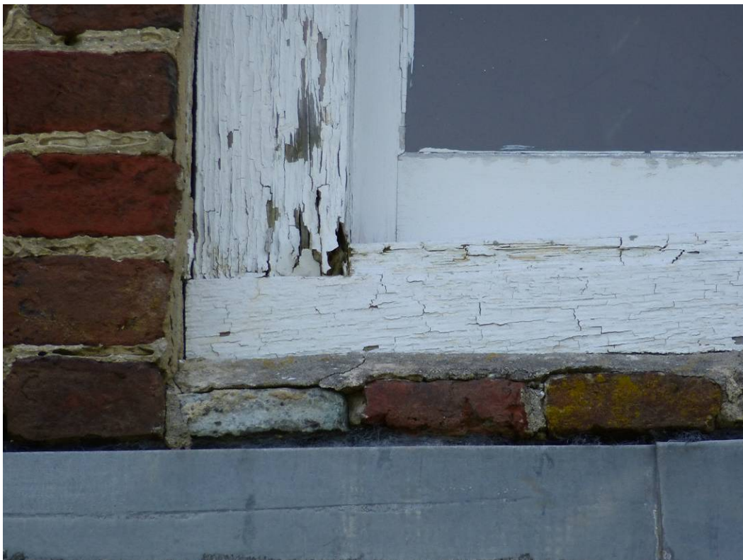
Figure 116. Detail of a damaged wood window frame (ERDC-CERL, 2012).
