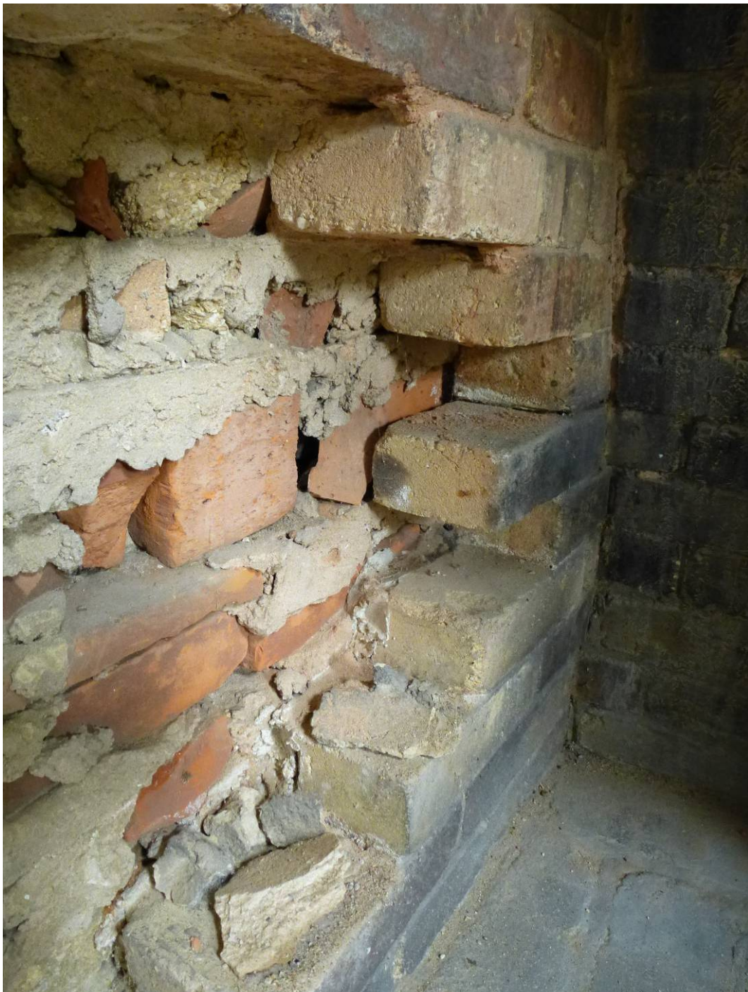
Figure 137. Brick infill when fireplace was converted to a stove, northwest hall fireplace (ERDC-CERL, 2012).
