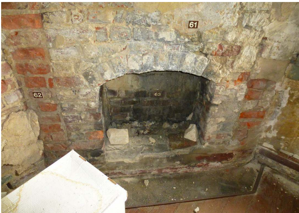
Figure 141. A third fireplace and chimney were constructed when the shed room (rear chamber) was added in Period II (ERDC-CERL, 2012).
