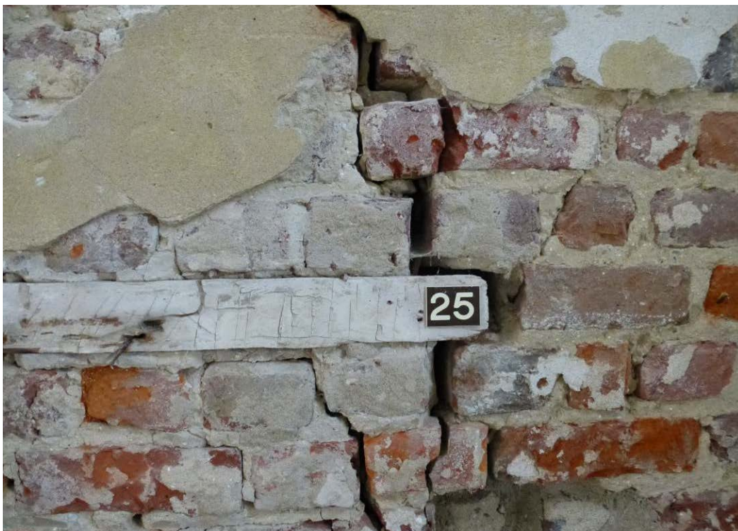
Figure 136. Large crack in brickwork around hall fireplace (ERDC-CERL, 2012).
