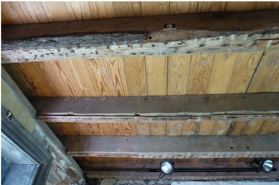
Figure 156. Ceiling joists in the Tower are some of the last remaining eighteenth-century framing in the house (ERDC-CERL, 2012).
