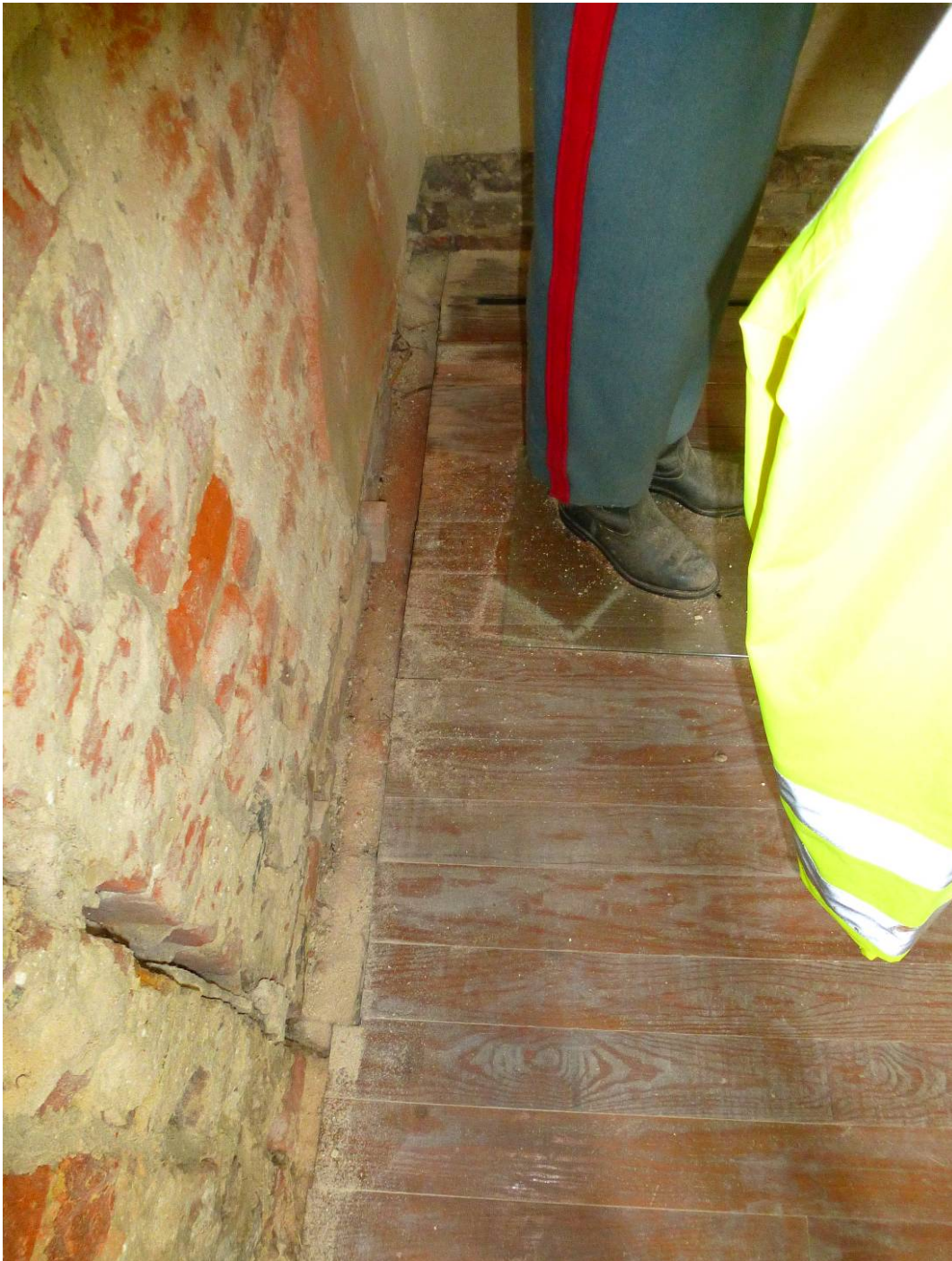
Figure 199. Gap between floor boards and brick wall where the baseboard and the shoe molding have been removed (ERDC-CERL, 2012).
