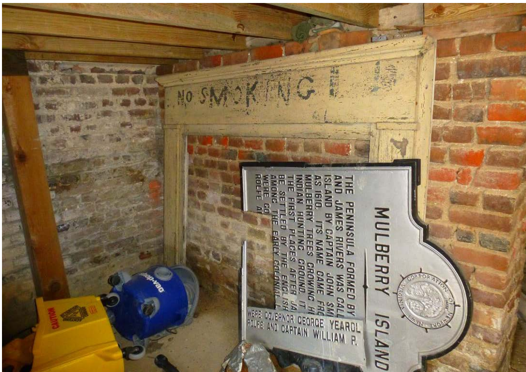
Figure 172. One of the original 1893 wood mantel (from first-floor hall) is being improperly stored when propped against a damp brick wall in the cellar (ERDC-CERL, 2012).
