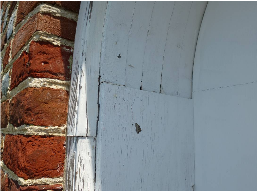
Figure 103. Glued arched jamb of the front door (ERDC-CERL, 2012).
