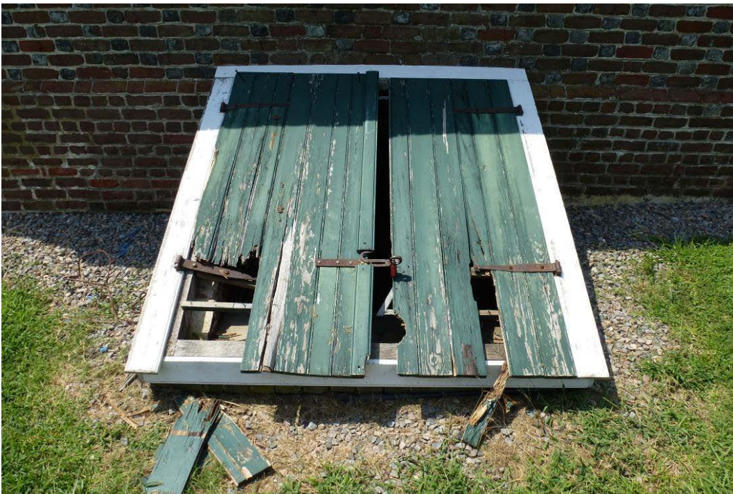
Figure 106. Damaged wood cellar doors have been replaced since this photograph was taken (ERDC-CERL, 2012).
