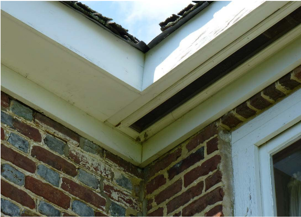
Figure 124. Underside of the wood soffit where vents have been cut in to provide attic ventilation (ERDC-CERL, 2012).
