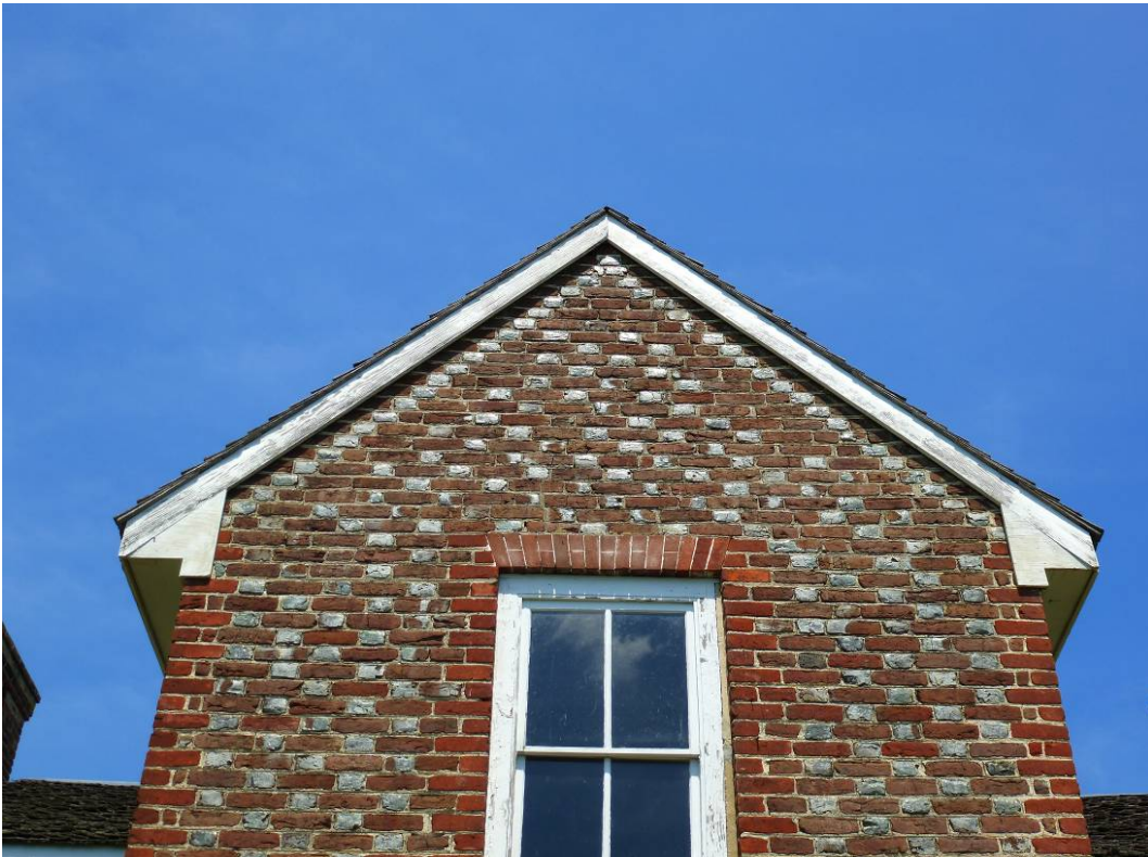
Figure 120. View of rakeboard on the southwest elevation of the porch tower (ERDC-CERL, 2012).
