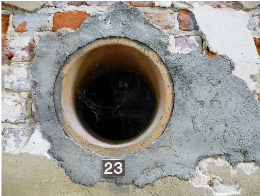
Figure 138. A stove thimble was added shortly after the 1893 remodeling to the northwest chimney (ERDC-CERL, 2012).
