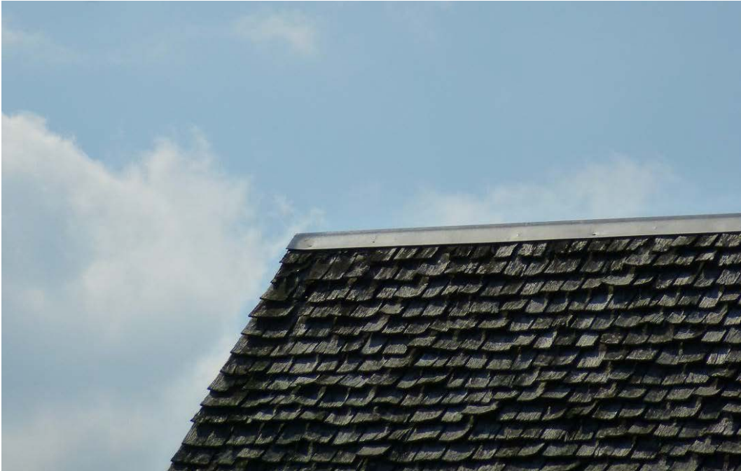
Figure 95. Metal ridge piece along gable of main block (ERDC-CERL, 2012).
