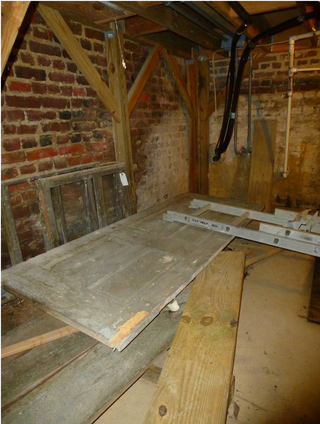
Figure 209. Doors that have been removed and are being stored should be stored in a dry place, unlike this one which is lying on the cellar floor (ERDC-CERL, 2012).
