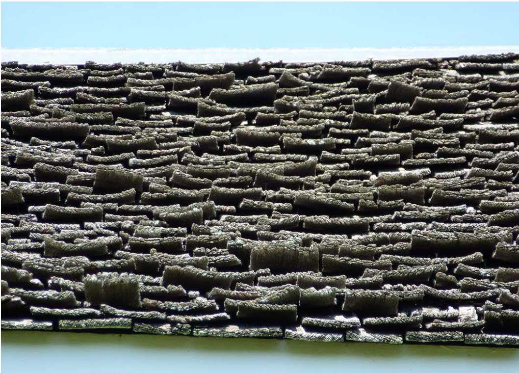
Figure 89. Cupping of the wood shingles, uniformly across entire roof (ERDC-CERL, 2012).
