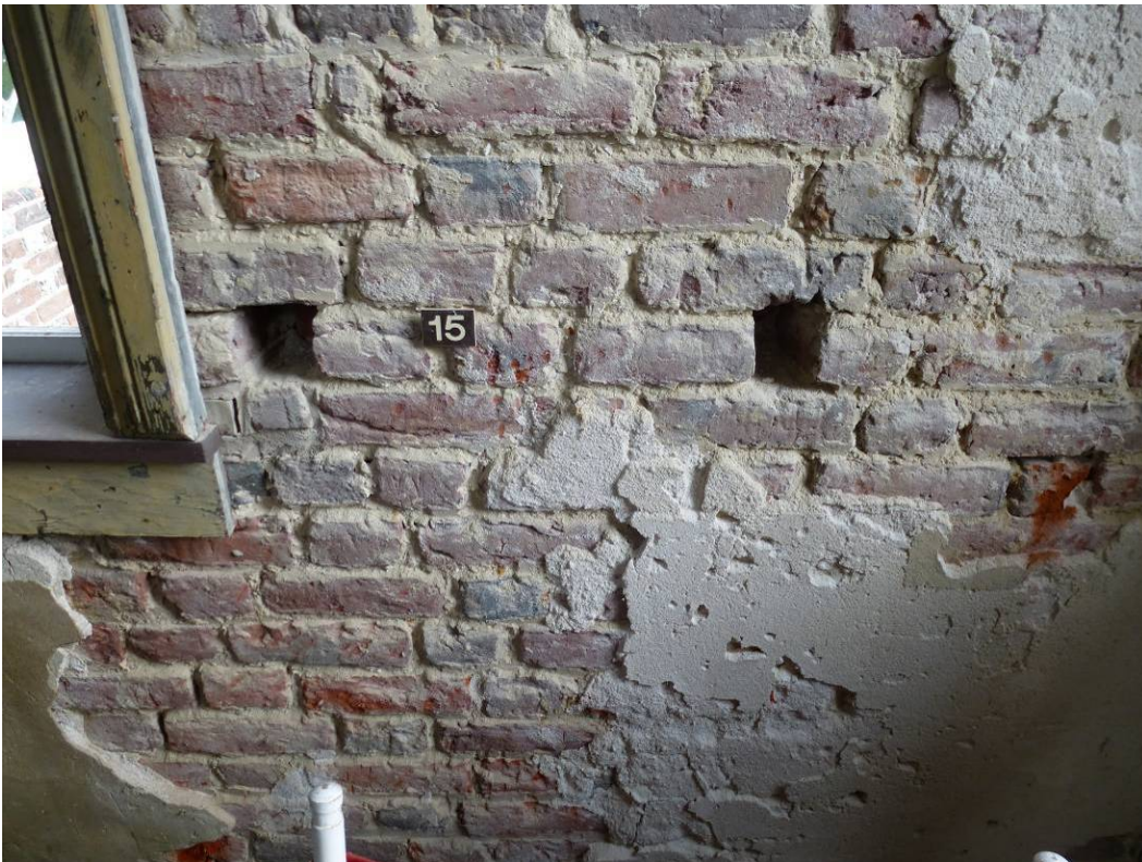
Figure 150. Holes in the brickwork around the perimeter of the hall were for chair board blocking ; when the frame walls were replaced with brick ca. 1730, wood blocks were installed to carry a chair board (ERDC-CERL, 2012).
