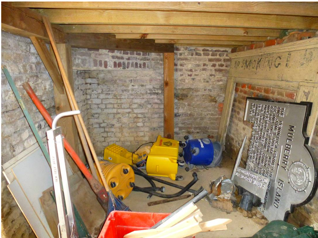
Figure 144. Looking at the southeast wall of the cellar and the corbelled base for the shed room (rear chamber) chimney (ERDC-CERL, 2012).
