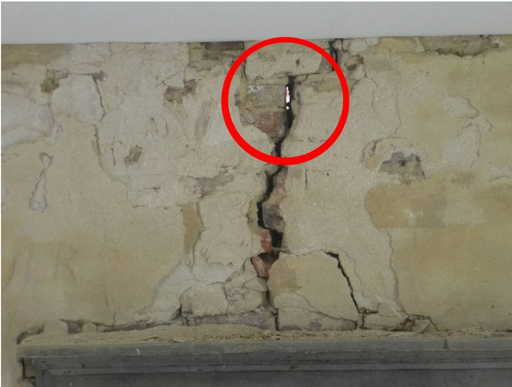
Figure 151. Structural crack above the fireplace on the northwest wall circled in red (ERDC-CERL, 2012).
