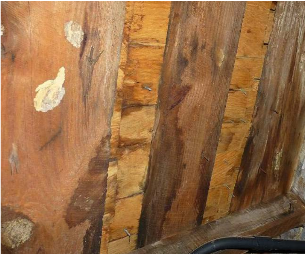
Figure 96. Underside of the wood shingles showing protruding nails and wet roofing members (ERDC-CERL, 2012).
