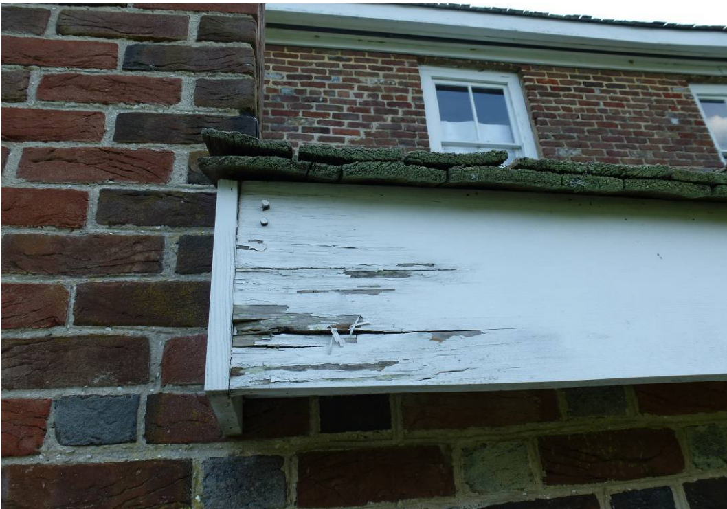
Figure 123. Damaged rakeboard on the northeast side of the shed room (rear chamber) (ERDC-CERL, 2012).
