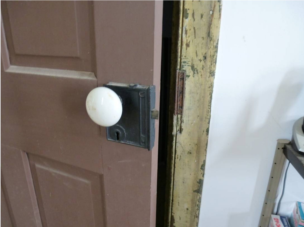
Figure 182. Typical door hardware with painted knob (ERDC-CERL, 2012).
