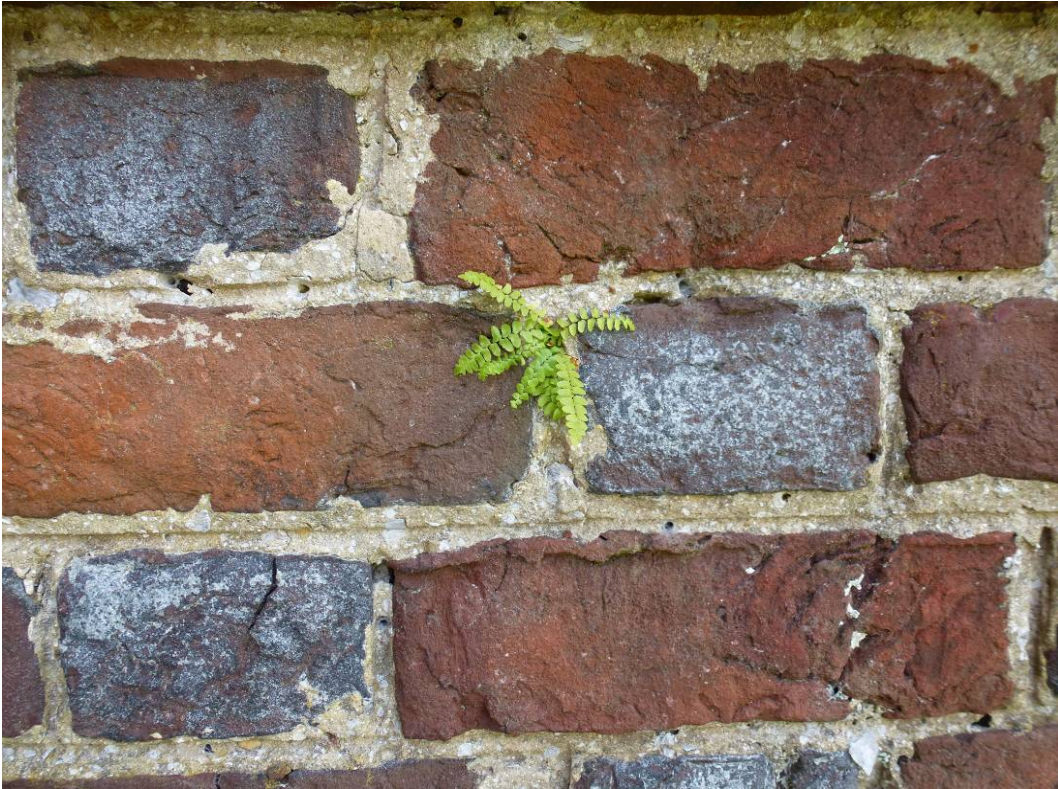
Figure 63. Vegetation growth within brickwork (ERDC-CERL, 2012).
