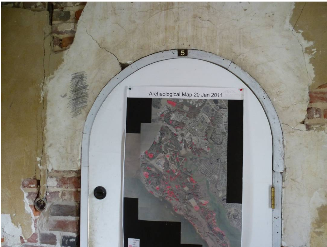
Figure 203. The laminated arched door jamb trim is virtually the only trim from the eighteenth century to survive in the house (ERDC-CERL, 2012).
