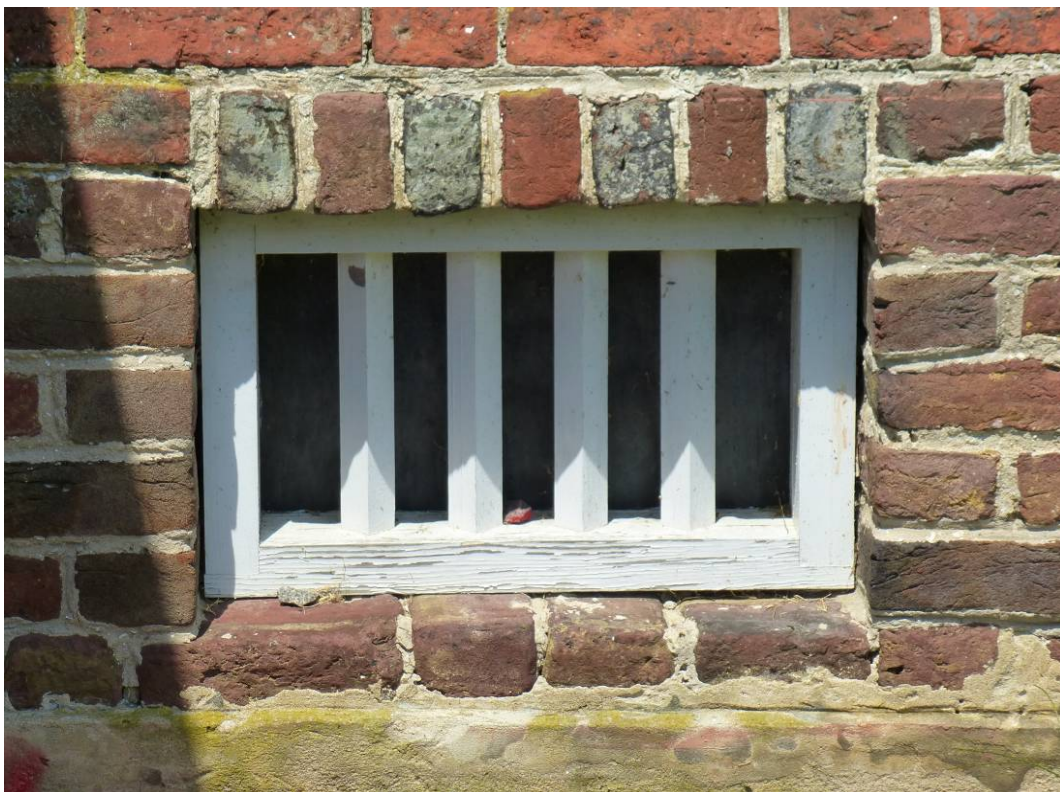
Figure 126. Wood-louvered vent on the southeast elevation that is blocked from the basement side (ERDC-CERL, 2012).
