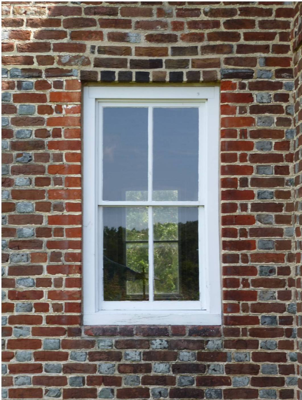
Figure 112. First-floor Period III window that needs to be replaced with an accurate Period II window (ERDC-CERL, 2012).
