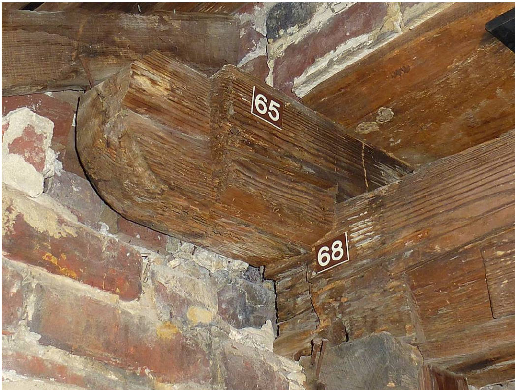
Figure 29. Original end joists (#65) along with other wood structural members in the Matthew Jones House should be maintained and preserved (ERDC-CERL, 2012).
