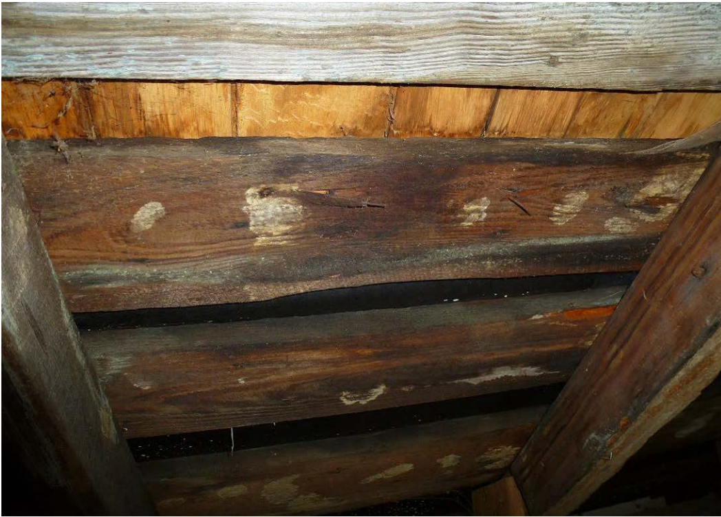
Figure 97. Moisture-soaked roofing members including joists, rafters, and wood shingles (ERDC-CERL, 2012).
