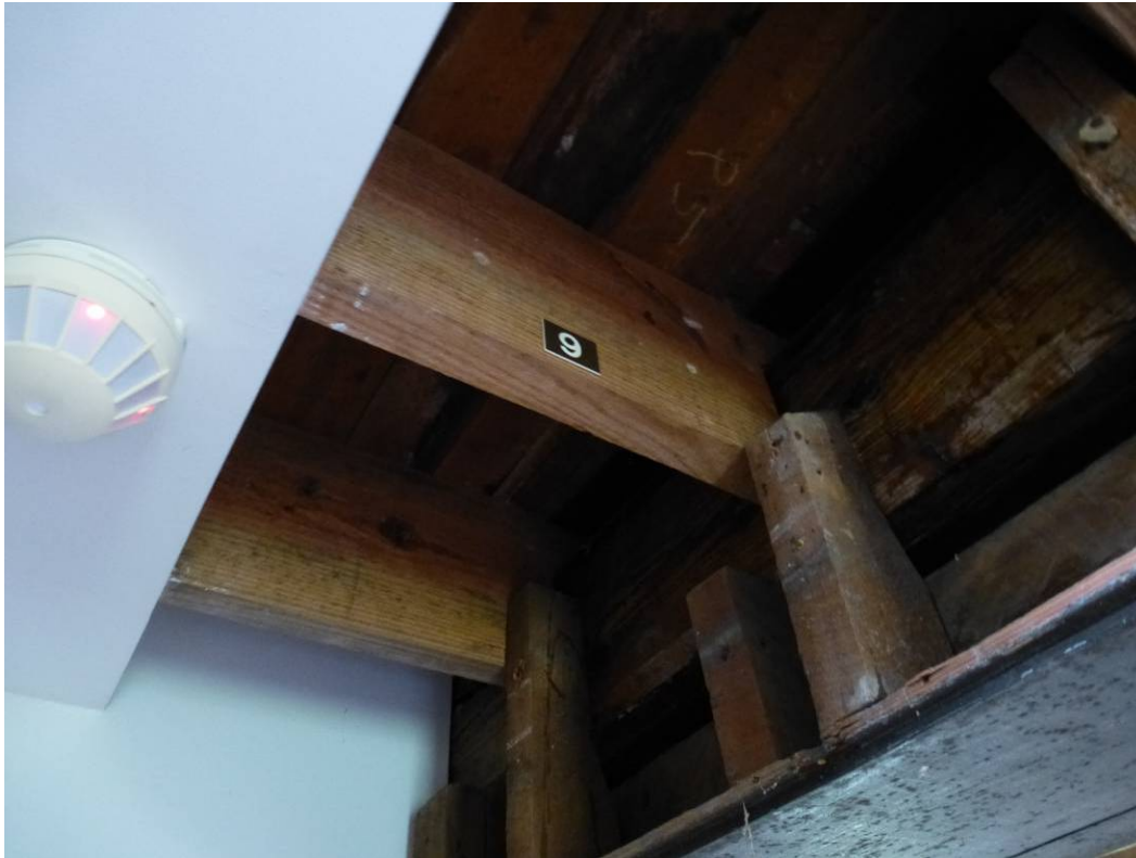
Figure 170. Most of the original ceiling joists in the main block of the house were replaced in Period III and then replaced in the preservation effort in 1993 due to decay (ERDC-CERL, 2012).
