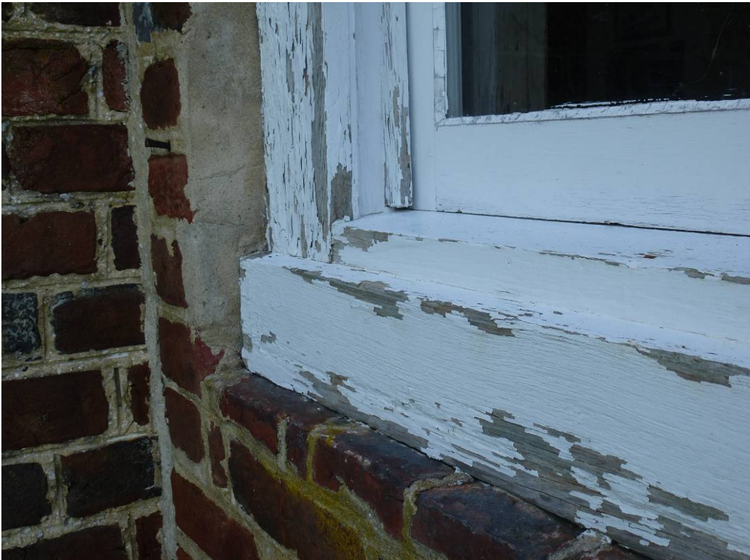
Figure 115. Deterioration of paint on wood window frame and sash (ERDC-CERL, 2012).
