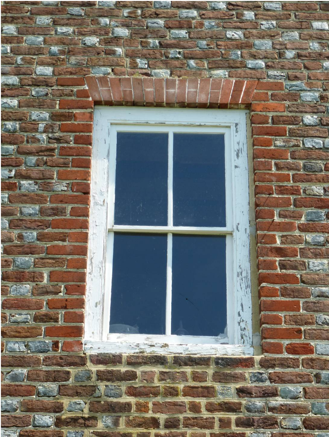
Figure 111. Second-floor Period III two-over-two wood window that should remain in place (ERDC-CERL, 2012).
