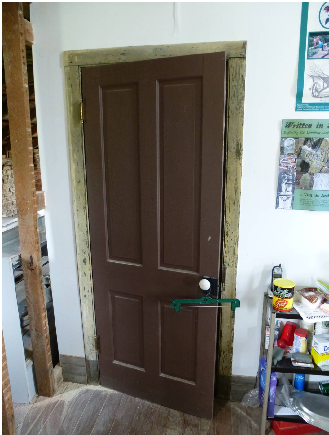
Figure 211. Typical wood panel interior door that has been painted (ERDC-CERL, 2012).
