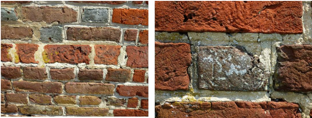
Figure 65. Incorrect mortar and excessive mortar used in previous repairs to the exterior brickwork (ERDC-CERL, 2012).
