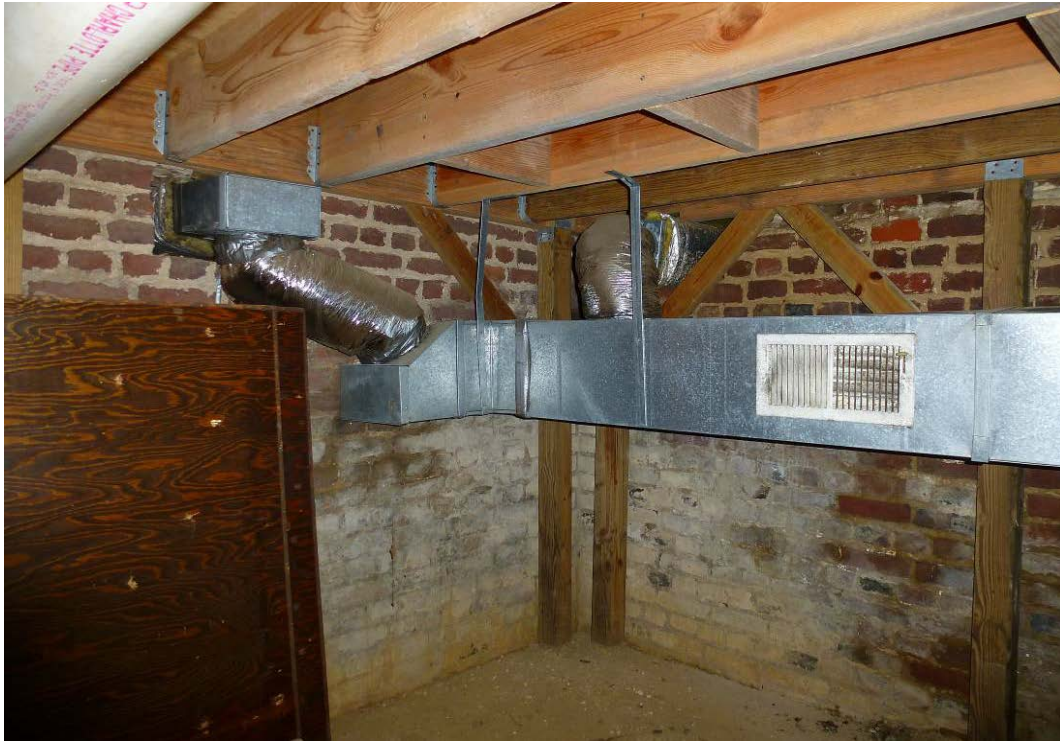
Figure 216. Either water from the ground or condensation from the HVAC system is damaging the brick cellar wall; damage is evident from the white appearance of the brick (ERDC-CERL, 2012).
