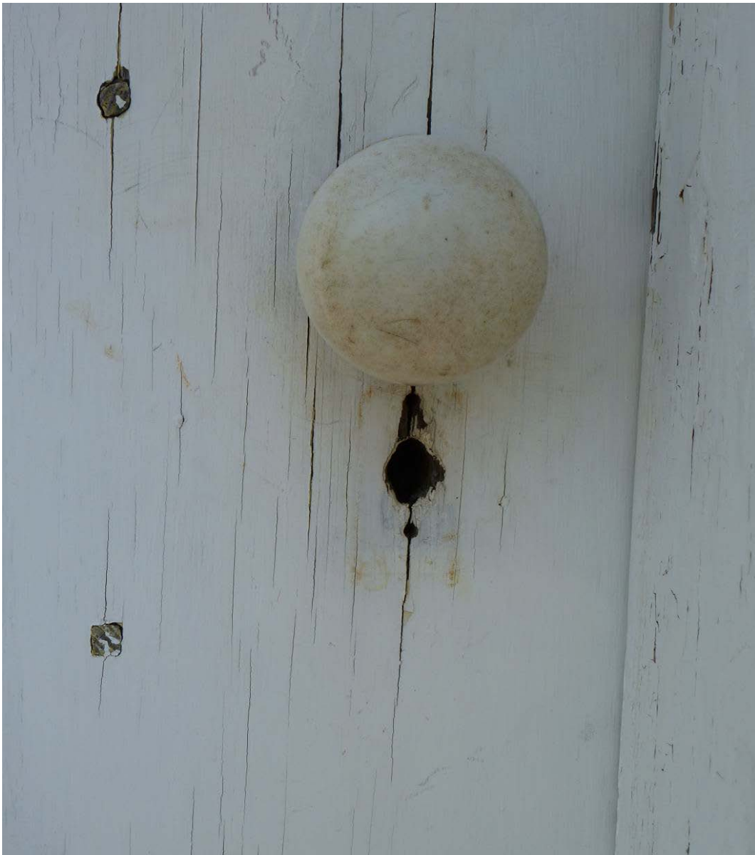
Figure 129. Door knob with missing keyhole on main front door on the southwest elevation (ERDC-CERL, 2012).
