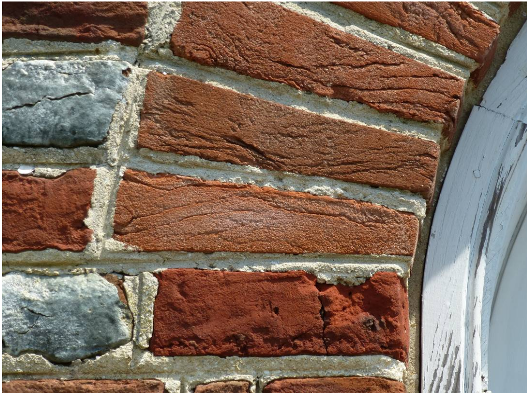
Figure 83. Close-up view of replacement bricks above arched door on the southwest elevation (ERDC-CERL, 2012).
