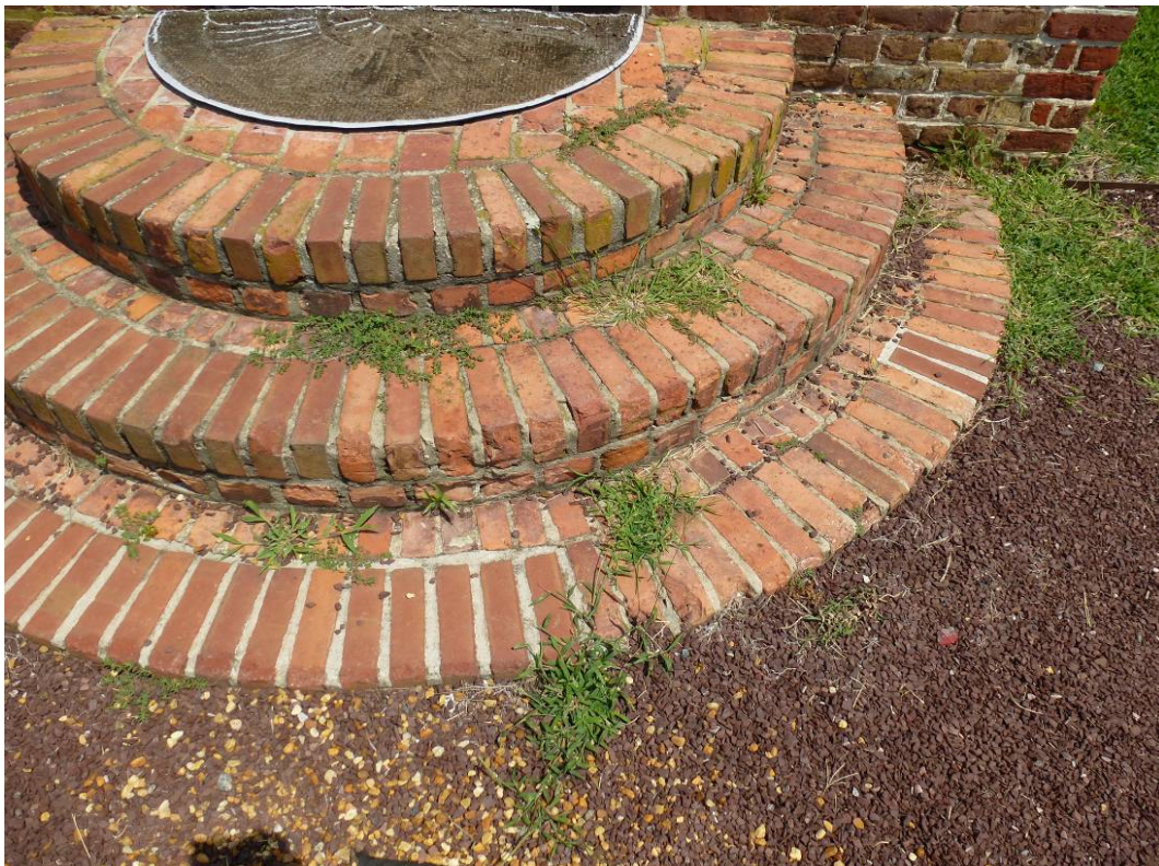
Figure 86. Semicircular design of front steps showing vegetation growth (ERDC-CERL, 2012).
