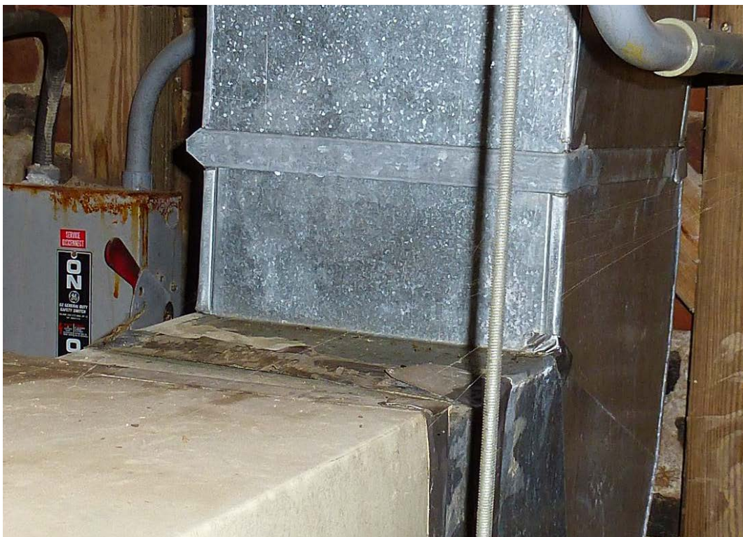
Figure 217. One of the HVAC vents is insulated, but the other is not (ERDC-CERL, 2012).
