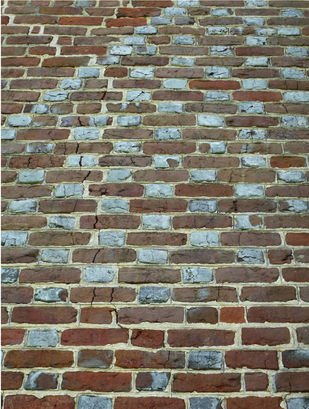
Figure 55. Long vertical crack in the northwest wall (ERDC-CERL, 2012).
