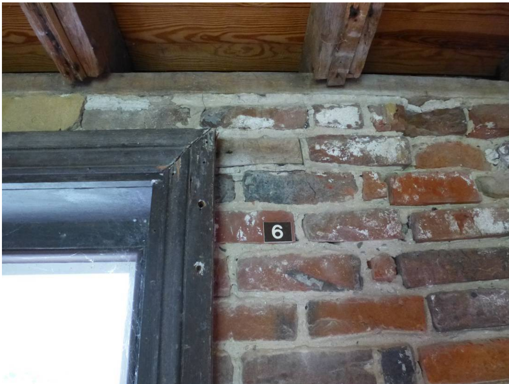
Figure 147. Brick wall in porch tower was roughly laid in Flemish bond and coarsely troweled, since the wall was intended to be plastered. (ERDC-CERL, 2012).
