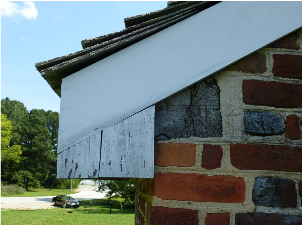
Figure 122. Split wood piece on the shed room (rear chamber) addition (ERDC-CERL, 2012).
