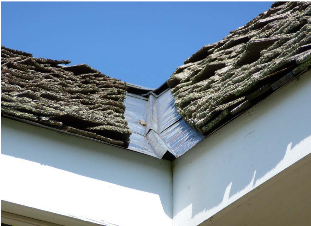
Figure 93. Flashing at the gable joint on the southeast corner of the main block and porch tower (ERDC-CERL, 2012).
