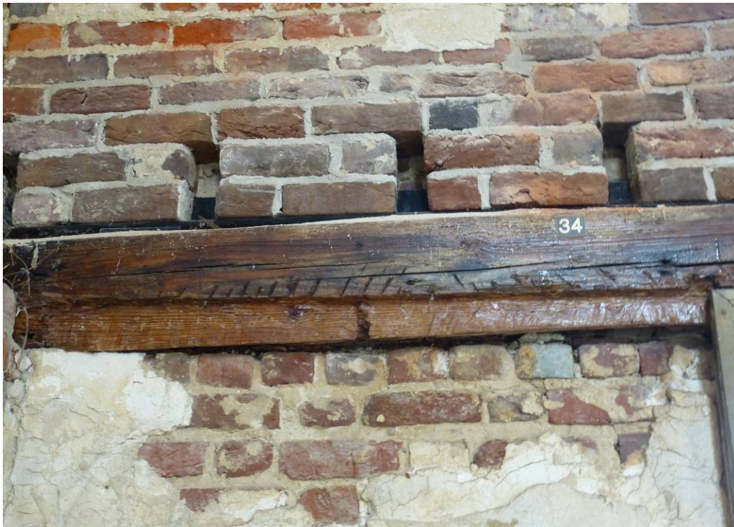
Figure 160. The rear wall plate (#34) is another surviving original timber. It was originally hand planed on the interior face, and its bottom edge was decorated with a chamfer and lamb's-tongue stops (ERDC-CERL, 2012).
