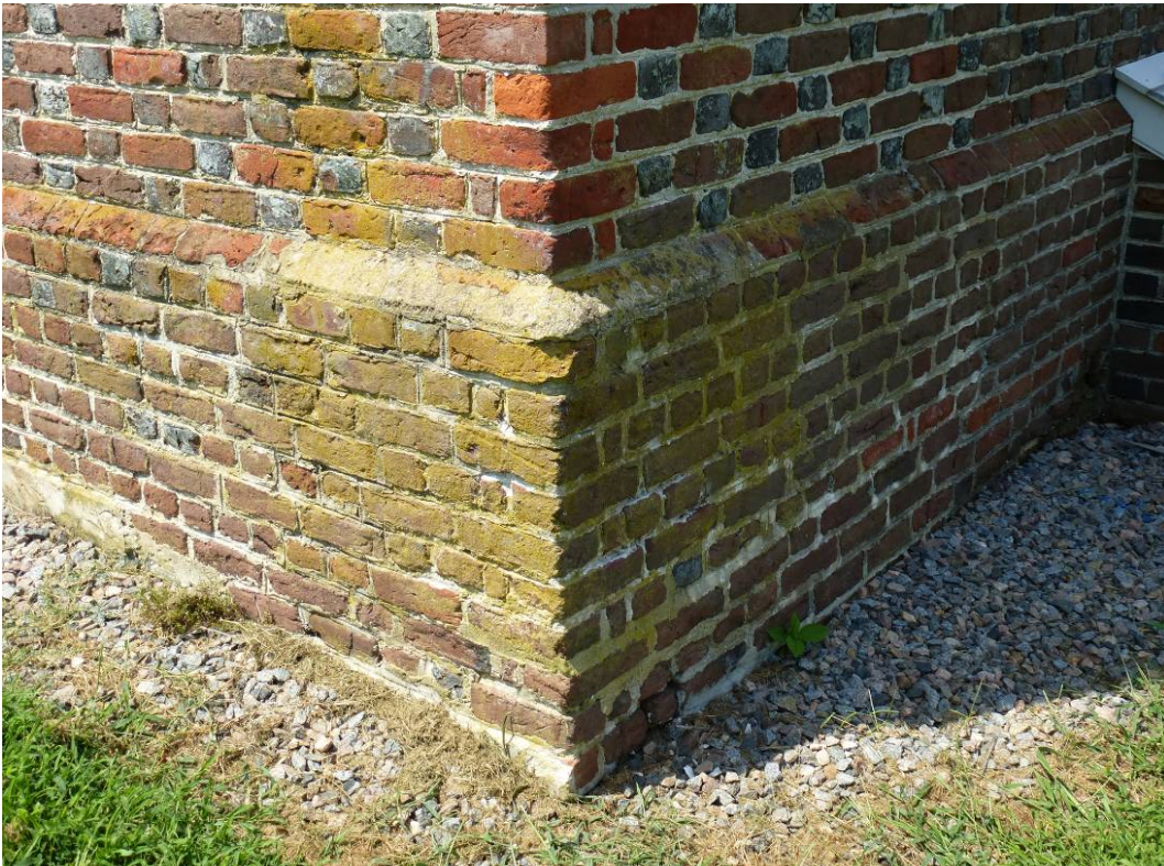
Figure 80. Stains and growth on the water table (ERDC-CERL, 2012).
