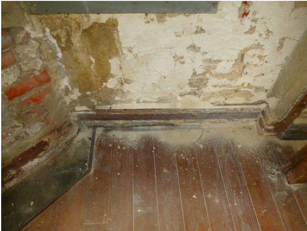
Figure 192. Failing plaster is evident with the piles of “dust” on the wood floor in the shed room (rear chamber) addition adjacent to the fireplace (ERDC-CERL, 2012).
