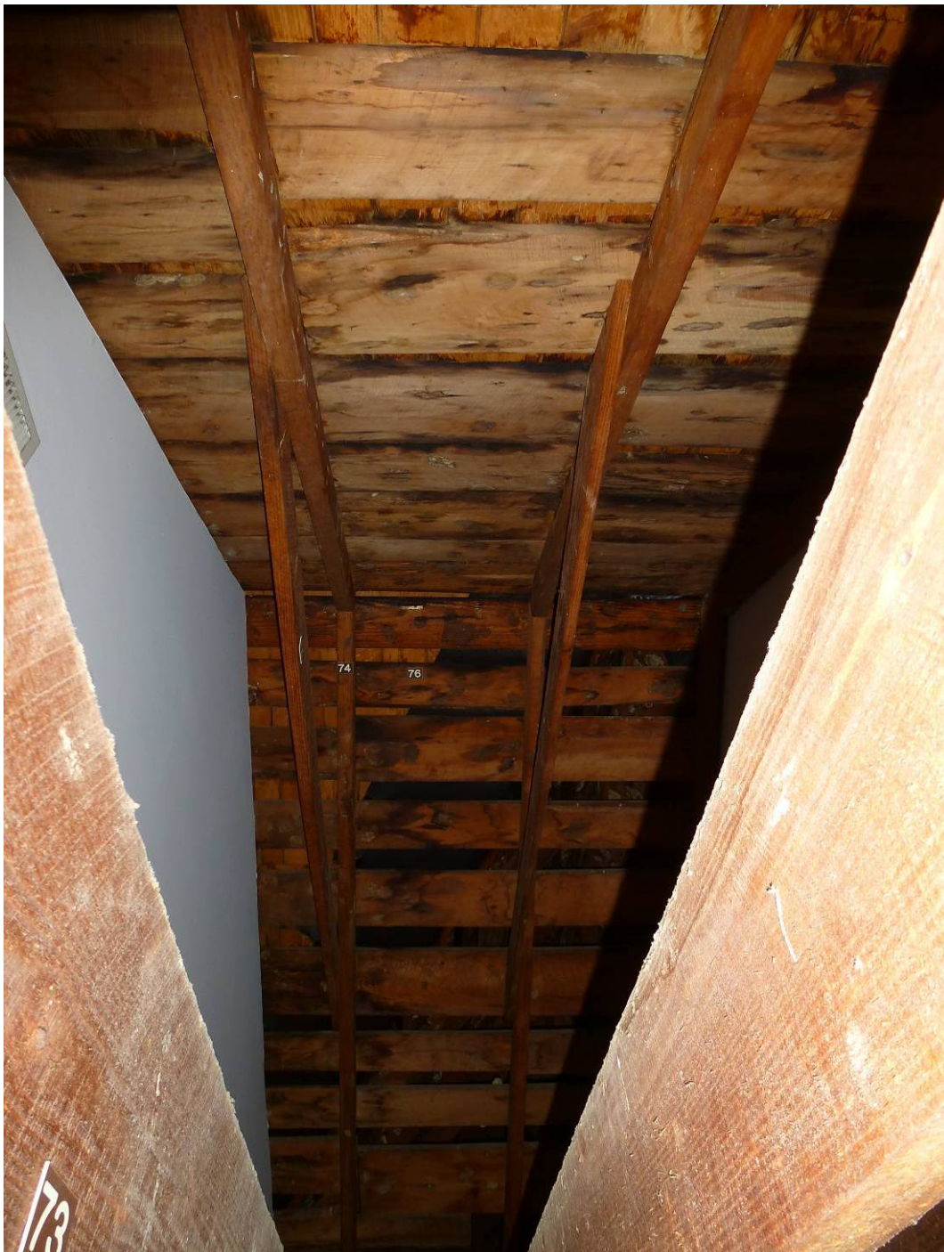
Figure 166. Looking up at the underside of the ceiling in the second-floor passage—ceiling joists, rafters, collars, and shingle lath (ERDC-CERL, 2012).
