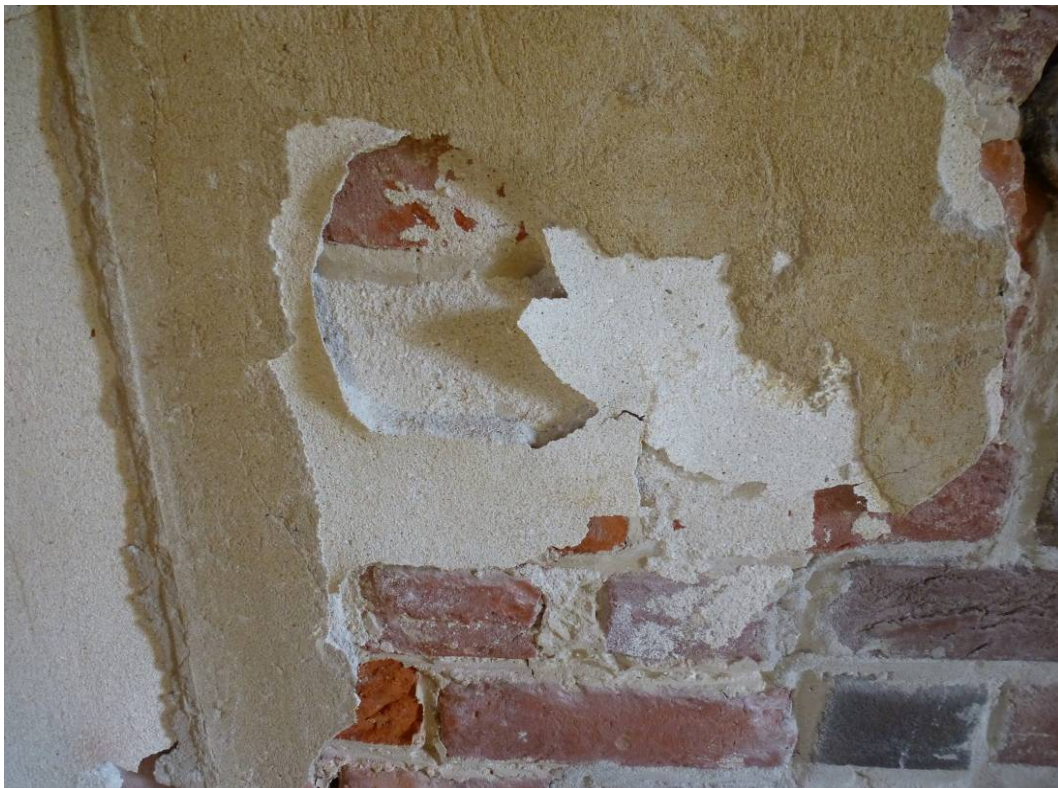
Figure 188. Failing plaster (ERDC-CERL, 2012).
