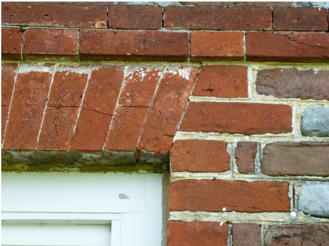
Figure 85. Close-up of rubbed brick lintel and jamb around wood window (ERDC-CERL, 2012).
