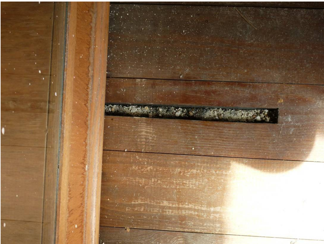
Figure 221. Debris should be cleaned out from all vents (ERDC-CERL, 2012).
