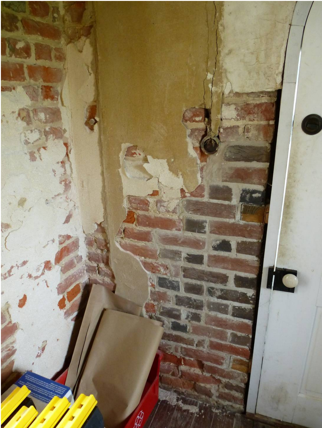
Figure 148. Northeast brick wall of porch tower with failing plaster work (ERDC-CERL, 2012).
