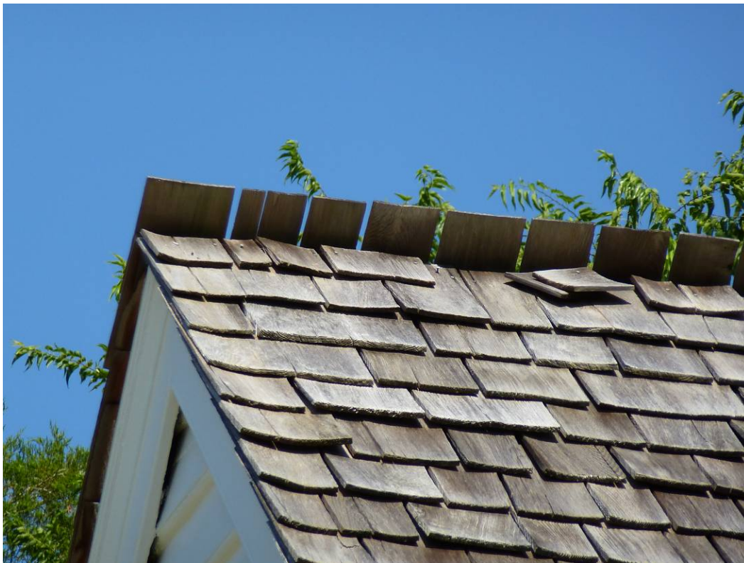
Figure 100. Example of a correctly installed cedar shingle roof at the ridge (photo taken at Yorktown, Virginia; ERDC-CERL, 2012).
