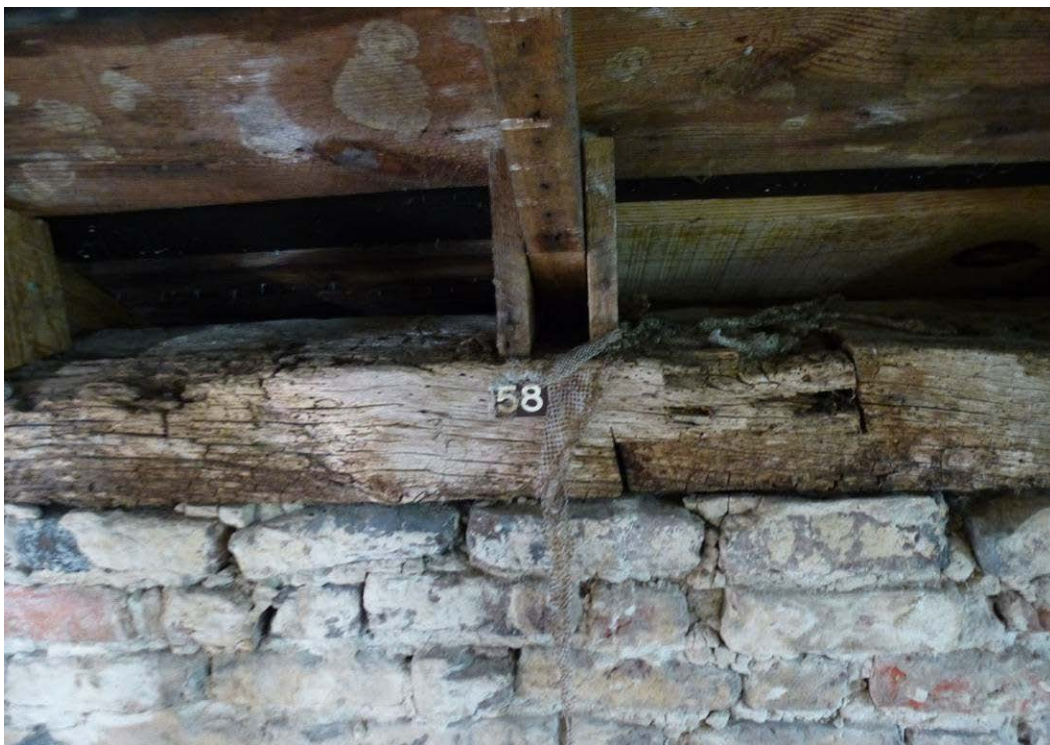
Figure 163. The rear wall plate for the shed (#58) has a “scarf” joint and is original to the construction of the shed ca. 1730. The rafters are all late nineteenth century and later replacements (ERDC-CERL, 2012).
