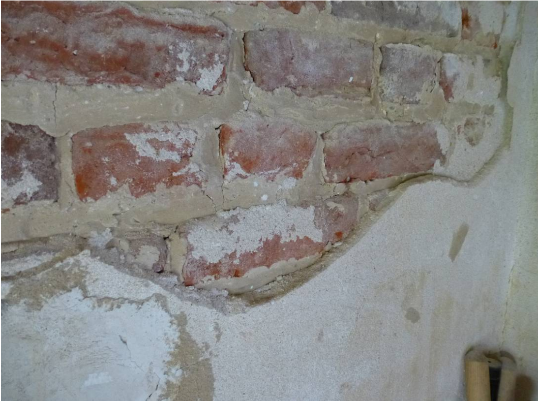
Figure 189. Plaster has fallen off the top half of the brick wall (ERDC-CERL, 2012).
