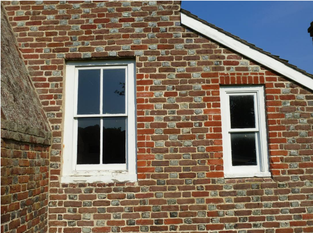
Figure 113. A two-over-two wood window on the main block and a one-over-one wood window on the southeast elevation of the shed room (rear chamber) addition that need to be replaced with an accurate Period II windows (ERDC-CERL, 2012).
