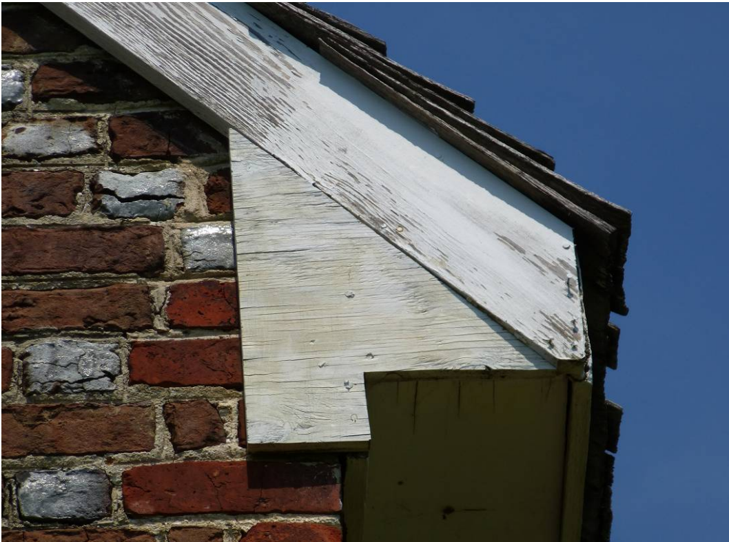
Figure 121. Close-up of weathered rakeboard (ERDC-CERL, 2012).
