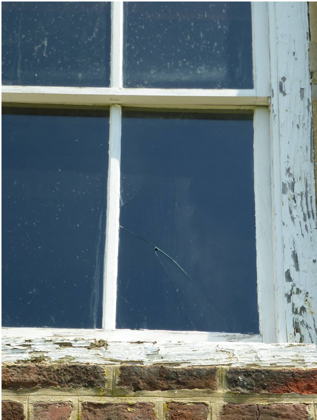
Figure 118. Cracked window pane that even has a hole in it that lets elements into the building (ERDC-CERL, 2012).
