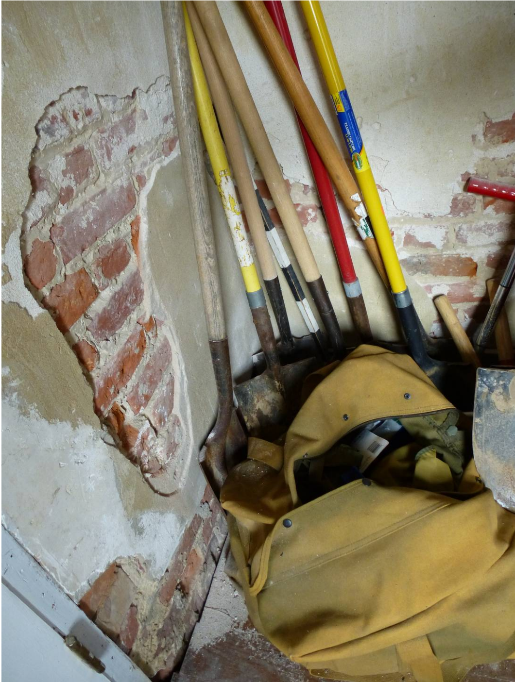
Figure 191. Equipment should be moved away from plaster walls (ERDC-CERL, 2012).
