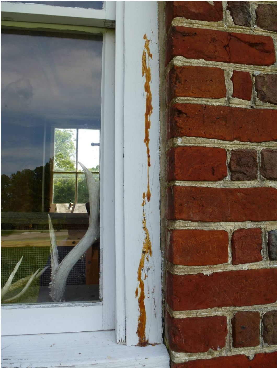
Figure 117. Stains on wood window frame need to be removed (ERDC-CERL, 2012).
