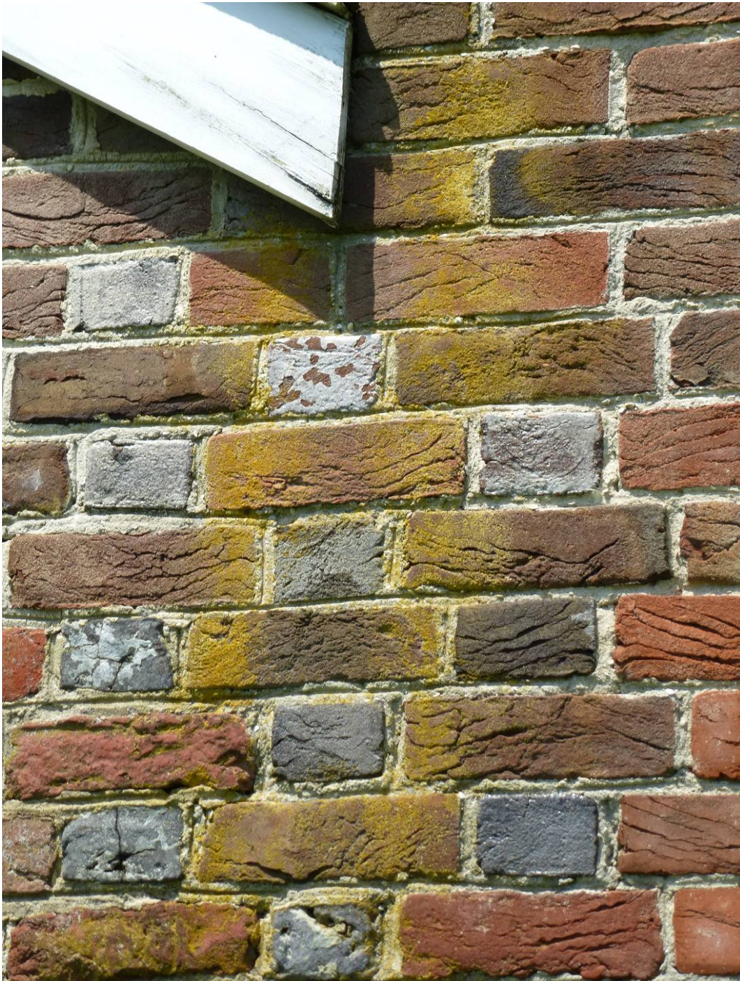
Figure 58. Growth and stains on the brickwork caused by water being shed from wood roof member (ERDC-CERL, 2012).
