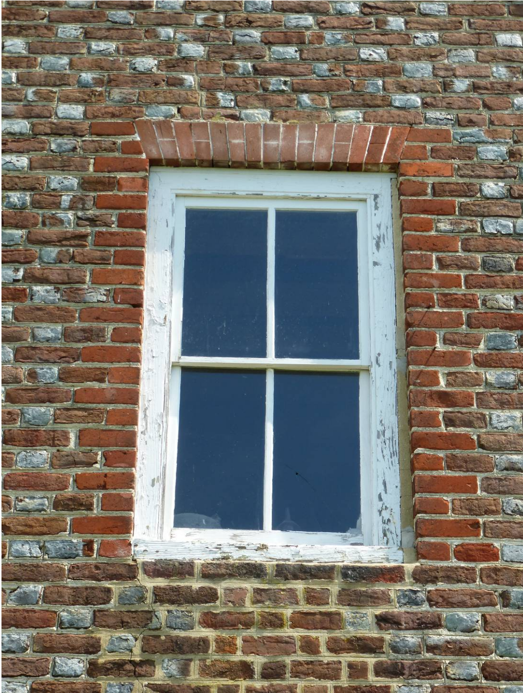
Figure 84. Rubbed brick lintel and jamb around wood window (ERDC-CERL, 2012).
