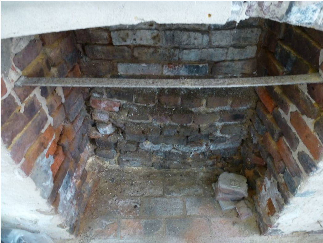
Figure 140. Brick infill when the fireplace jambs were made narrower in Period II to fireplace on the southeast wall (ERDC-CERL, 2012).
