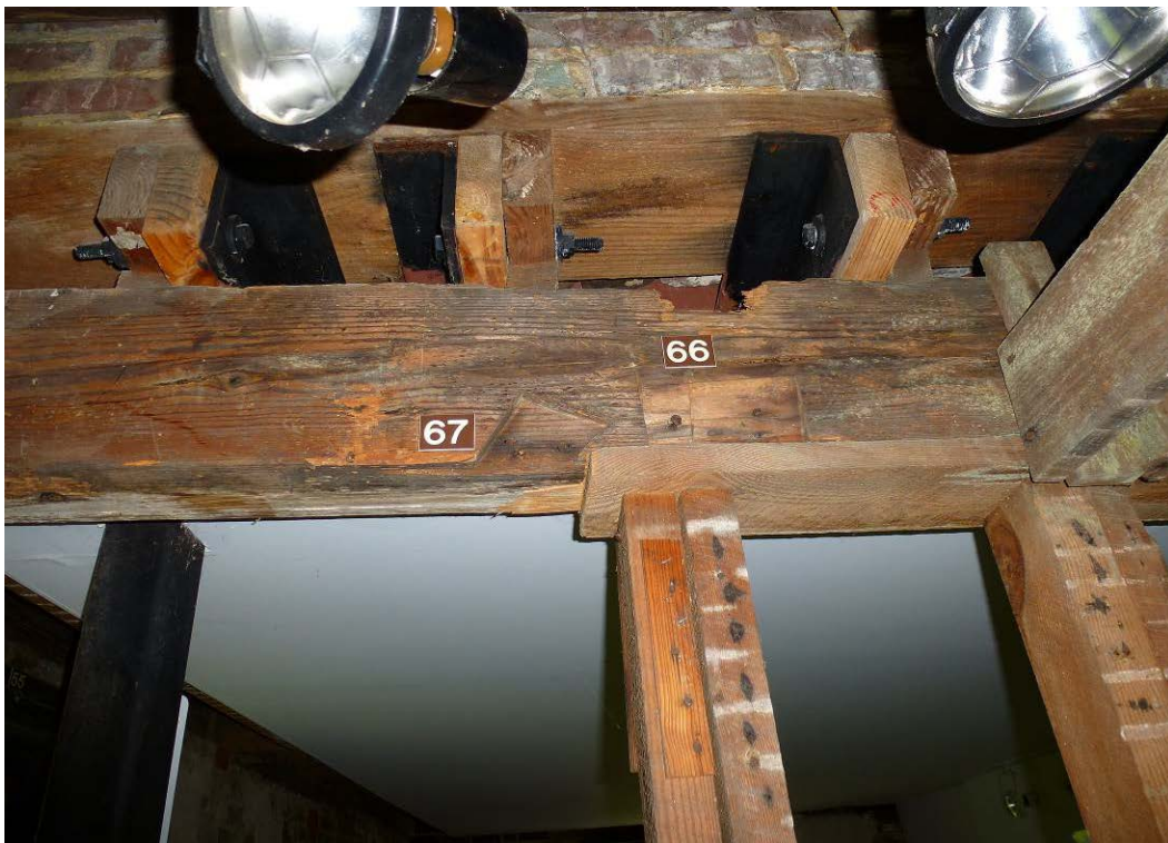
Figure 165. Rear wall plate (main block) exhibits the joints for framing from Period I and Period II (ERDC-CERL, 2012).
