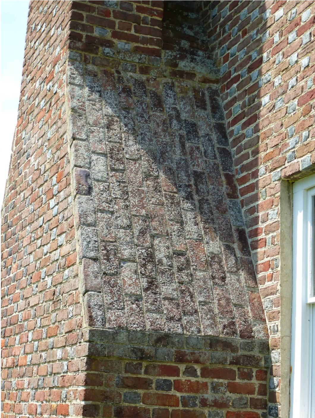
Figure 74. Efflorescence on the chimney brickwork (ERDC-CERL, 2012).
