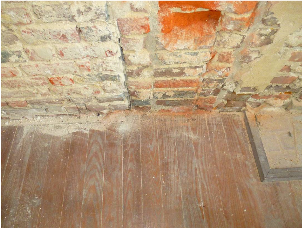
Figure 88. Interior of brick wall showing the “brick dust” (ERDC-CERL, 2012).
