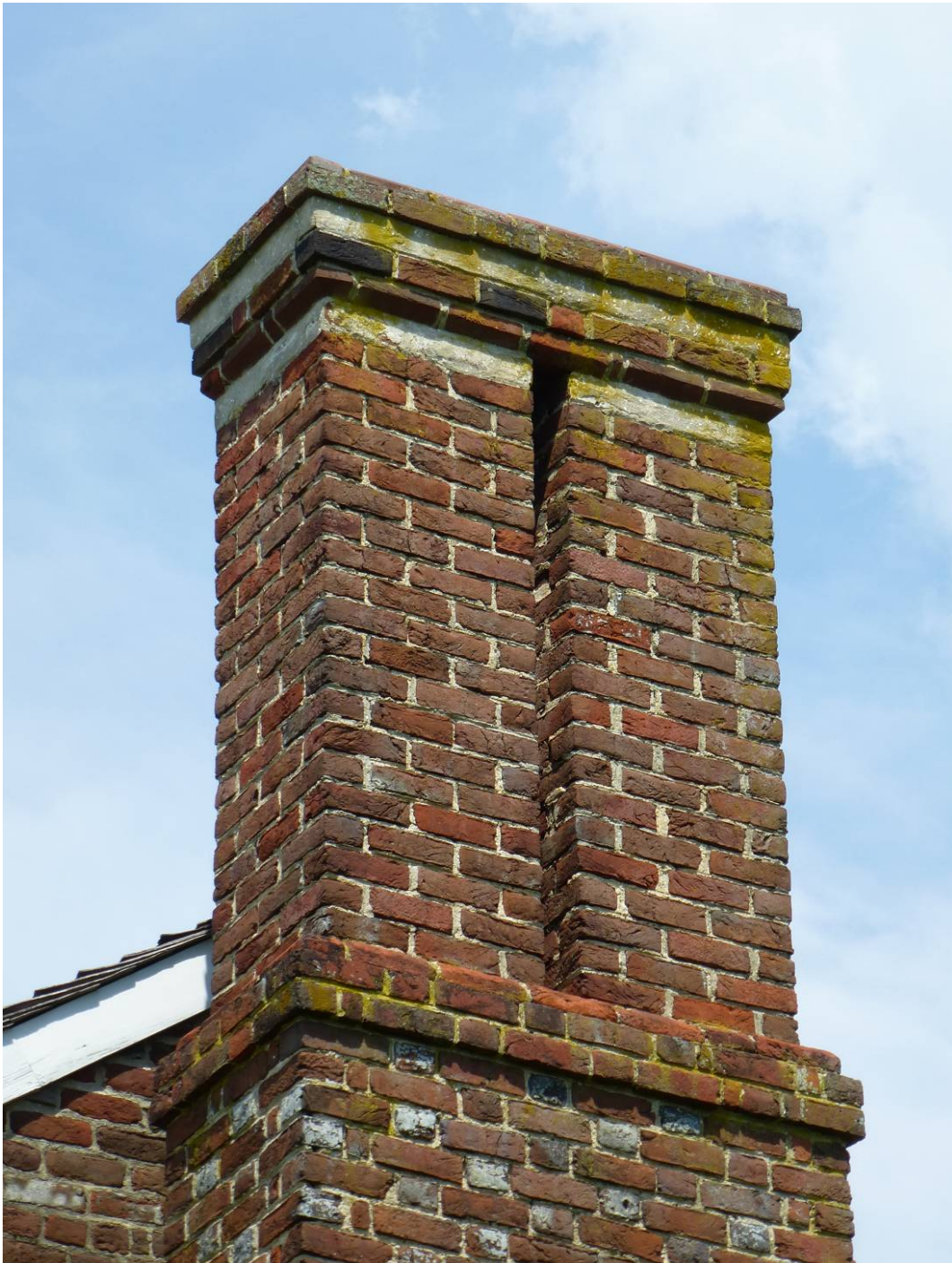
Figure 71. The top three courses of the original cap survive under the late nineteenth-century stack extensions (ERDC-CERL, 2012).
