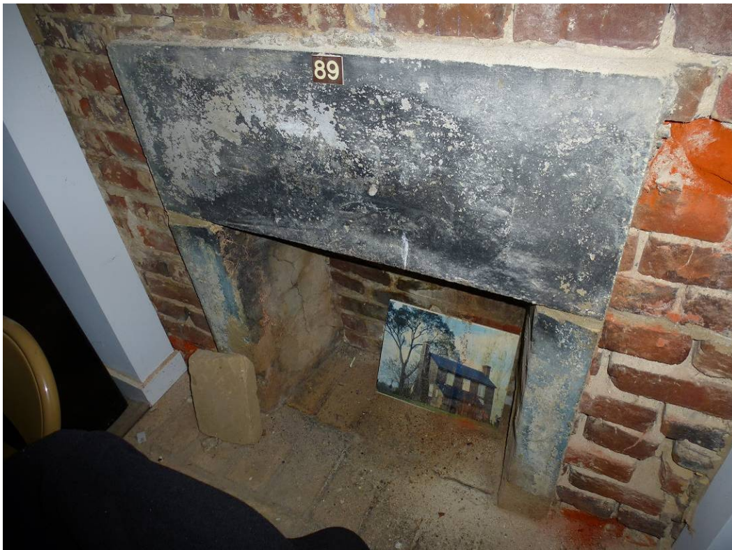
Figure 143. Fireplace on the second floor on the southeast wall. The fireplace was cut into the original chimney in Period II. The concrete was added in 1893 (Period III) (ERDC-CERL, 2012).
