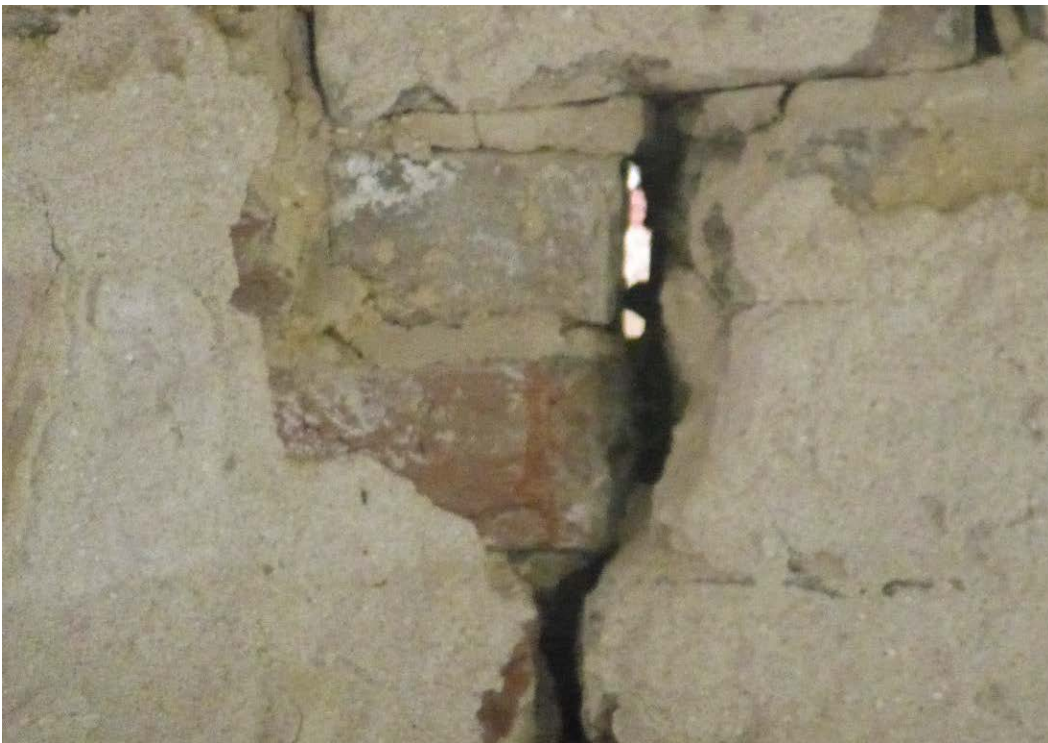
Figure 152. Close-up of the structural crack above the fireplace on the northwest wall (ERDC-CERL, 2012).
