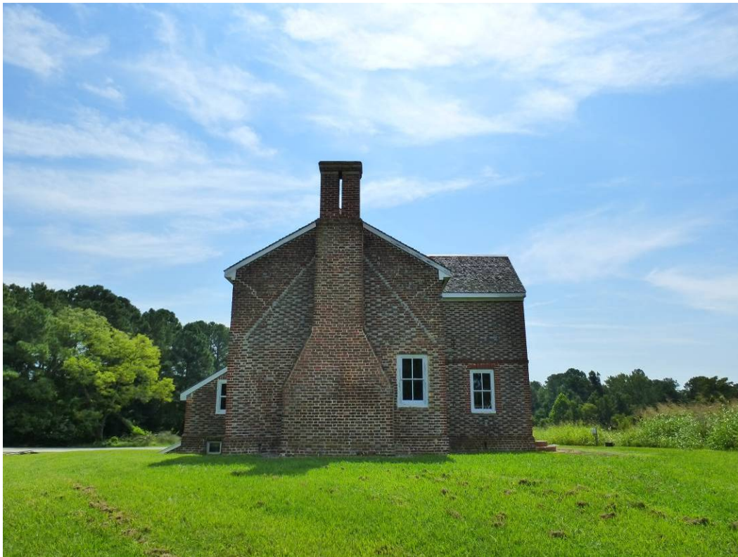
Figure 9. Northwest elevation of Matthew Jones House showing original chimney, ca. 1730 brick walls, porch tower (right), and rear shed (left) (ERDC-CERL, 2012).
