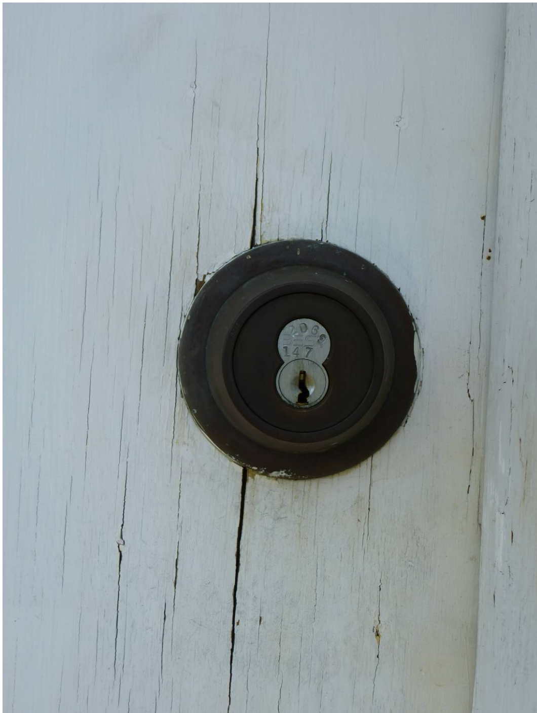
Figure 130. Newer lock added to the front door on the southwest elevation; notice the cracking wood from insertion of the hardware (ERDC-CERL, 2012).
