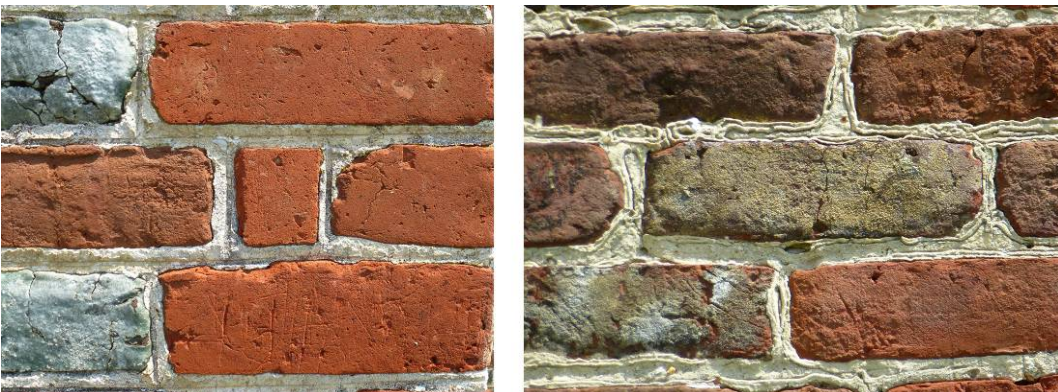
Figure 67. Comparison photographs: Correct technique for grapevine mortar joint on the left compared to incorrect technique on the right (ERDC-CERL, 2012).
