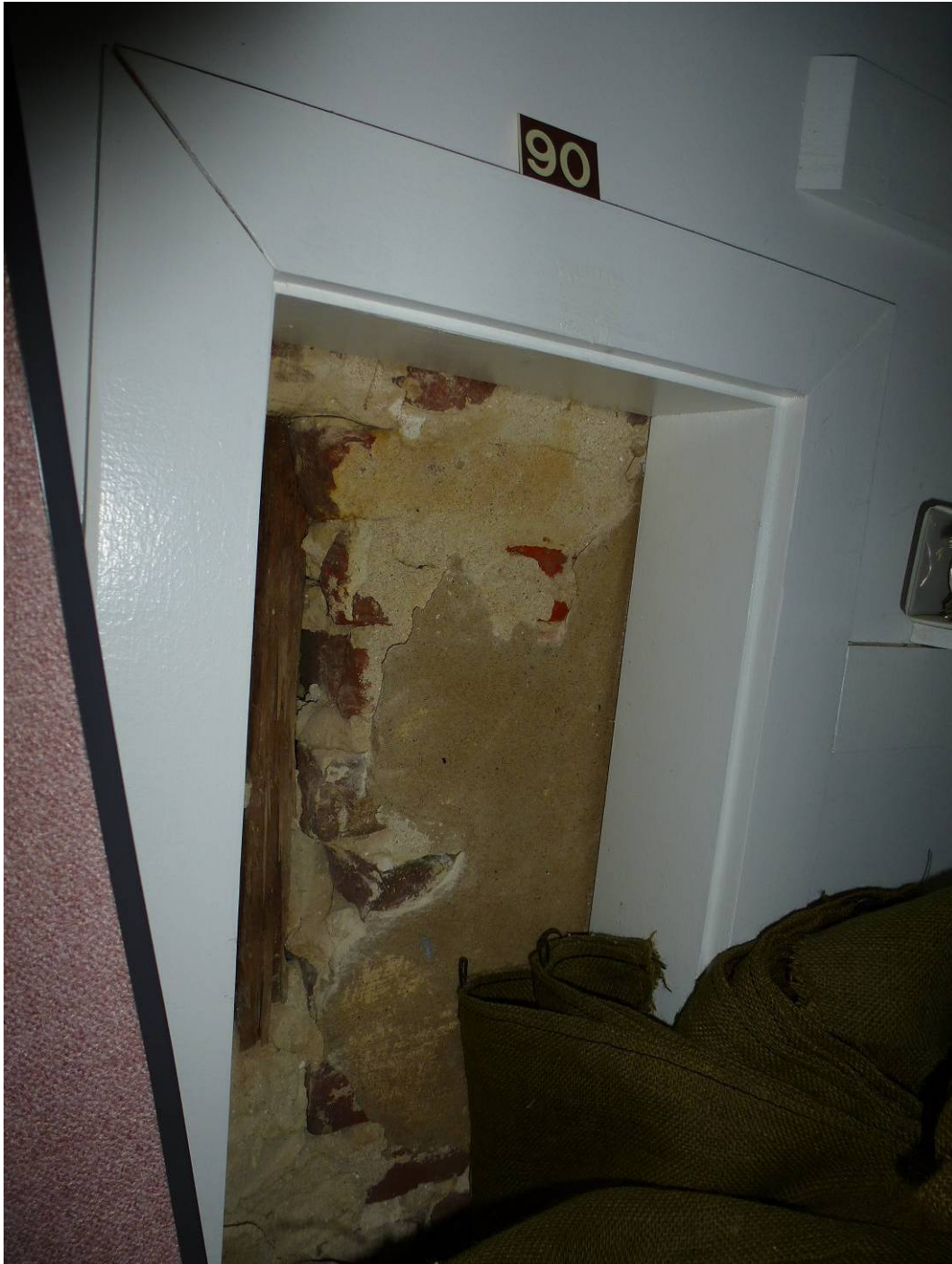
Figure 169. The knee-wall stud is a Period I feature, left in place during both the ca. 1730 and 1893 renovations. The brick work to the right of the stud was added when the building was raised fully to two stories in Period II. (ERDC-CERL, 2012).
