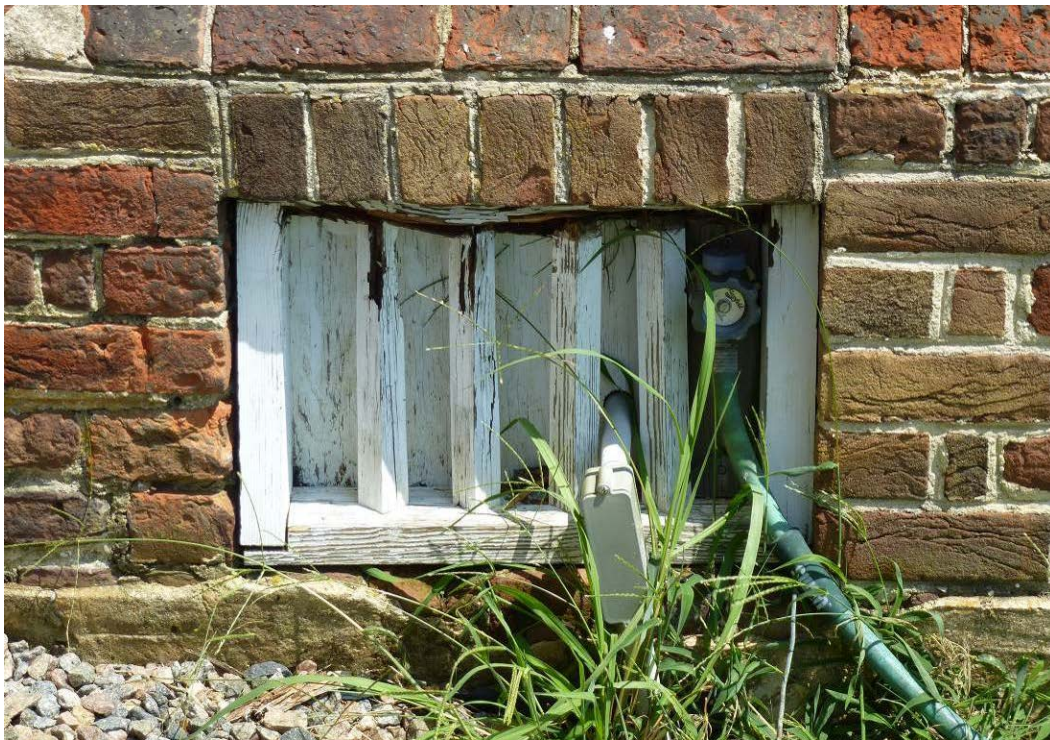
Figure 127. Wood-louvered cellar vent with garden house connection on the southwest elevation (ERDC-CERL, 2012).
