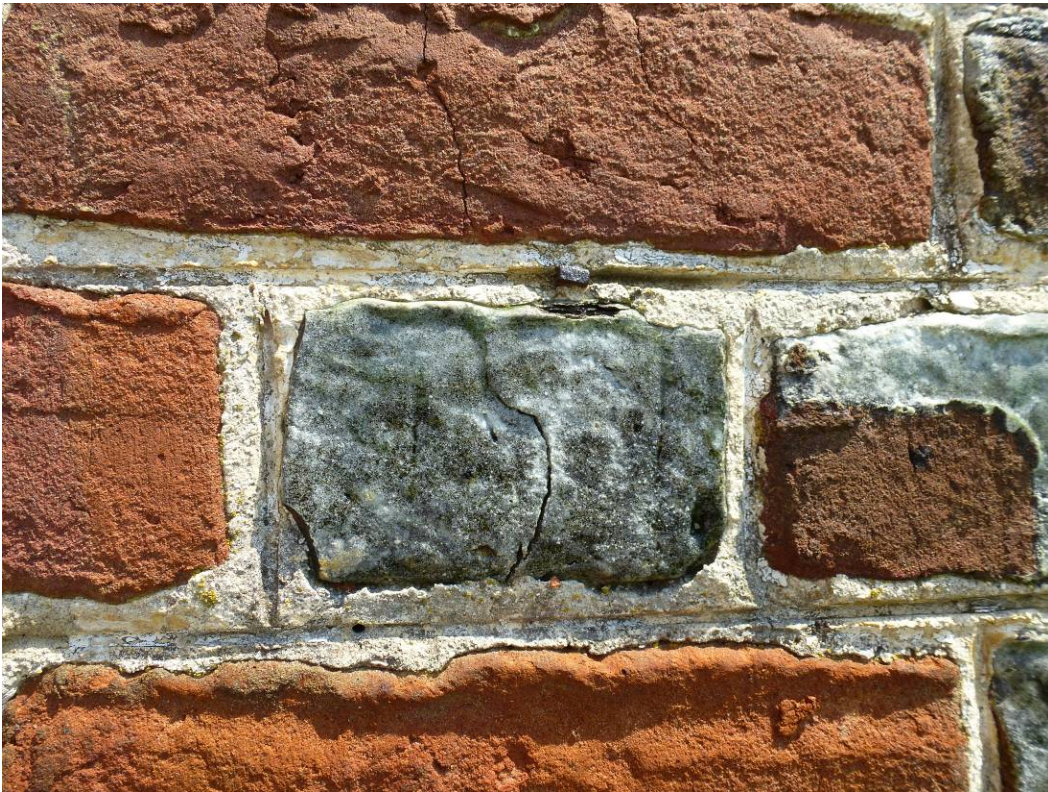
Figure 59. Flaking of the glaze on the brick (center right) is visible on several glazed bricks on the exterior wall (ERDC-CERL, 2012).
