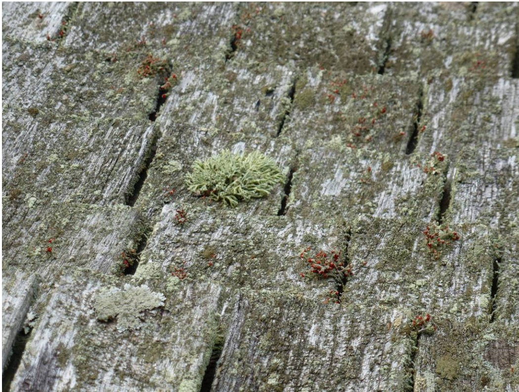
Figure 91. Mold and lichen growth on wood shingles (ERDC-CERL, 2012).
