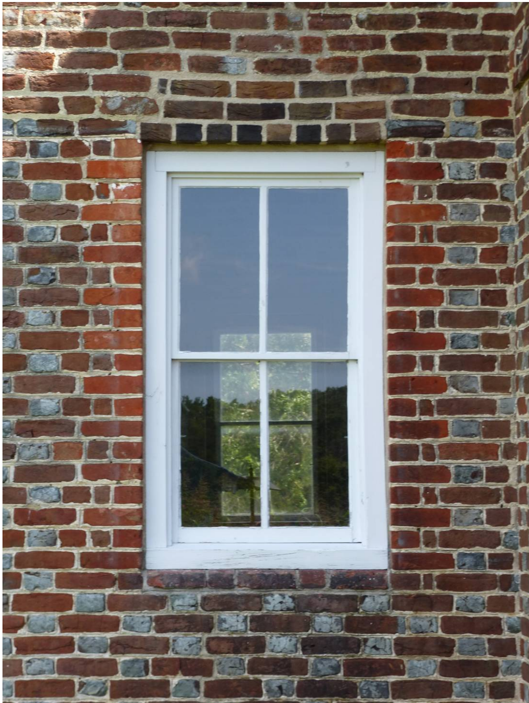
Figure 33. Wood windows on the first floor of the Matthew Jones House need to be replaced with more appropriate Period II windows (ERDC-CERL, 2012).
