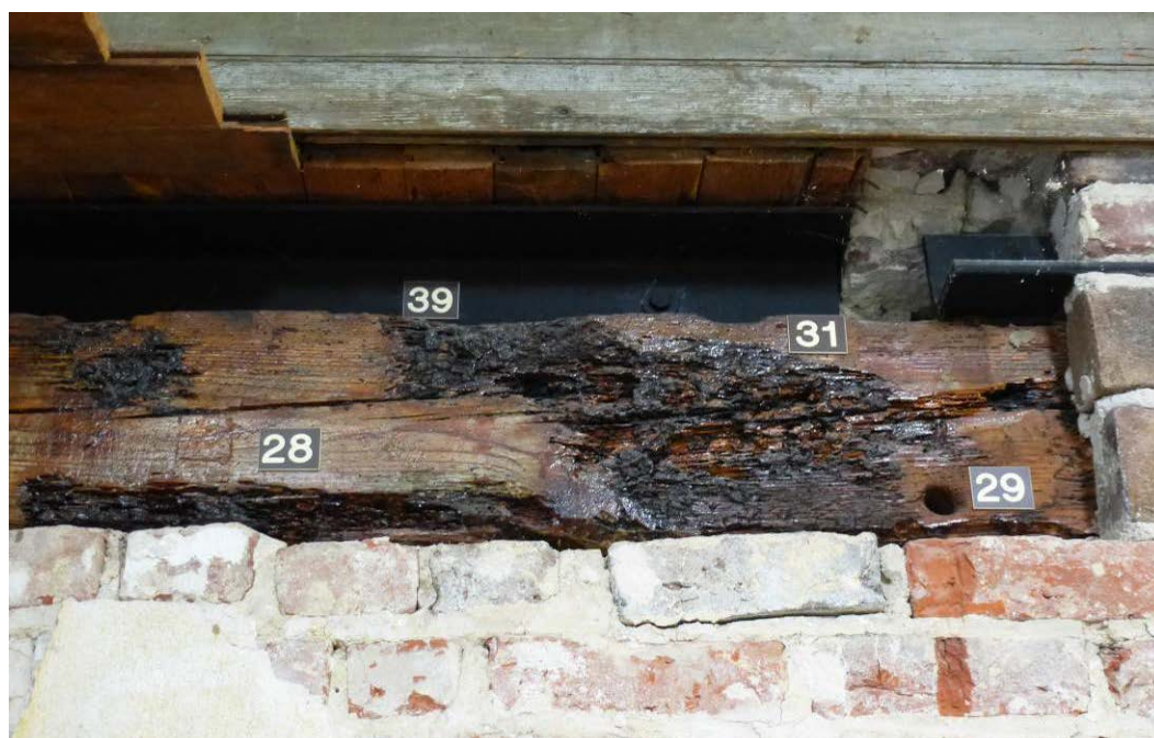
Figure 157. Architectural study feature #28-points out the front wall plate on the southwest wall that is one of the four main timbers to survive from Period I. Feature #29 highlights the peg hole representing the location of one of the four main posts along the front wall. The peg secured the tenon of a post that was exposed in the room. Feature #31 highlights ghost joists. The original joists were removed in 1893. Feature #39 highlights steel supports added during the 1993 preservation efforts (ERDC-CERL, 2012).
