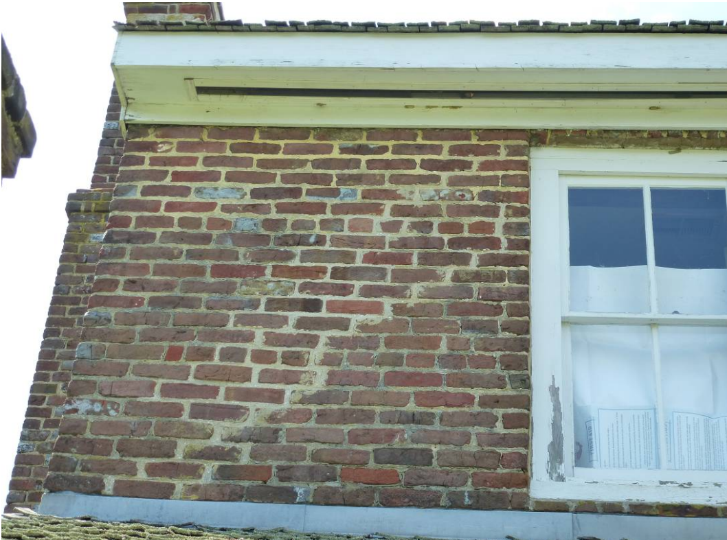
Figure 62. Replacement mortar used on the second floor on the northeast elevation (ERDC-CERL, 2012).
