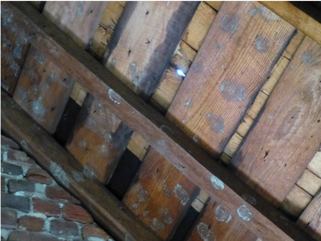
Figure 98. Gaps in the wood shingles where you can see light through, and allowing exterior elements to penetrate into the interior of the house (ERDC-CERL, 2012).
