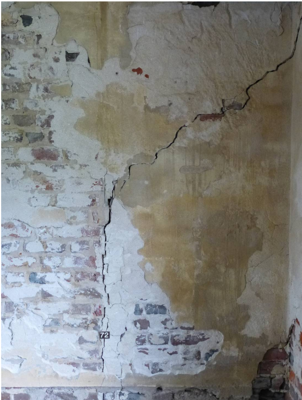
Figure 153. The knee-wall studs on the northwest wall caused vertical cracks not only in the plaster but also in the brick wall (ERDC-CERL, 2012).
