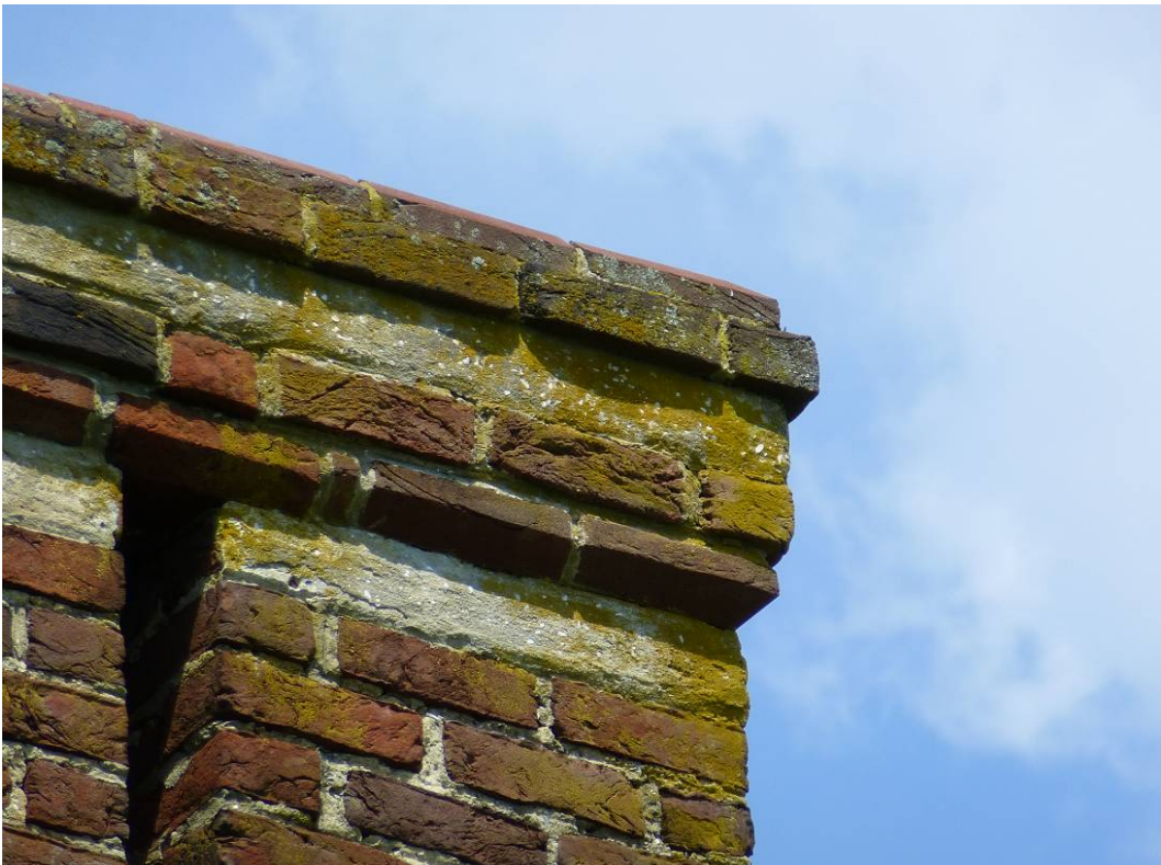
Figure 73. Growth/stains on the top of the chimney brickwork (ERDC-CERL, 2012).
