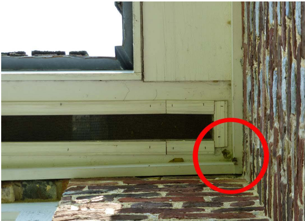
Figure 125. Several areas under the wood soffit where insect nests have formed. Here, one area is circled in red. All should be removed (ERDC-CERL, 2012).
