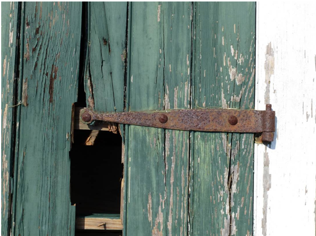
Figure 131. Door hinge on wood cellar door. Whenever the doors are replaced, the hardware should either be repaired or replaced in-kind (ERDC-CERL, 2012).
