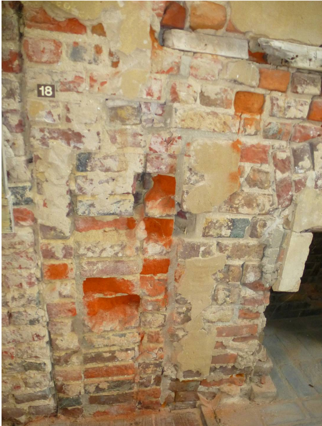
Figure 134. Joint with brick wall showing the brick infill used to make the original large hall fireplace smaller. Also note the deterioration of the brick in the west fireplace (ERDC-CERL, 2012).
