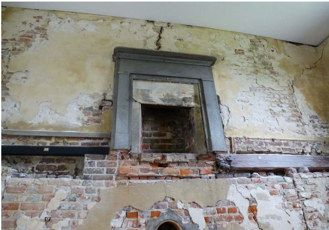
Figure 139. This fireplace (on the second-floor chambers northwest wall) was cut into the chimney ca. 1730 (ERDC-CERL, 2012).
