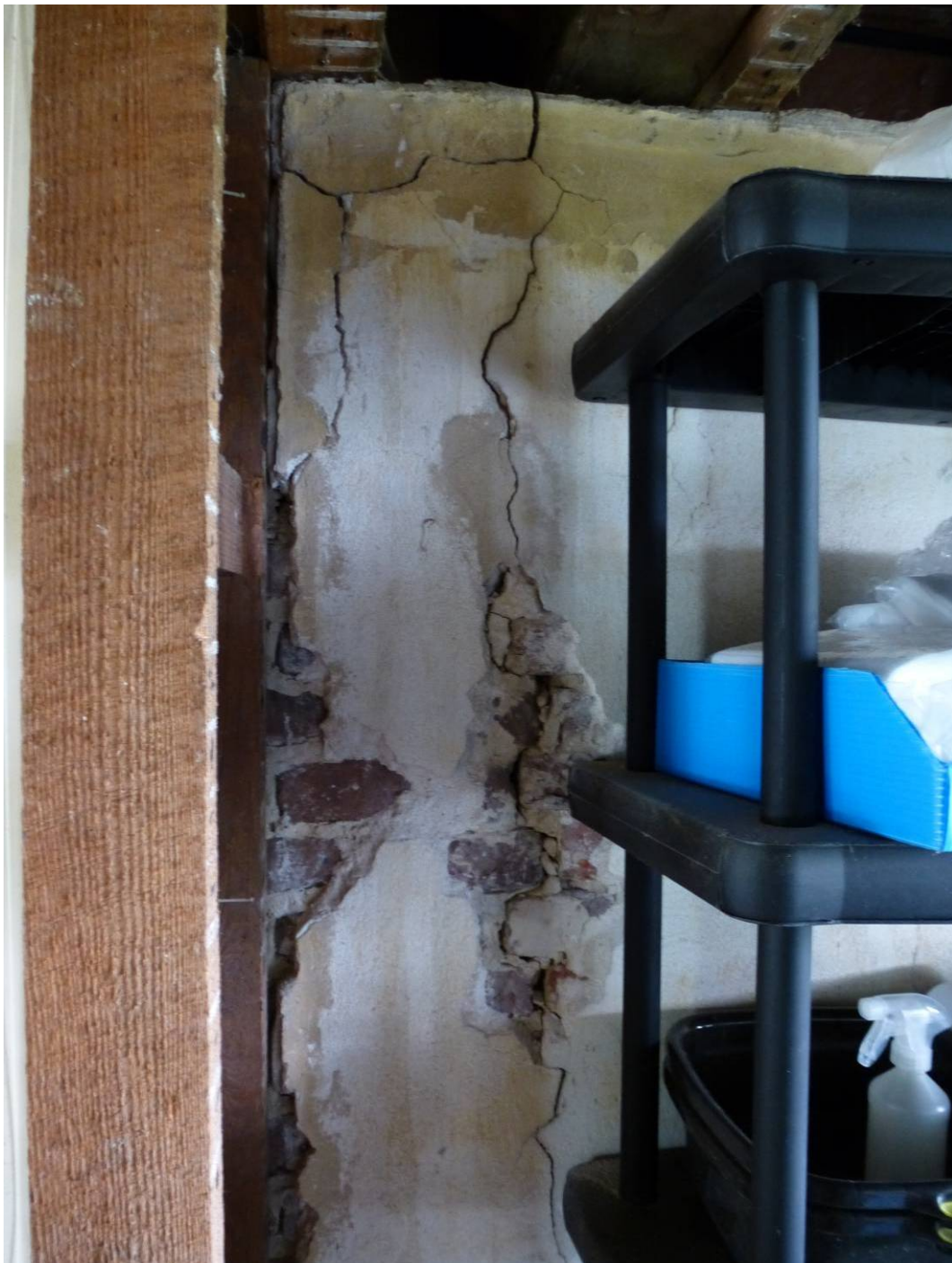
Figure 154. Second-floor southeast wall of porch tower is showing signs of cracking in both plaster lath and brick exterior wall (ERDC-CERL, 2012).
