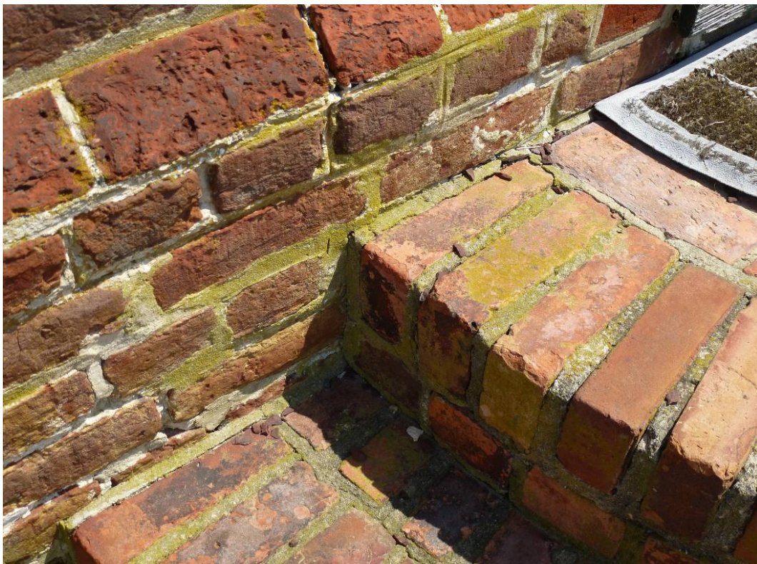
Figure 87. Growth and stains on front steps from rain water (ERDC-CERL, 2012).
