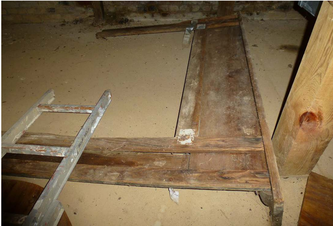
Figure 172. One of the original 1893 wood mantel (from first-floor hall) is being improperly stored when propped against a damp brick wall in the cellar (ERDC-CERL, 2012).
