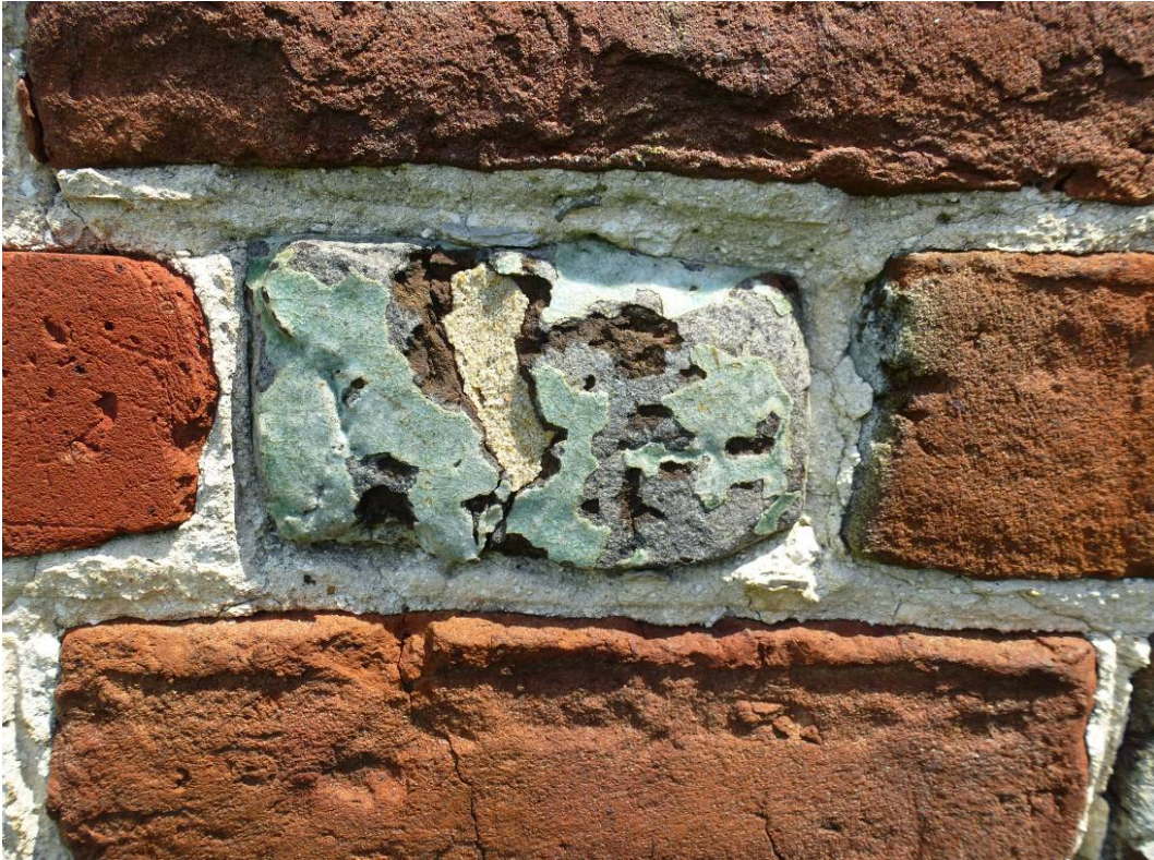
Figure 61. Improper repair of glazed header brick (ERDC-CERL, 2012).
