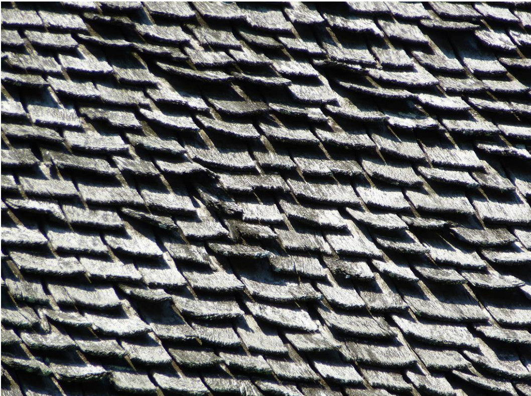
Figure 90. Weathered wood shingles, uniformly across entire roof (ERDC-CERL, 2012).
