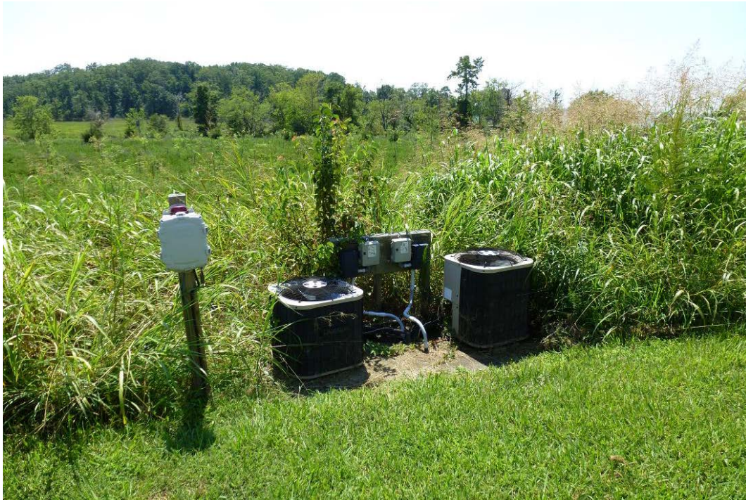
Figure 214. Exterior AC units located on the south side of the property; the vegetation should be cut back and removed where immediately adjacent to the units (ERDC-CERL, 2012).
