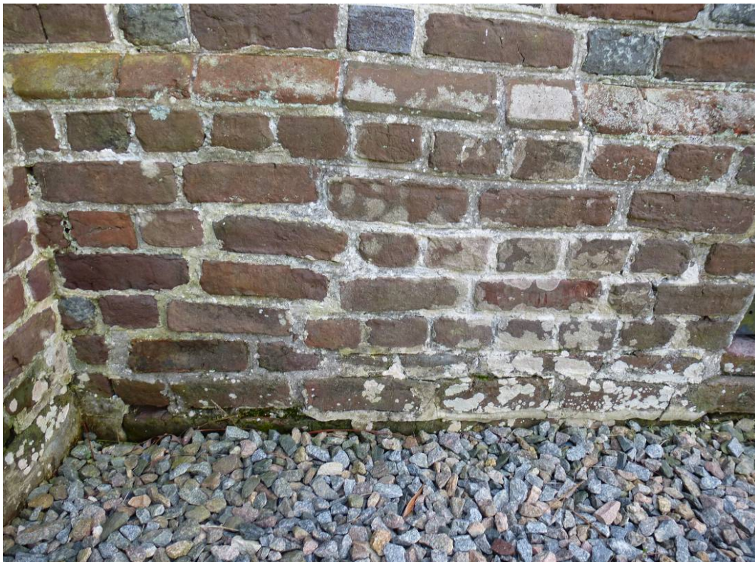
Figure 78. Lichen growth and efflorescence on the water table caused by rain water shedding from roof and splashing back onto the brickwork (ERDC-CERL, 2012).
