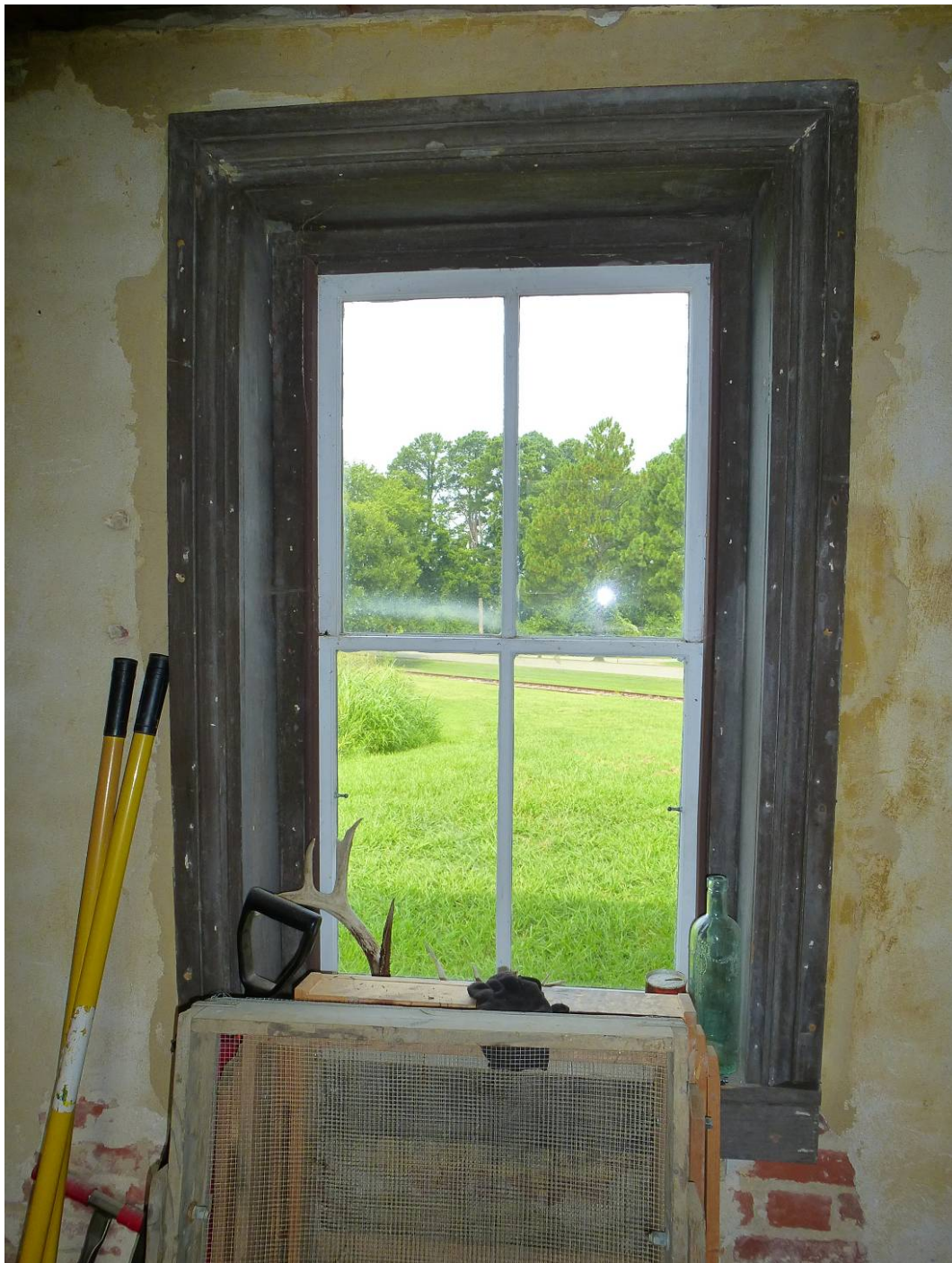
Figure 204. All jambs throughout the house were replaced in the late nineteenth century (ERDC-CERL, 2012).
