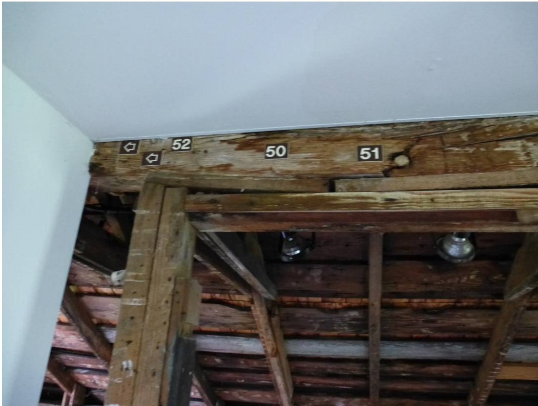
Figure 162. Rear wall plate in dining room indicated by #50 (ERDC-CERL, 2012).
