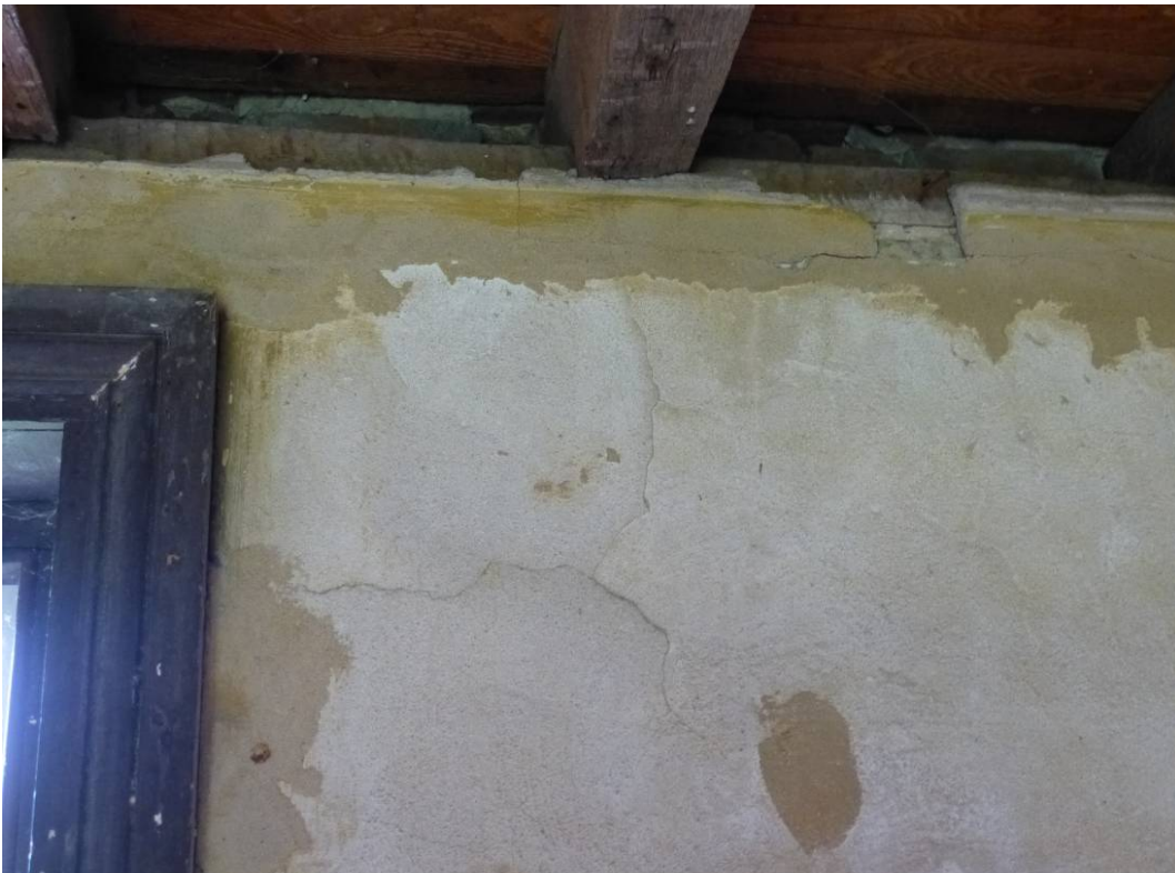
Figure 190. Here there are cracks in plaster wall (ERDC-CERL, 2012).
