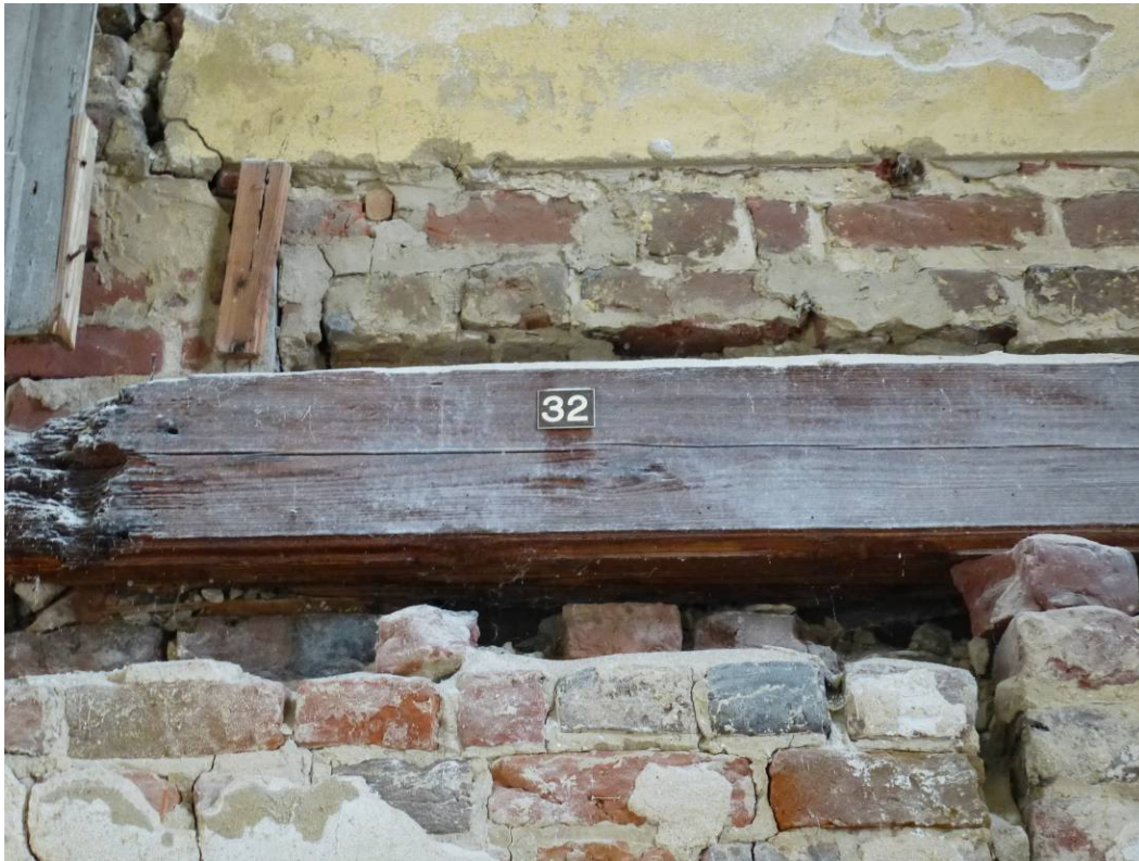
Figure 158. End joist in hall (ERDC-CERL, 2012).
