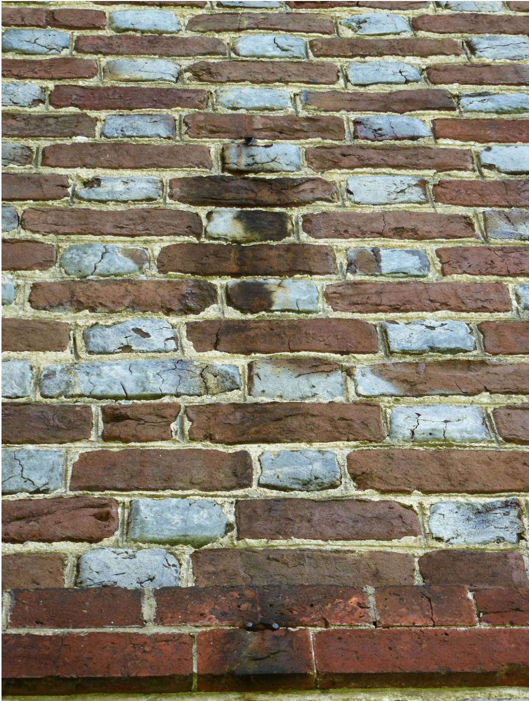
Figure 57. Stains on the brickwork caused by protruding nails should be cleaned according to the Secretary of Interior Standards for Rehabilitation (ERDC-CERL, 2012).
