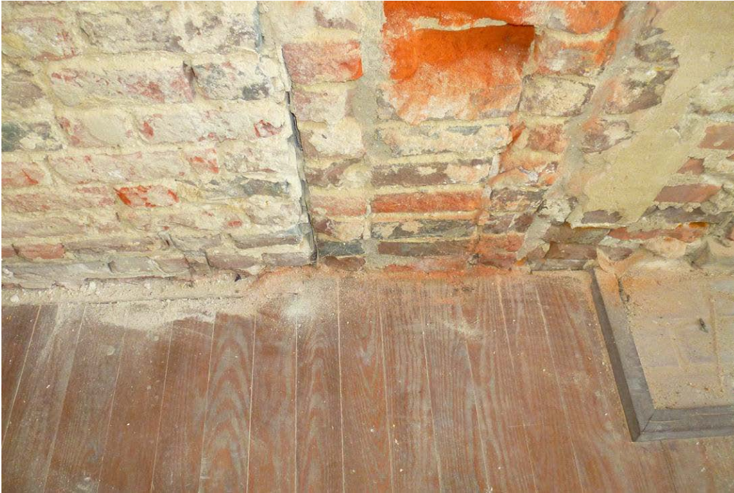
Figure 149. Brick “dust” from deteriorating bricks (ERDC-CERL, 2012).
