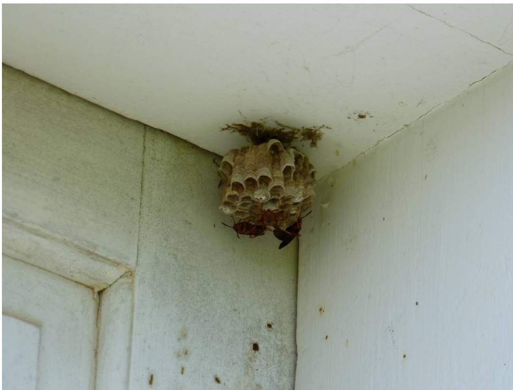
Figure 107. The insect growth/nests should be removed from all wood members (ERDC-CERL, 2012).
