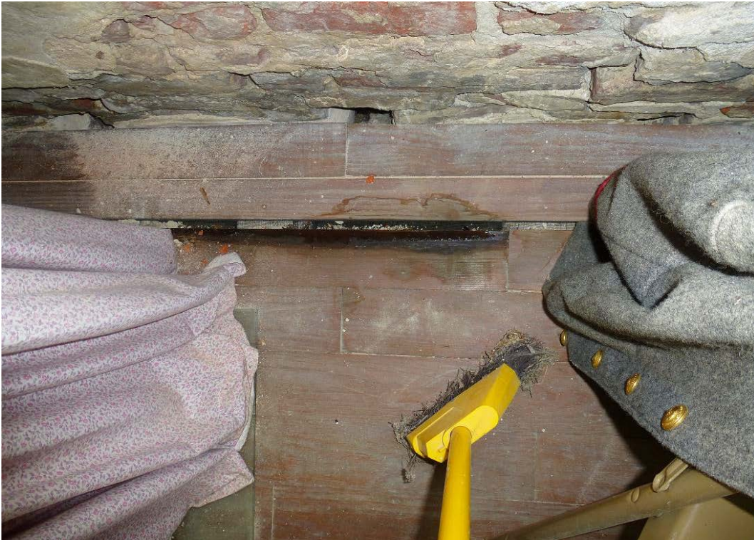
Figure 200. A newer HVAC vent has been cut in narrow slits in various places in the wood floor. The moisture from the HVAC system is damaging the floorboards (ERDC-CERL, 2012).
