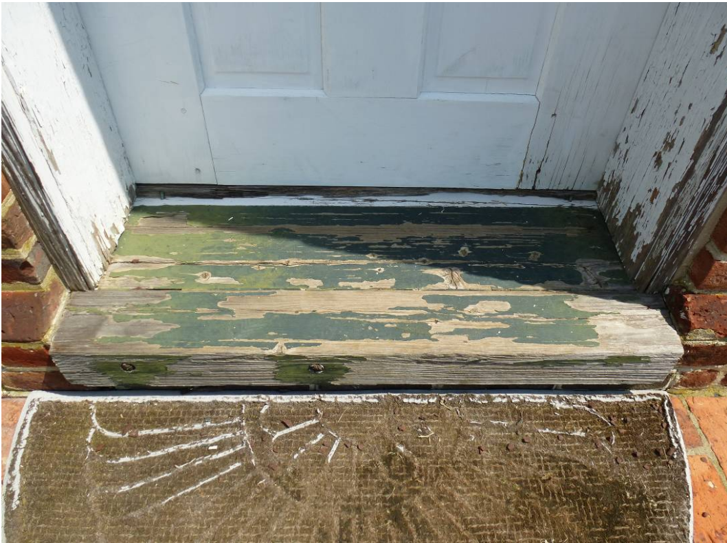
Figure 102. Wood threshold for the main door with chipped paint (ERDC-CERL, 2012).
