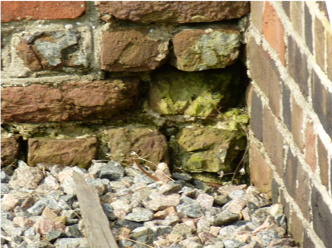
Figure 79. Deteriorated brick caused by the water that splashes off of the large gravel. This type of deterioration is called erosion (ERDC-CERL, 2012).
