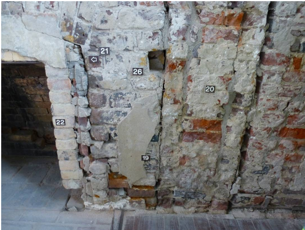
Figure 135. Feature #19 points out fireplace opening for Period I; #20 is original masonry jamb; #21-is fireplace opening in Period II; #22-is fireplace opening in Period III; and #26 shows pockets for Period II mantel blocking (ERDC-CERL, 2012).
