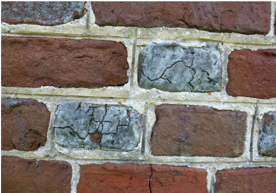
Figure 60. Glazing on header bricks is failing due to the evidence of crazing effects within brick (ERDC-CERL, 2012).
