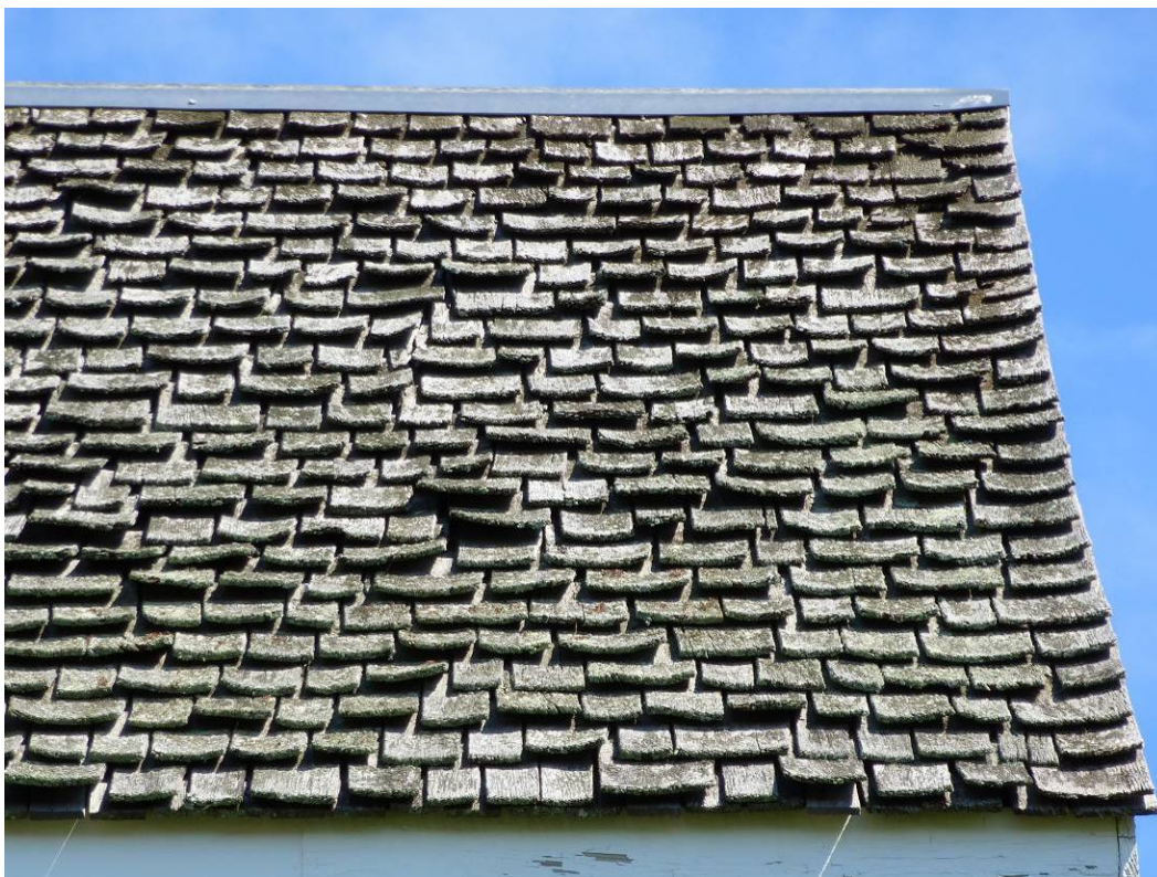
Figure 30. Wood shingle roof on main block gable, porch tower gable, and shed room (rear chamber) roof (ERDC-CERL, 2012).
