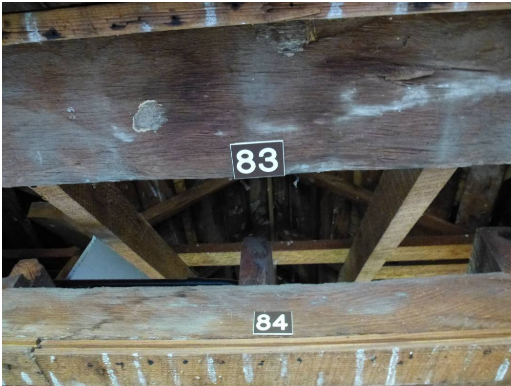
Figure 167. Some of the last remaining eighteenth-century framing in the house. These joists were set in place during the construction of the porch tower ca. 1730. They are made of oak and are hewn and pit sawn (ERDC-CERL, 2012).
