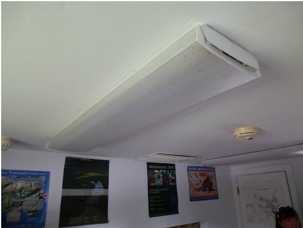
Figure 181. Addition of fluorescent tube lighting the second-floor chamber over the dining that is now being used for office space (ERDC-CERL, 2012).
