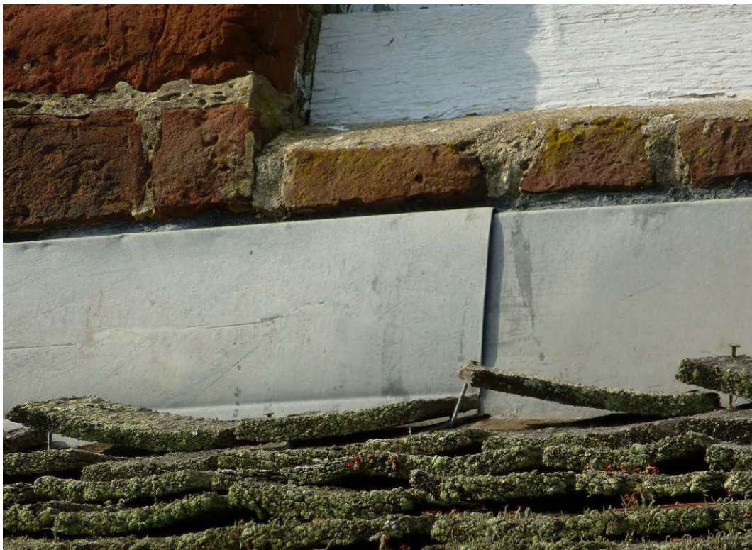
Figure 94. Flashing at the joint of the shed roof and brick wall of main block (ERDC-CERL, 2012).
