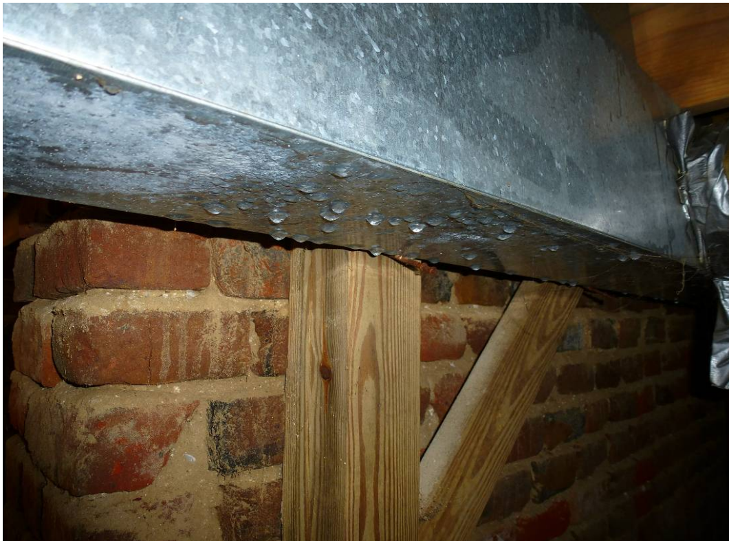
Figure 215. Condensation is visible on the HVAC equipment in the cellar (ERDC-CERL, 2012).
