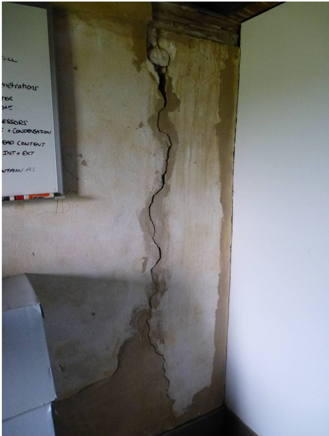
Figure 195. Long vertical crack in plaster. Located in the upper chamber room on the southeast (now office) over the dining room (ERDC-CERL, 2012).
