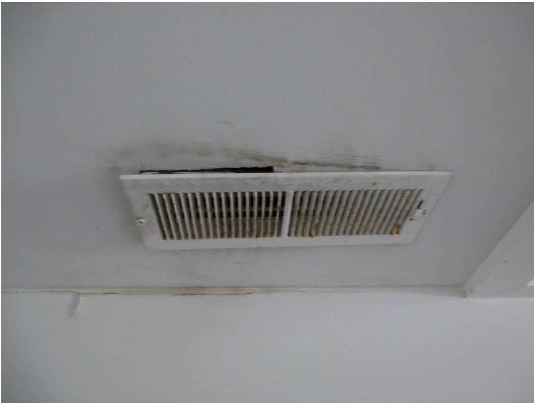
Figure 223. Ceiling vent in the second-floor chamber above the dining room. Vent is not properly attached, and mold is evident (ERDC-CERL, 2012).
