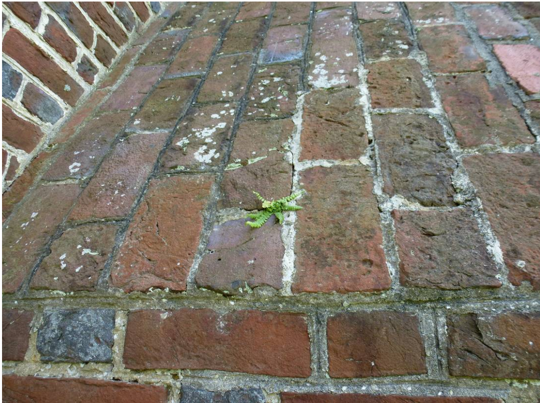
Figure 75. Vegetation growth on chimney brickwork (ERDC-CERL, 2012).
