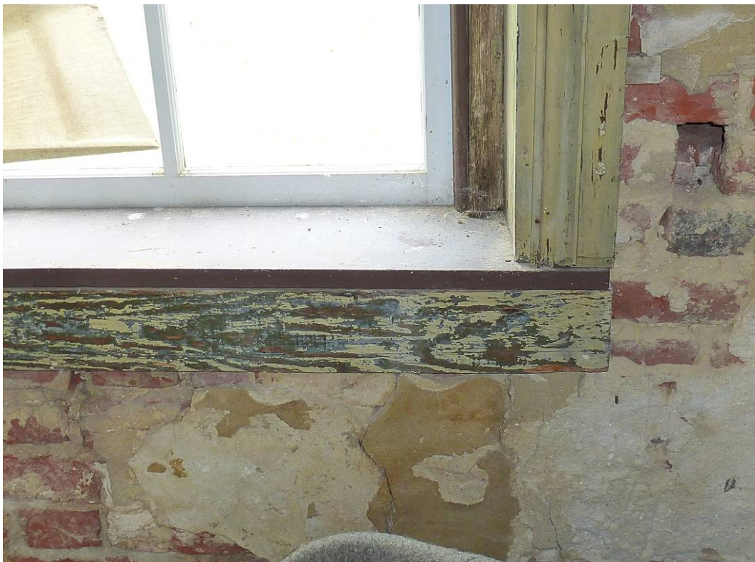
Figure 206. Paint is failing on the wood window trim (ERDC-CERL, 2012).
