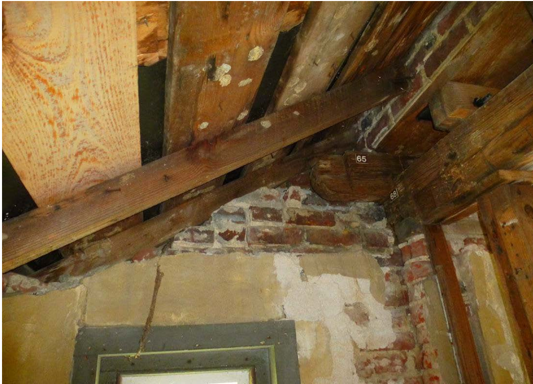
Figure 164. The only original end joint that has not been removed (#65) is located on the northeast wall, visible in the shed room (rear chamber) addition (ERDC-CERL, 2012).
