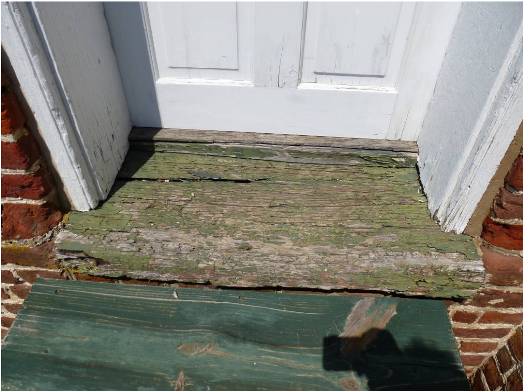
Figure 105. Deteriorated wood threshold for the side door is too damaged for repair and needs to be replaced (ERDC-CERL, 2012).
