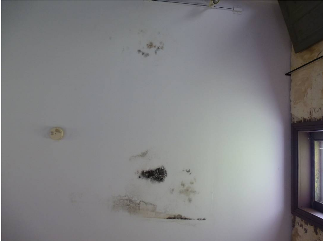
Figure 218. Looking up at mold on the ceiling above the hall (ERDC-CERL, 2012).
