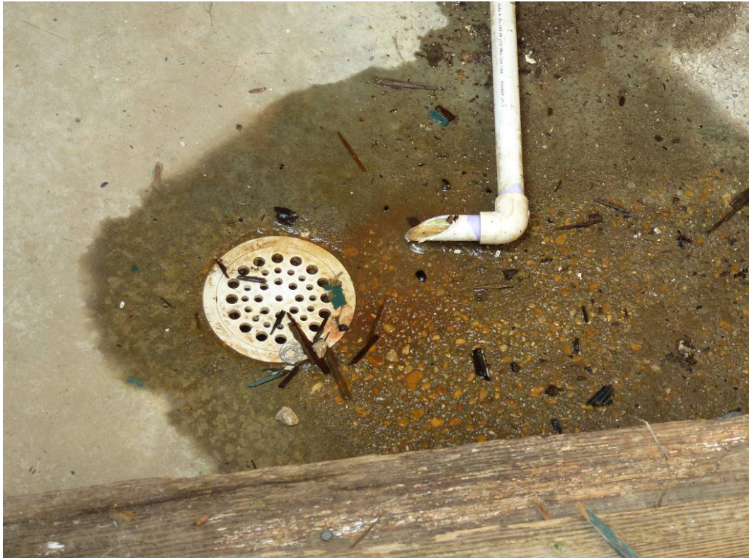
Figure 225. Water is being allowed to pool on the concrete cellar floor. The pipe is coming from the HVAC unit but does not meet the drain in the floor (ERDC-CERL, 2012).
