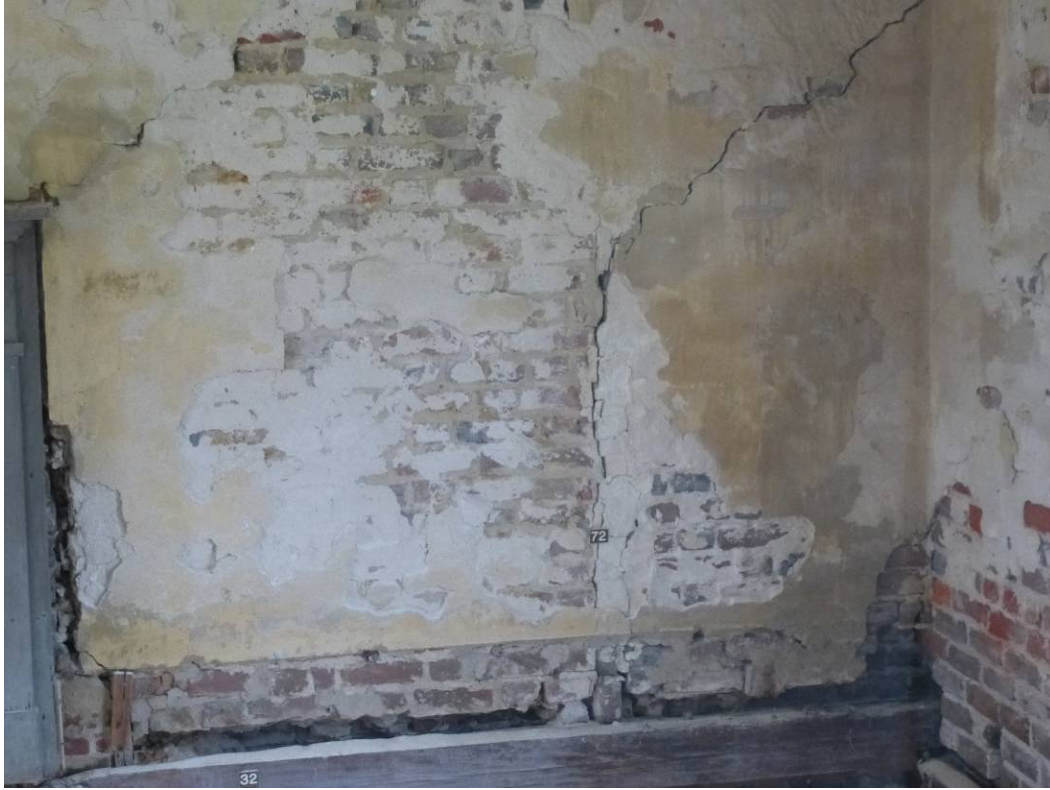
Figure 194. Vertical cracks in the plaster flanking the fireplace are Period I features caused by knee wall studs, left in place during both the ca. 1730 and 1893 renovations. They were plastered over in 1893 and are represented here by cracks in the plaster (ERDC-CERL, 2012).
