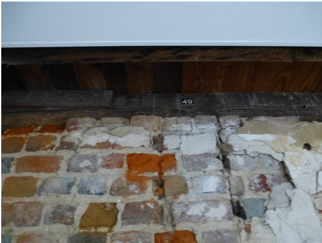
Figure 161. End joist in dining room indicated by #49 (ERDC-CERL, 2012).
