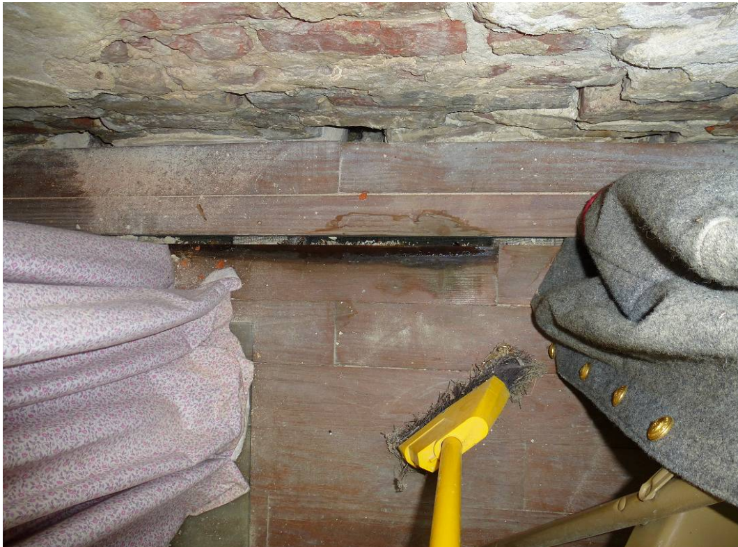
Figure 219. The moisture from the HVAC system is causing the floorboards in the hall to become wet (ERDC-CERL, 2012).
