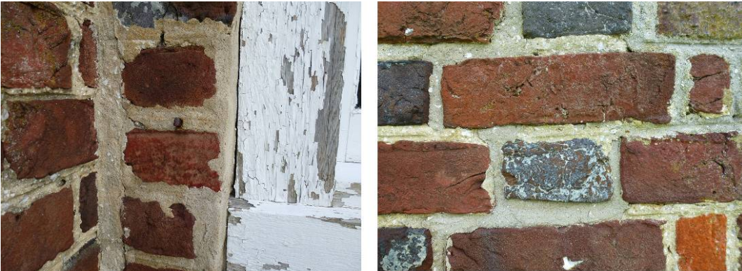
Figure 66. Examples of poor craftsmanship with replacement mortar (ERDC-CERL, 2012).
