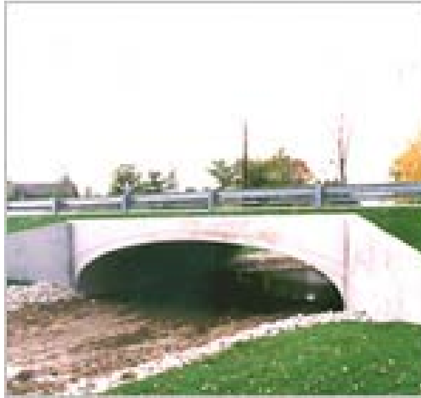
Figure 3 Similar Bridge Construction to Proposed Action
