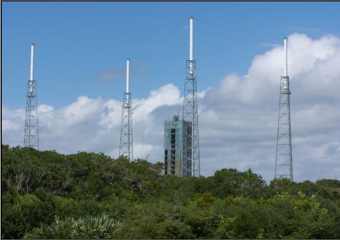
Facility 47141: Lightning Suppression System
