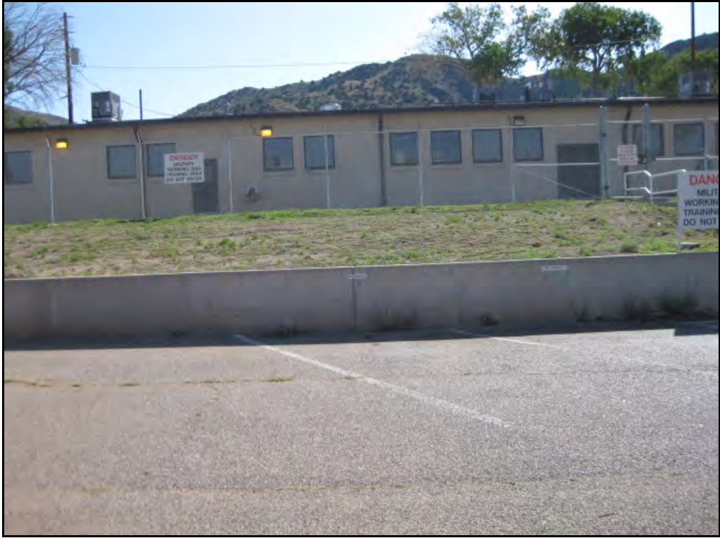
C1. Existing MWD Facility, Building 30126
