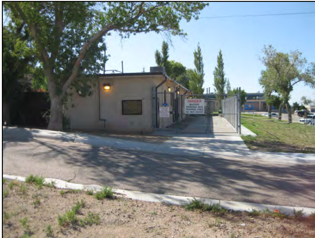
C2. Existing MWD Facility, Building 30126
