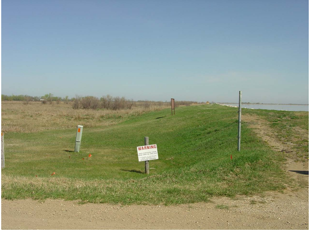
Figure 2.3 Photo of 47 acre palustrine/lacustrine wetland system # LS-02 looking north along the west edge of the lagoon primary cell one
