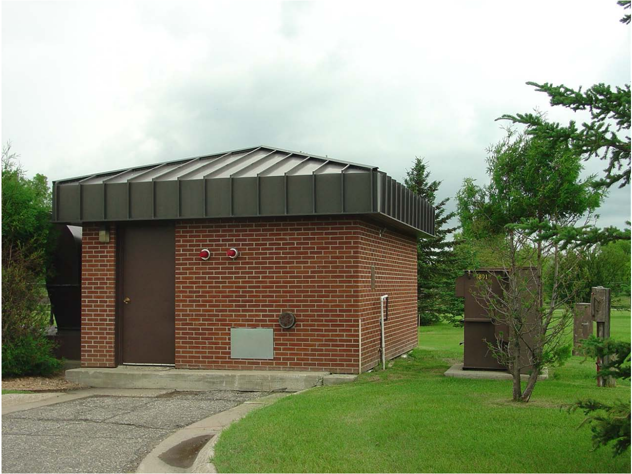
Figure 2.5 Photo of Building 801, the lift station at the main gate of Grand Forks AFB
