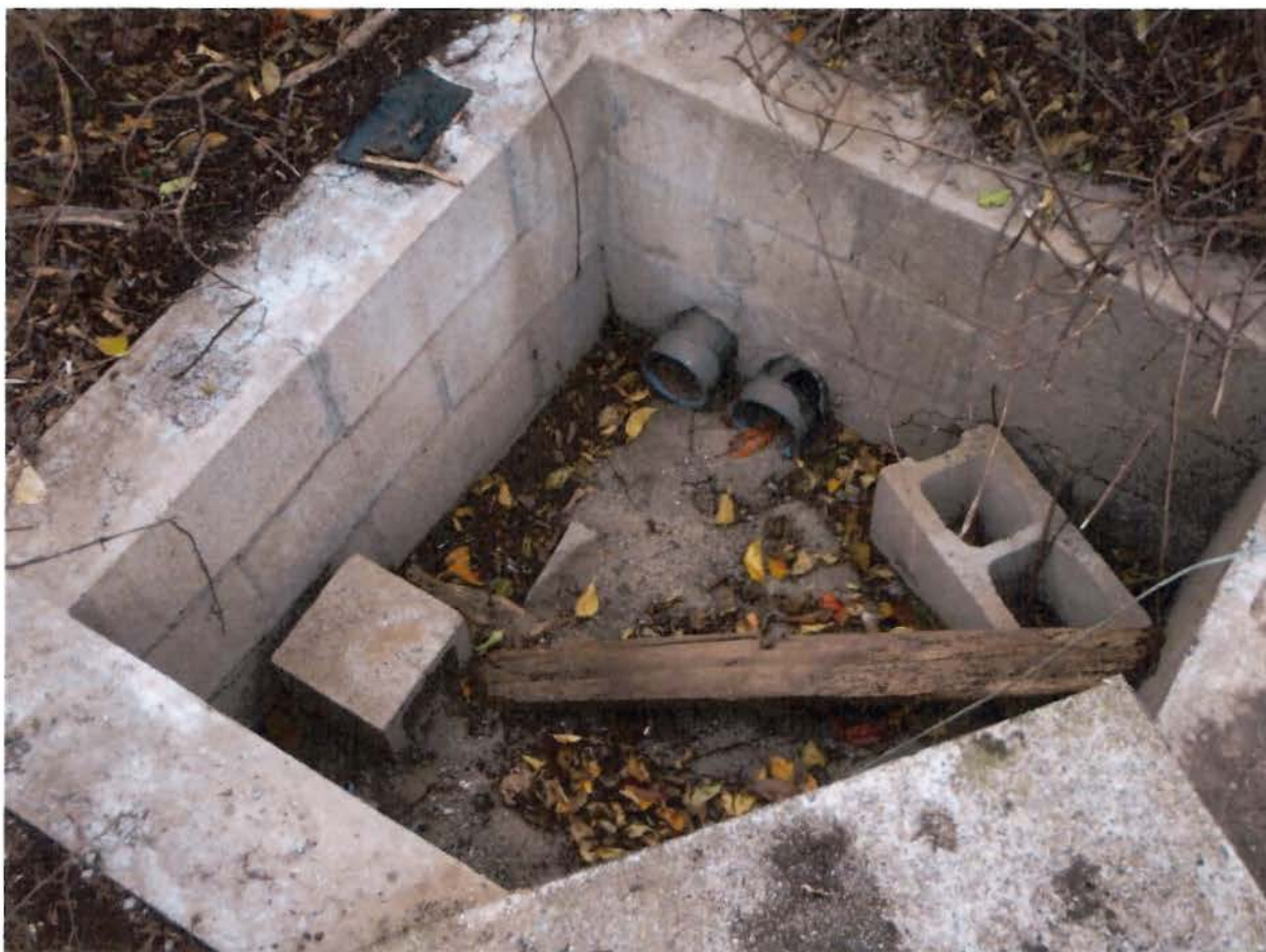
ELECTRIC HAND HOLE ALONG SERVICE ROAD "E"
