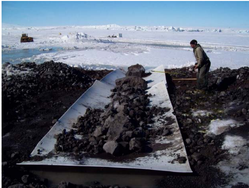
Figure 5. The fines and plastic are installed, and the large rock is placed along the center of the drain.
