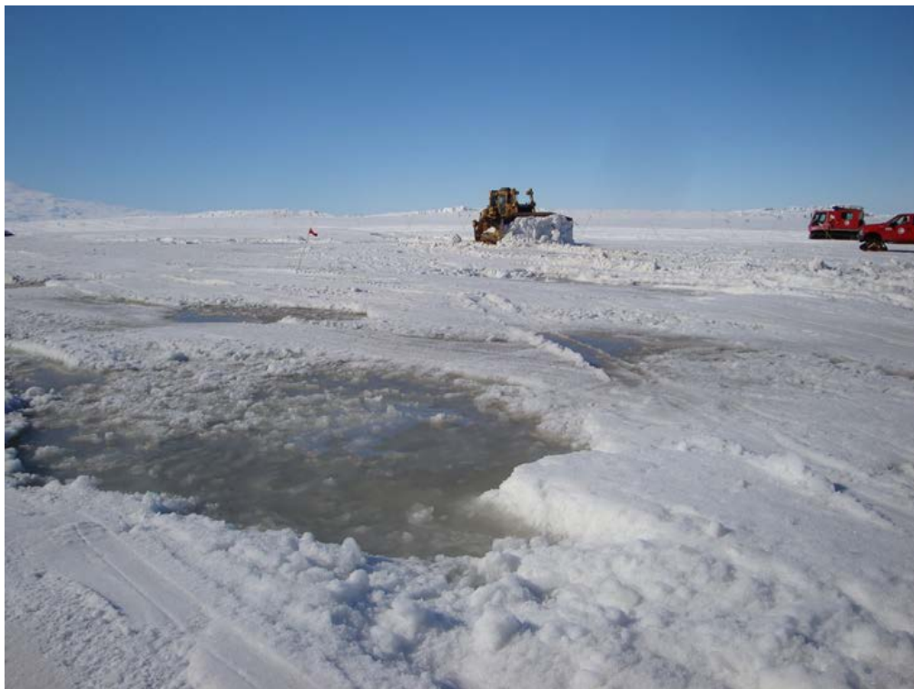
Figure 24. Melt pools requiring maintenance on the Ice Transition.
