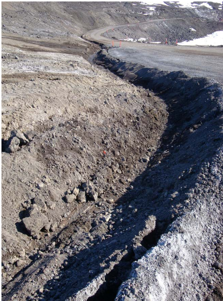
Figure 3. Upslope drainage ditches along the Land Transition of the SBT.
