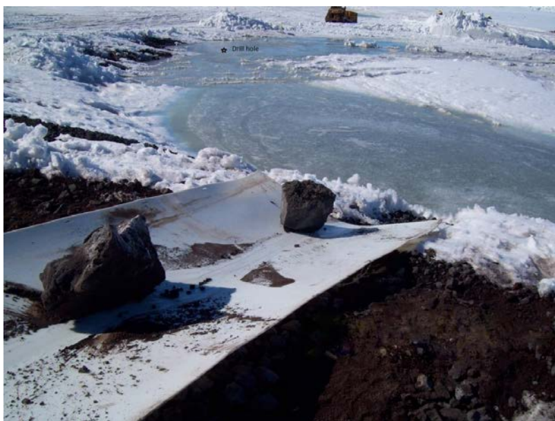
Figure 6. The plastic sheet forms an outlet to protect the Land Transition's side slope from settlement and erosion.
