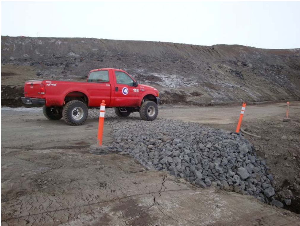
Figure 8. Unlined french drain crossing built with clean-off rock only.
