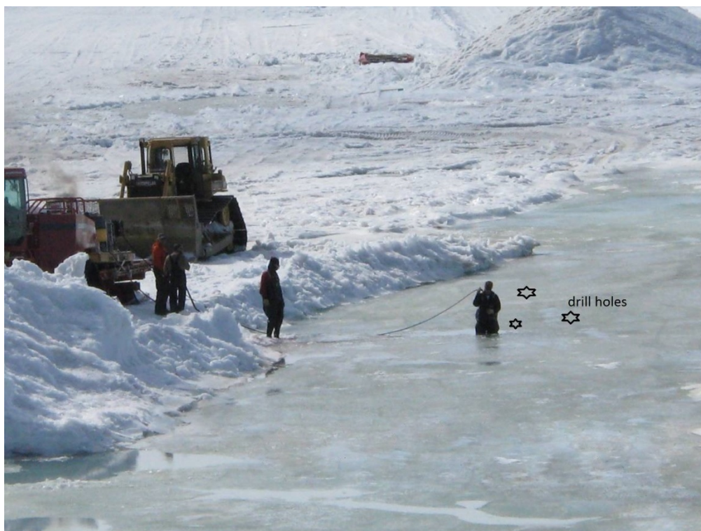
Figure 19. Hot water drilling to drain the retention ponds.
