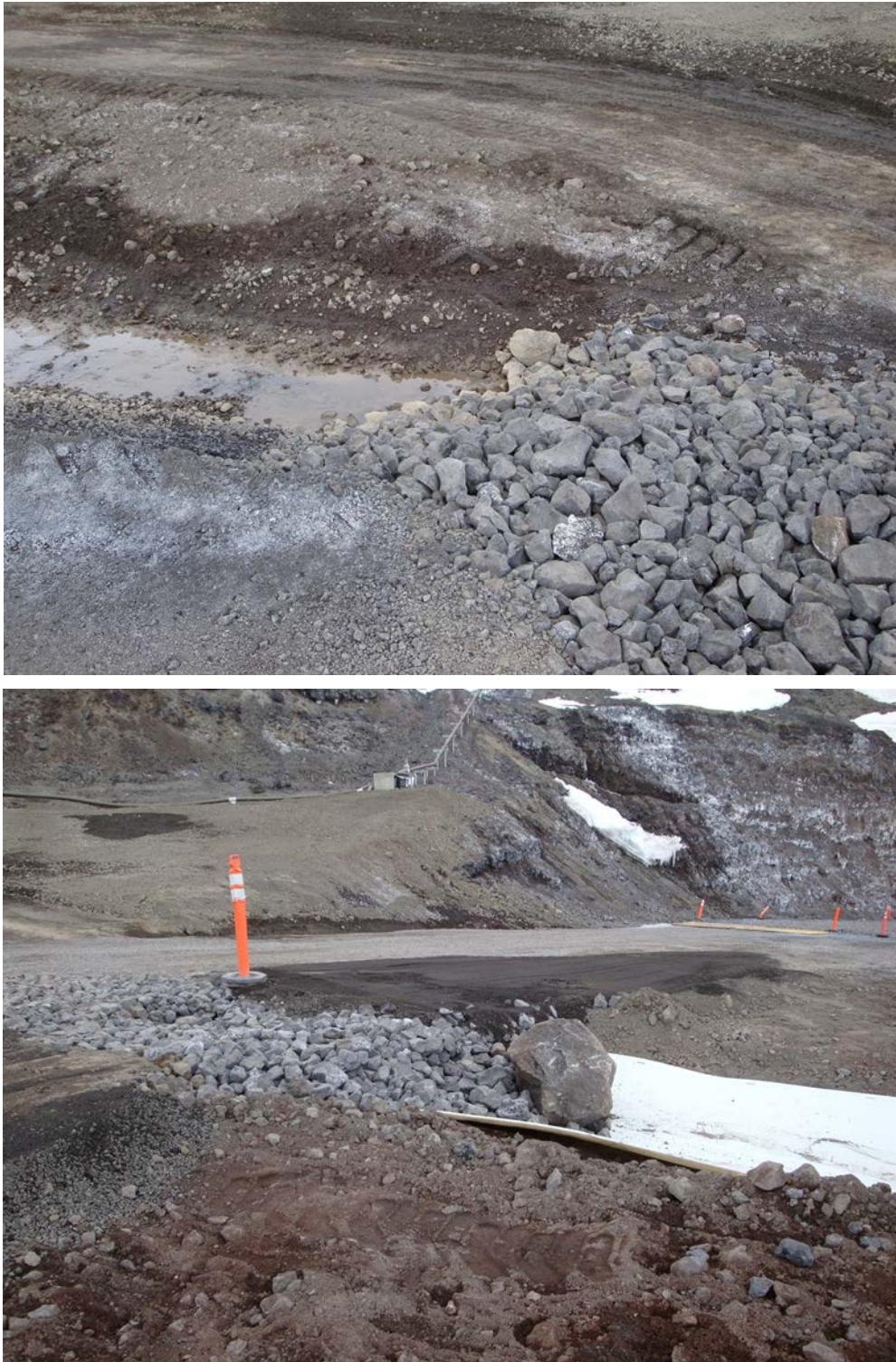
Figure 7. The finished Antarctic drain inflow (top) and outflow (bottom).
