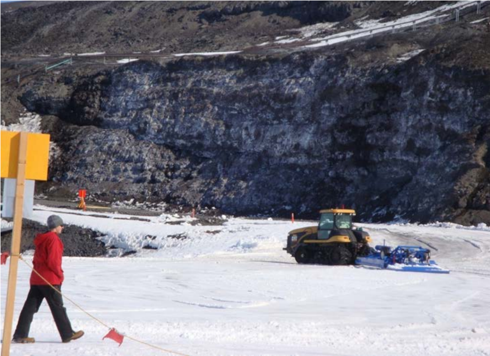
Figure 26. The Keweenaw Research Center SnowPaver mixes and compacts the wet snow at the SBT (January 2012).
