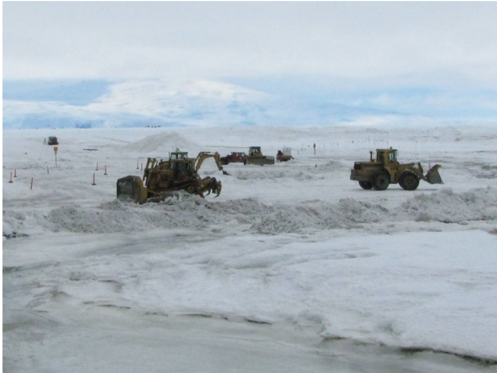
Figure 25. Scraping, ripping, and patching the rest of the Ice Transition after stabilizing the primary lanes.
