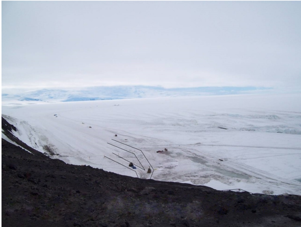
Figure 22. Continued construction during the 2010–2011 season.
