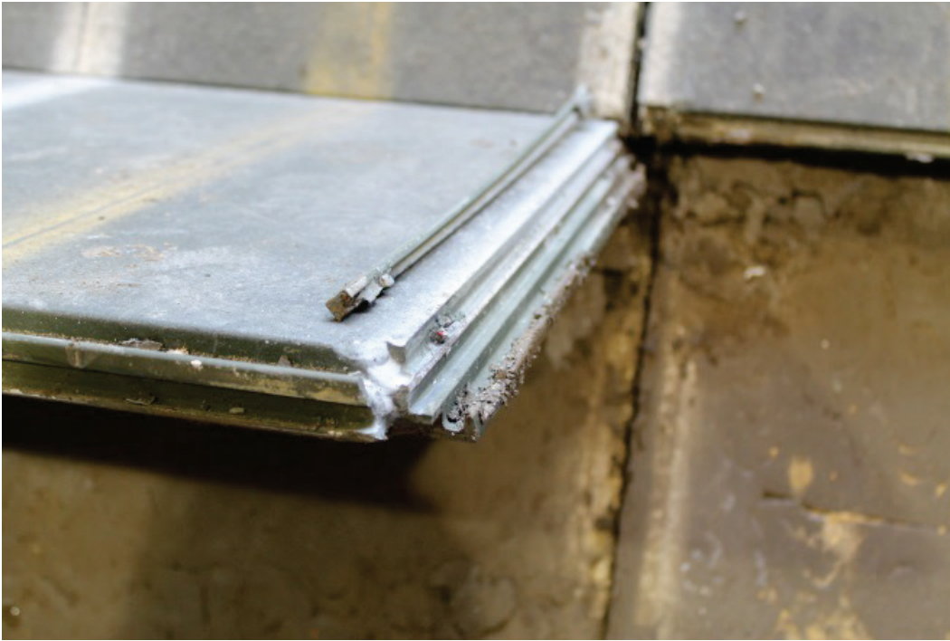
Figure 32. Typical broken upper underlap rail.
