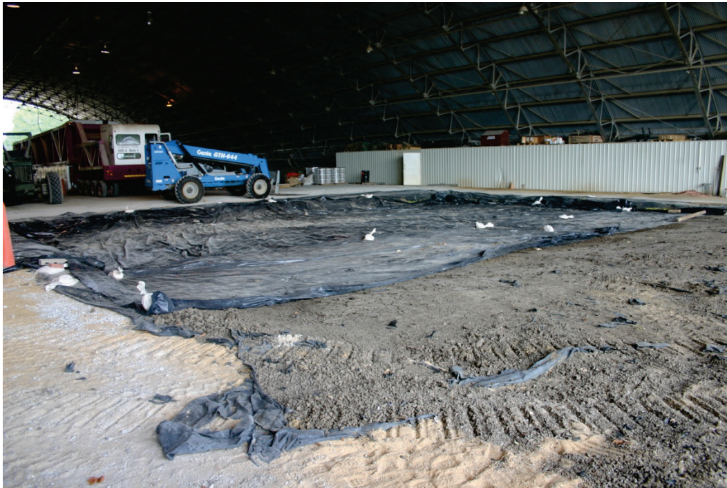
Figure 8. Test pit lined with impervious sheeting.
