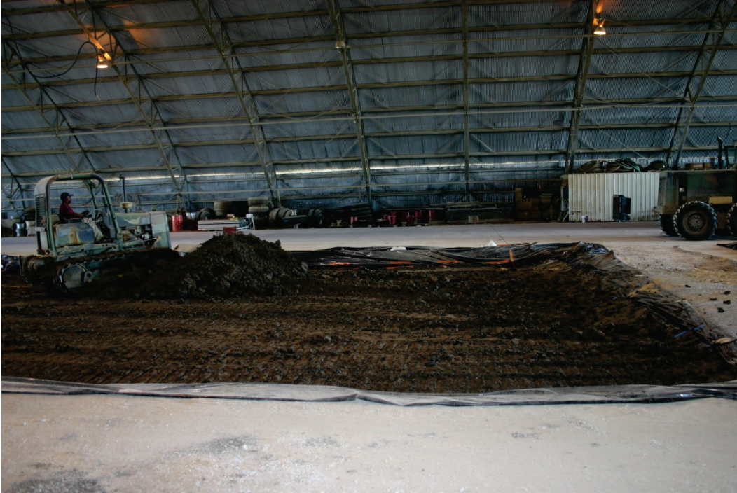
Figure 12. Leveling CH material in test pit prior to compaction.
