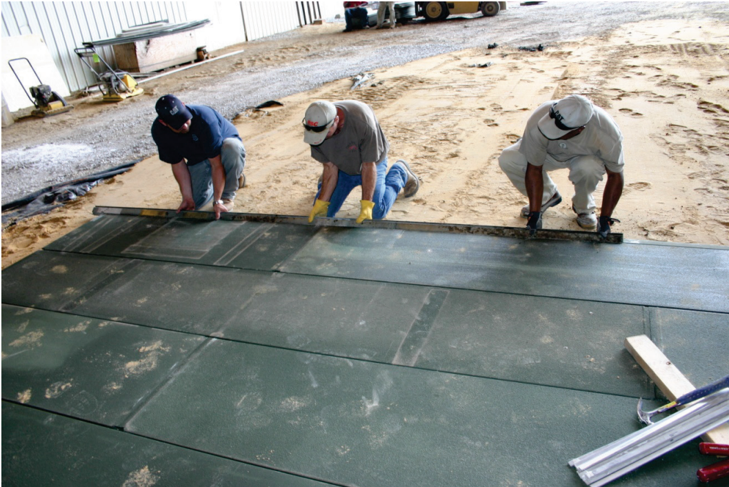
Figure 21. Typical Installation of male keylock.
