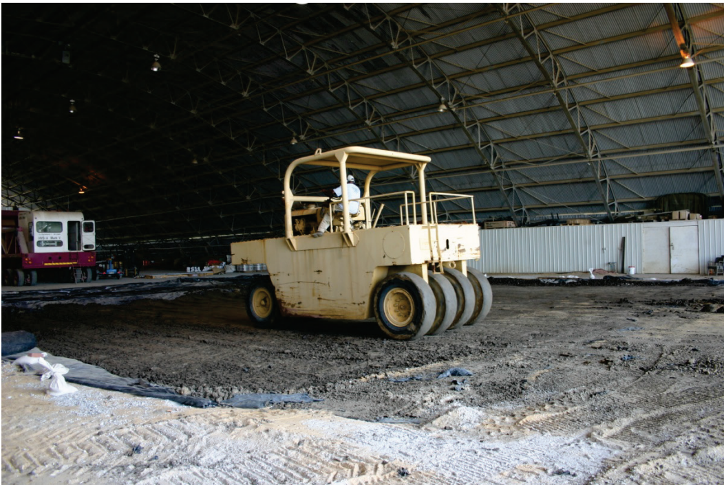
Figure 13. Compacting CH subgrade with pneumatic roller.
