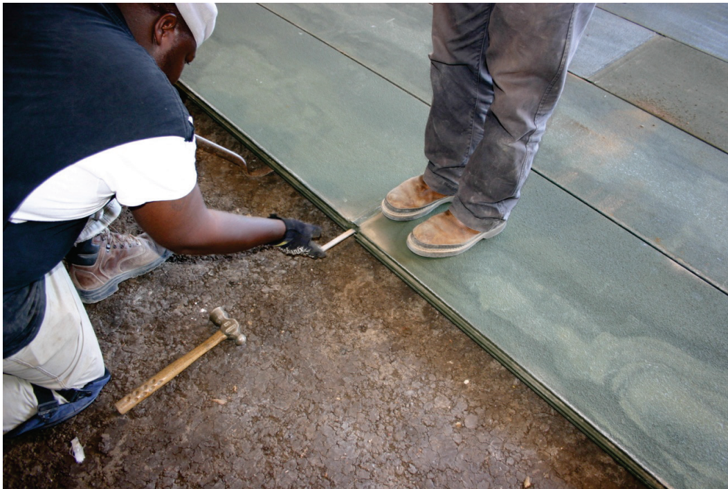
Figure 19. Insertion of aluminum locking bar between adjacent panels.
