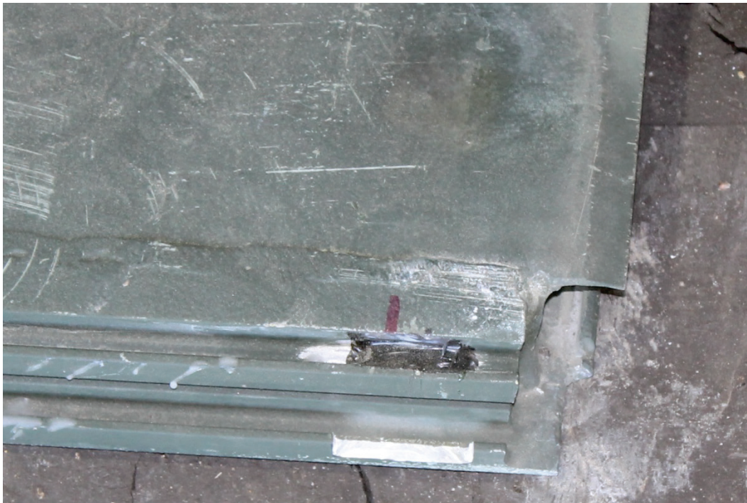
Figure 17. Typical strain gauge installation on lower overlap region of AM2 panel end connector.
