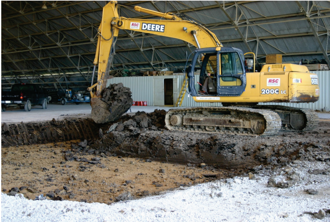
Figure 7. Test section excavation.
