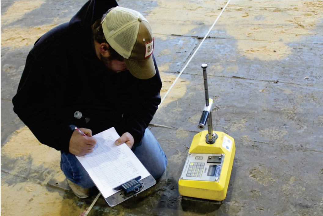
Figure 14. Nuclear moisture-density gauge test.
