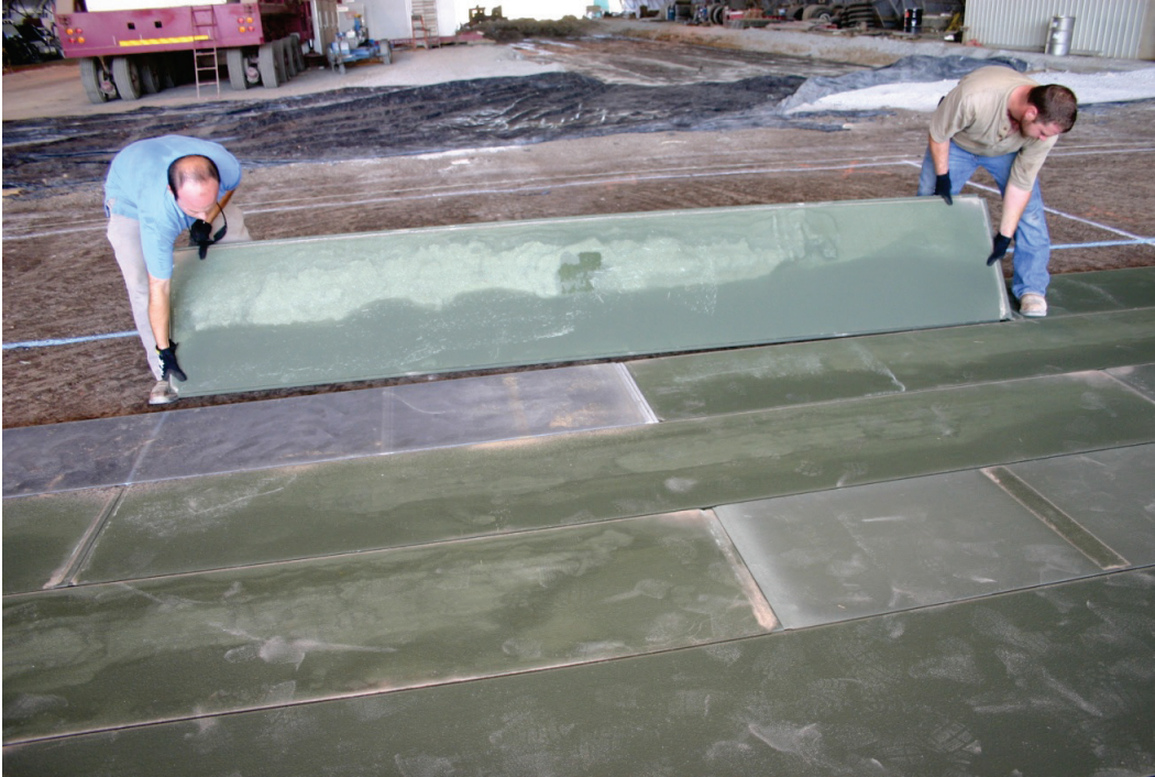
Figure 20. Installation of AM2 panels on the test section subgrade.
