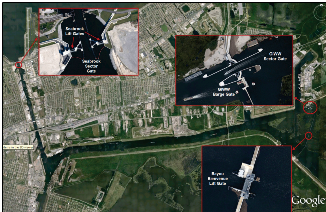
Figure 17. Gate structures included in the alternative conditions.
