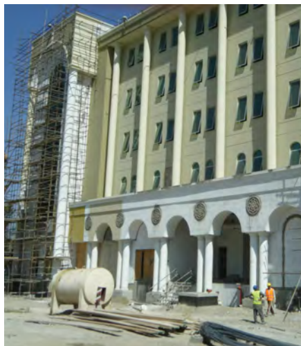
Ministry of Defense Headquarters Building under construction in Kabul, September 2014. (CSTC-A photo)
