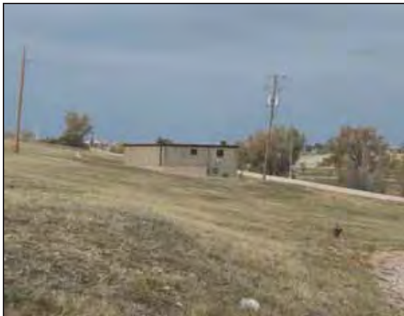
Building 3015 – O/W Separator
