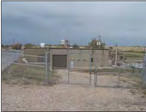
Building 3013 – Pretreatment Facility
