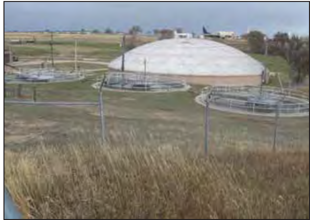
Building 3010 – Trickling Filter
