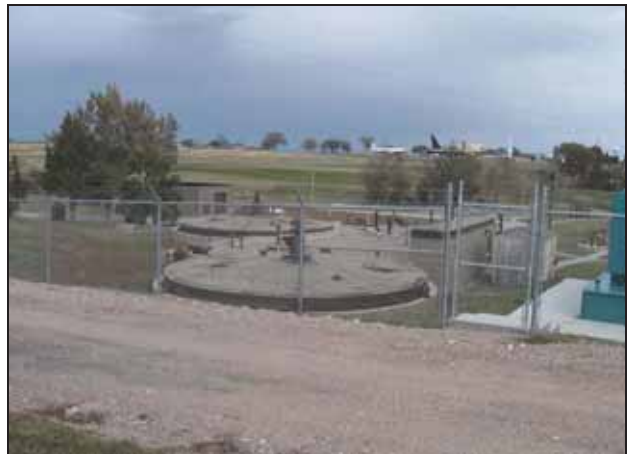
WWTP Facilities Adjacent to Building 3007
