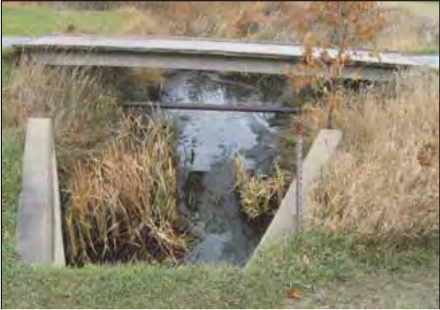
Outfall 005 to Unnamed Creek
