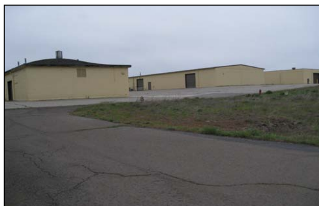
Figure 2.2 Photograph of a portion of the area to be demolished i.e., Buildings 1462, 1460, and 1458, associated concrete pads and asphalt access road.
