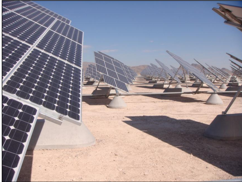
Figure 4-3 PV Solar Array at Nellis AFB
