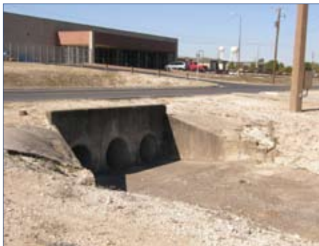
Storm Water Culverts
