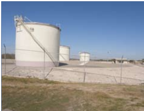
Fuel Storage Tanks
