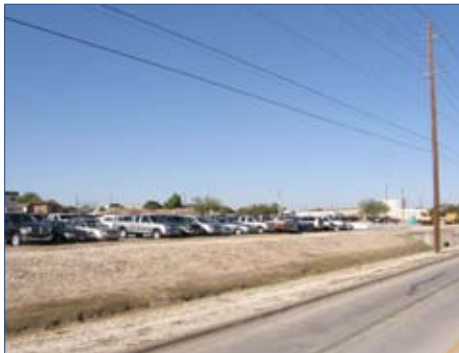
Storm Water Channel along Second Street
