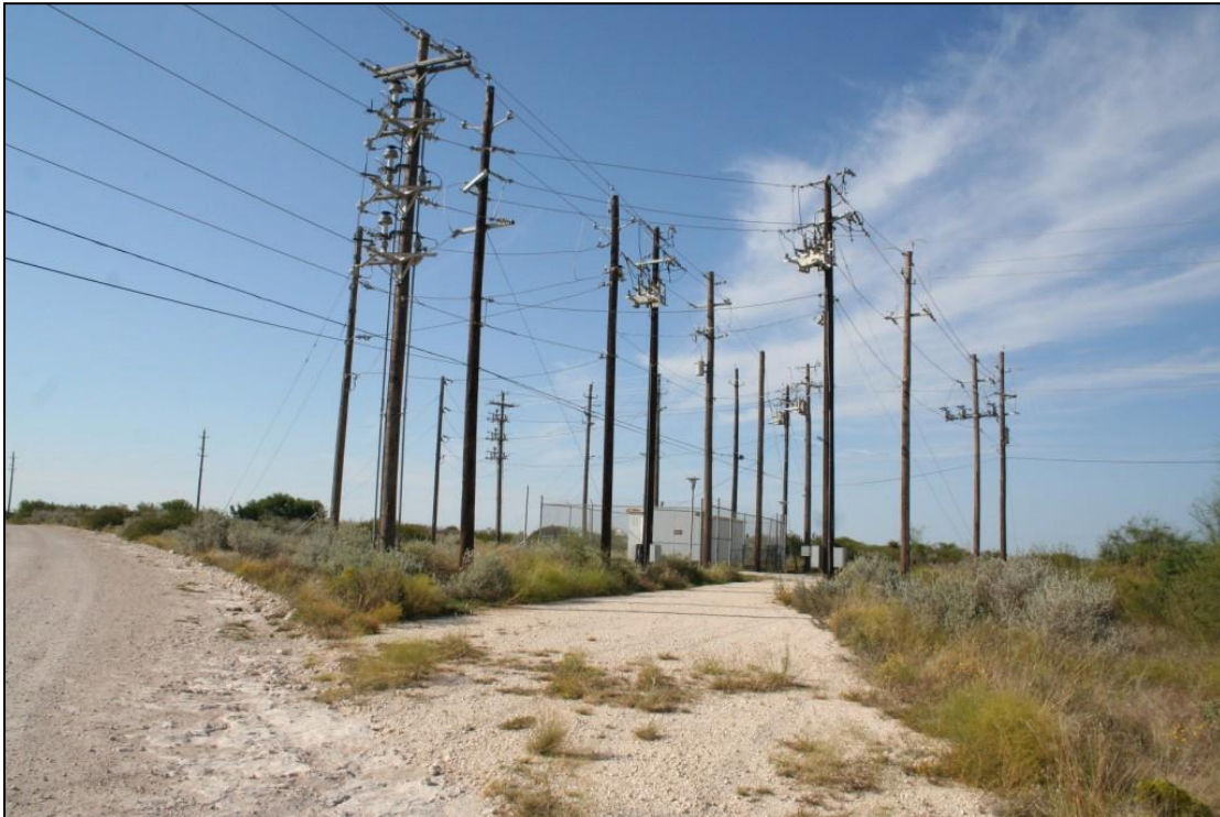
Figure 4-5 Overhead Electromagnetic Interference Sources
