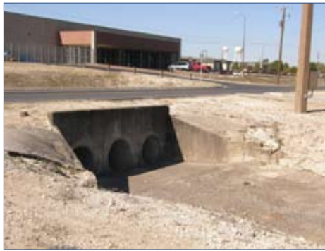
Storm Water Culverts
