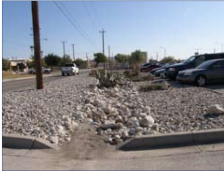
Storm Water Drainage
