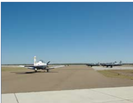
Concrete and Asphalt Pavements on Airfield
