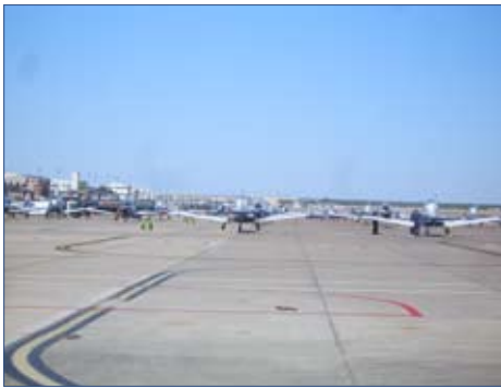
Concrete Parking Apron
