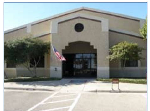
47th Installation Support Squadron Building
