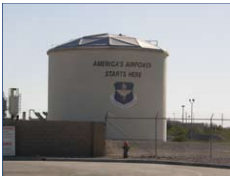
Jet Fuel Storage Tank
