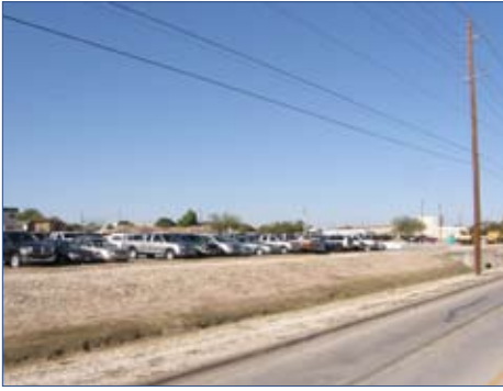
Storm Water Channel along Second Street
