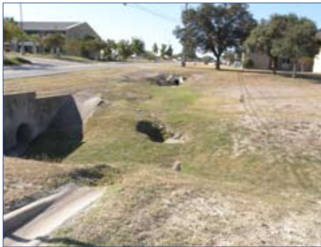
Storm Water Culverts
