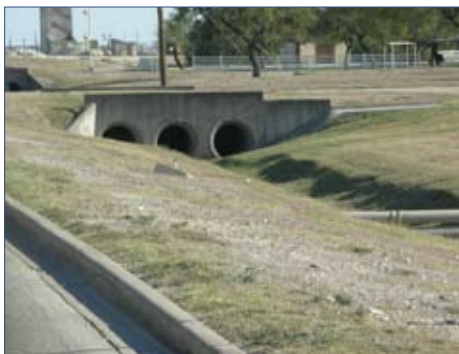
Storm Water Culverts
