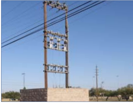
Overhead Power Lines
