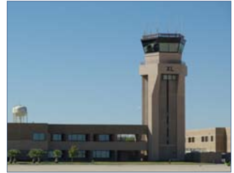
Air Traffic Control Tower
