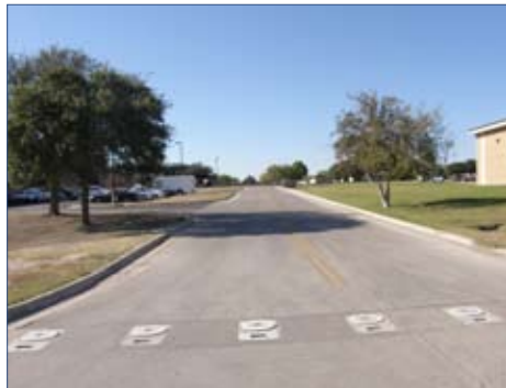
Automatic Bollard System
