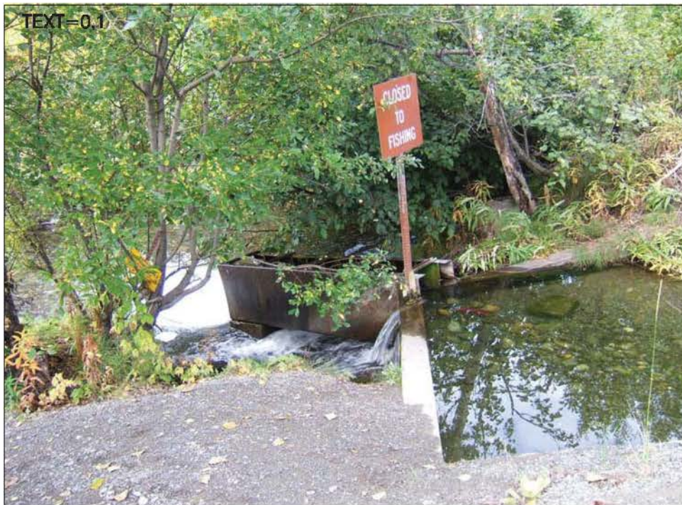
EXISTING SIXMILE CREEK FISH LADDER (UPSTREAM VIEW)
