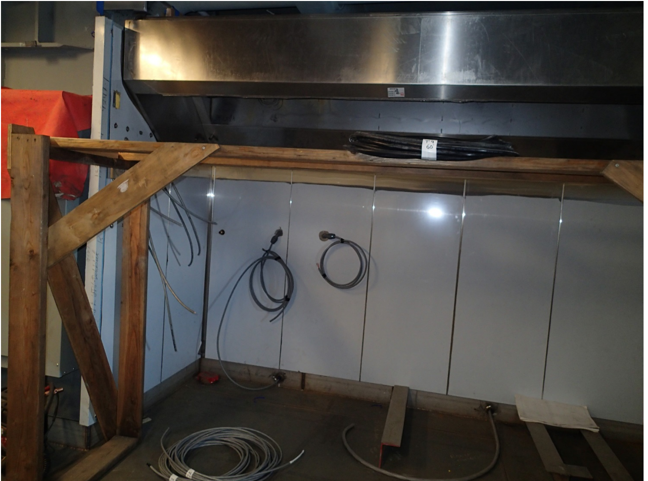
Galley range hood with panels & wiring
