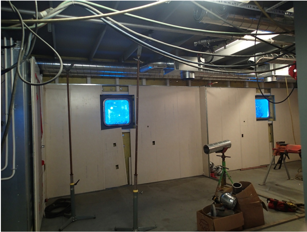
Foc'sle Deck Joiner work
