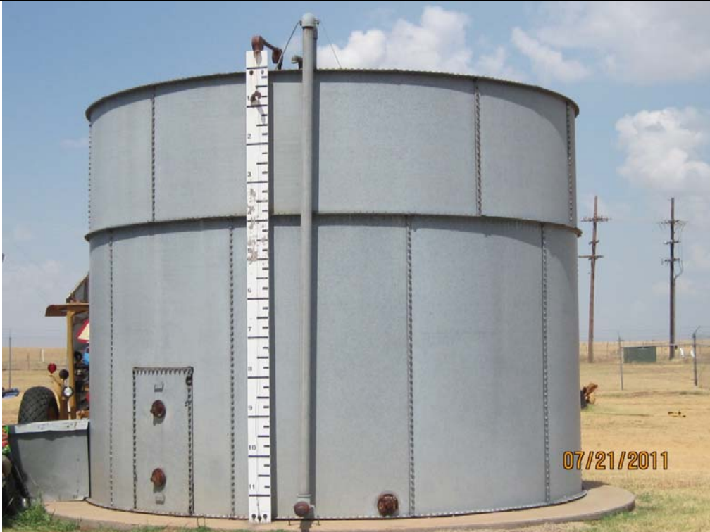
Photo 2: Water Tank for Demolition
