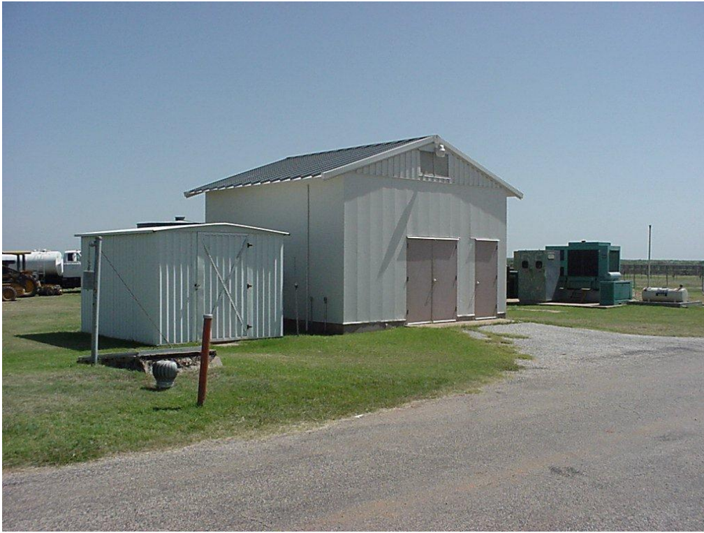
Photo 1: Storage Sheds for Demolition
