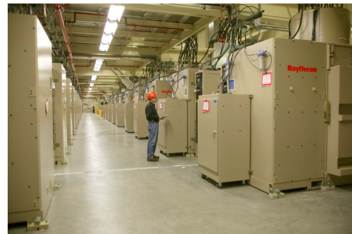
Figure 1. Completed Capacitor Bay with 48 modules, capable of storing ~100 MJ of electrical energy for flashlamps.
