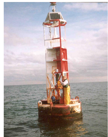
Figure 4. USCG buoy serves as a FRONT gateway buoy.
