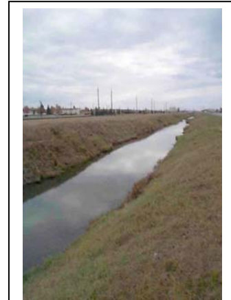
Garrison Slough is channelized where it passes through the BDA. Bank height provides an indication of the thickness of fill material built-up within the BDA.
