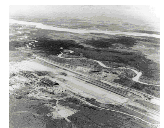
Eielson in 1945. Eielson's airfield and developed areas are constructed on fill material deposited in cleared forest wetlands.
