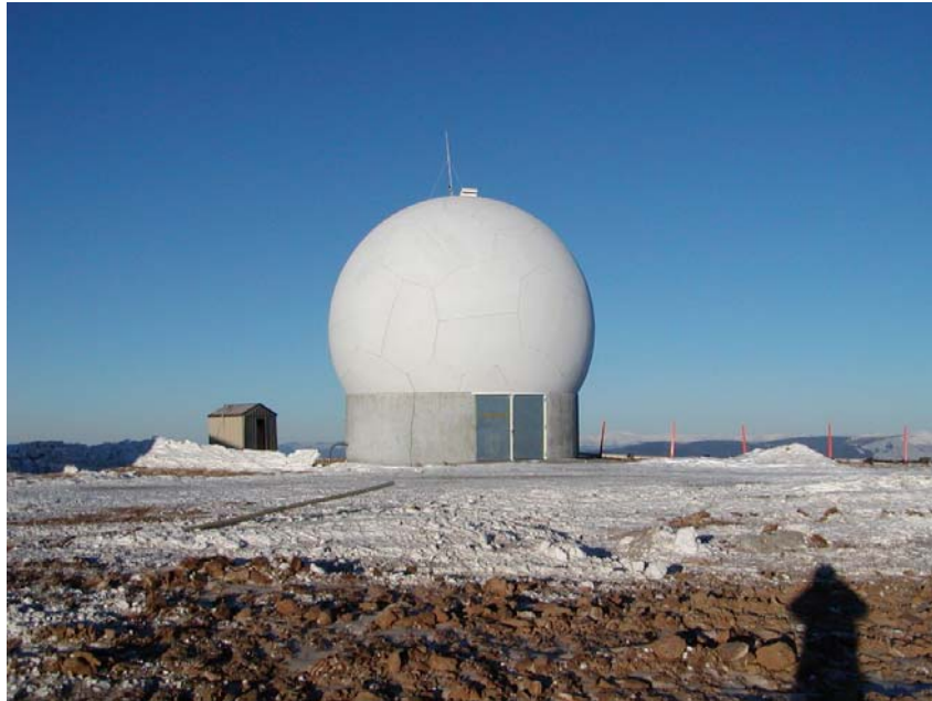
Photograph 1 – Typical Radome Structure
