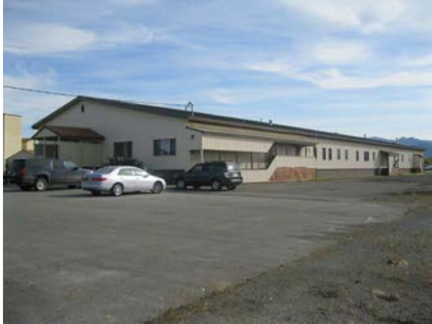
Photo No. 9 – Building 5312 – 8/29/2012 Southwest corner
