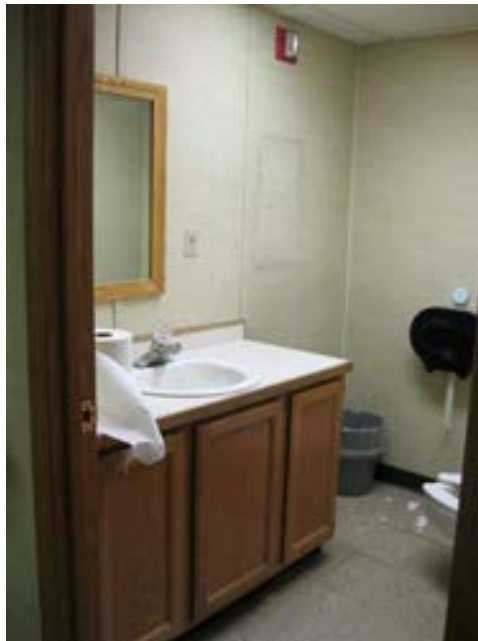
Photo No. 6 – Building 5303 – 8/29/2012 Western (partitioned) portion – bathroom
