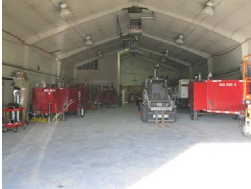
Photo No. 3 – Building 5303 – 8/29/2012 Eastern portion of building
