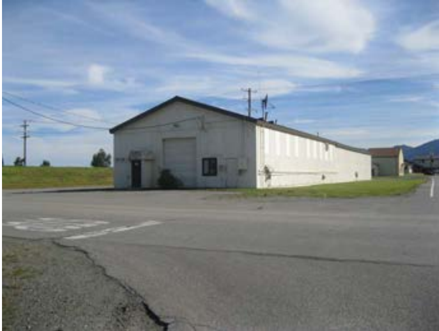
Photo No. 1 – Building 5303 – 8/29/2012 Southwest corner
