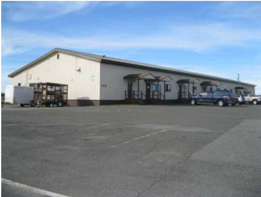
Photo No. 10 – Building 5312 – 8/29/2012 Northeast corner
