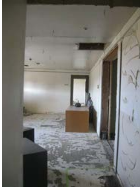
Photo No. 11 – Building 5312 – 8/29/2012 Eastern portion of Building #1
