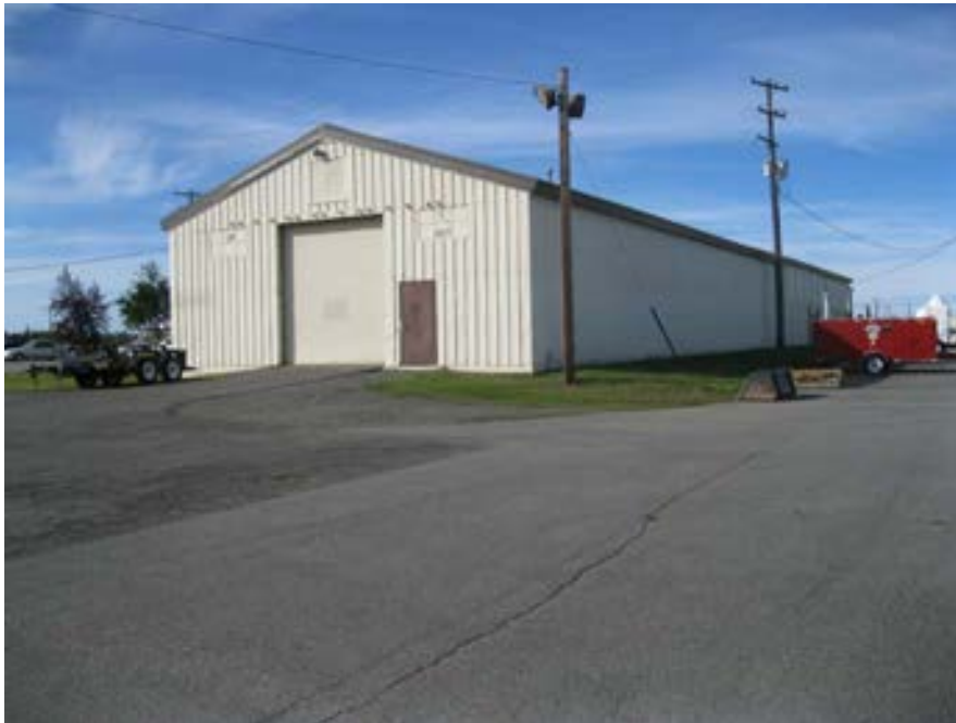
Photo No. 2 – Building 5303 – 8/29/2012 Northeast corner
