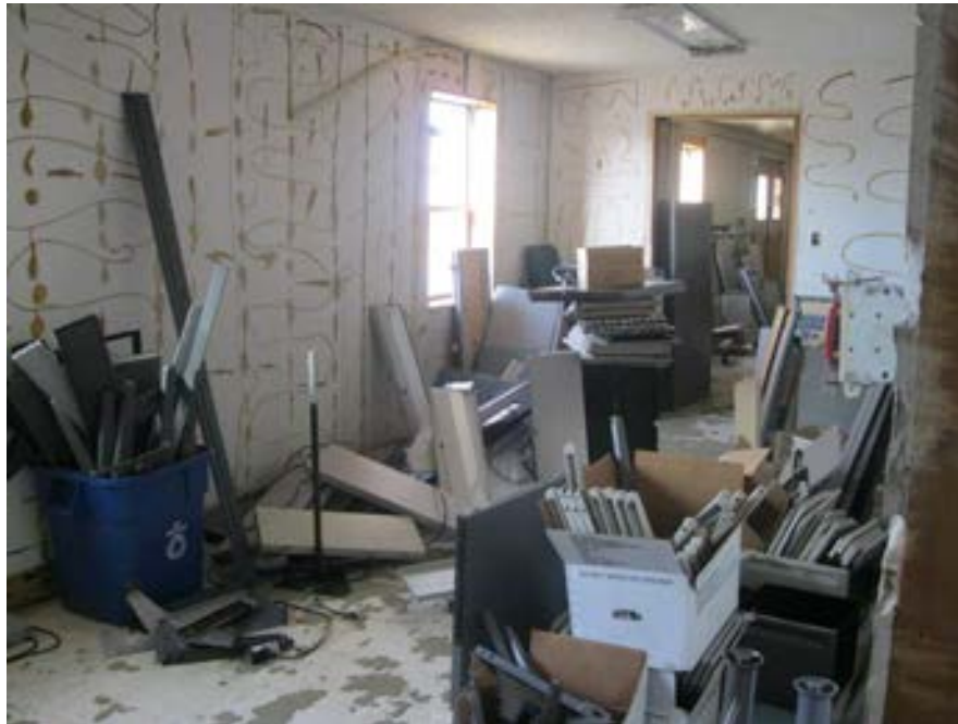
Photo No. 12 – Building 5312 – 8/29/2012 Eastern portion of Building #2
