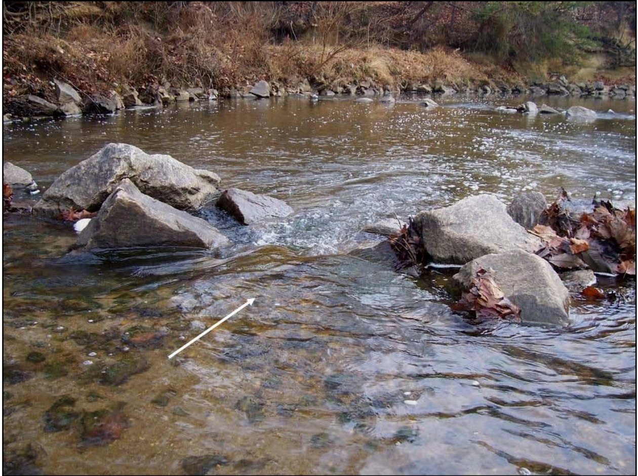
Figure 19. Close-up of crest of bendway weir 2, 14 January 2008 (10 years after construction). Mini plunge pool, aeration, structure, hydraulic cover and solid stable substrate for benthic invertebrates.
