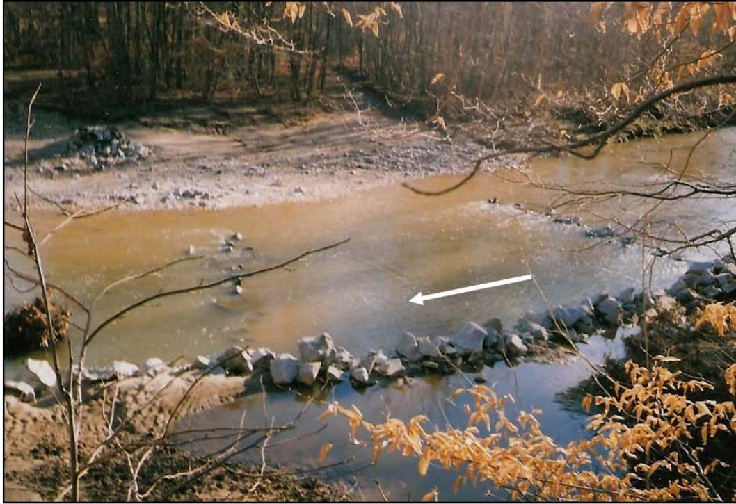
Figure 12. Mid-project from cliff looking at LPSTP and weirs 2 and 3, 1 February 1998 (5 months after construction). Note: low area and water landward of LPSTP.
