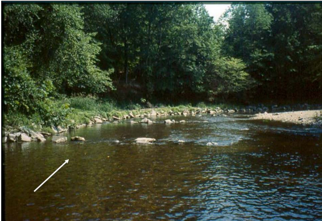
Figure 10. Looking downstream at bendway weirs 1-3, 17 May 2000 (2.75 years after construction).
