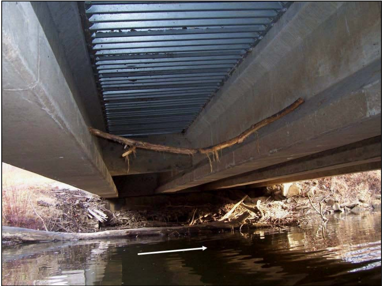
Figure 6. Undersized bridge opening, Panther Bridge at downstream end of project (branch stuck up under bridge).
