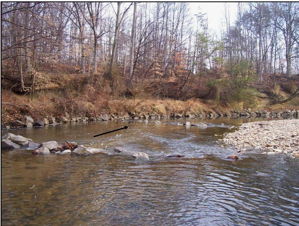
Figure 18. Closer view of stream end of bendway weir 3, 14 January 2008 (10 years after construction). In addition to surface disturbance and aeration there is great diversity and complexity of velocities, depths, and subsubstrate (sand patches within cobble-gravel) within weir field.
