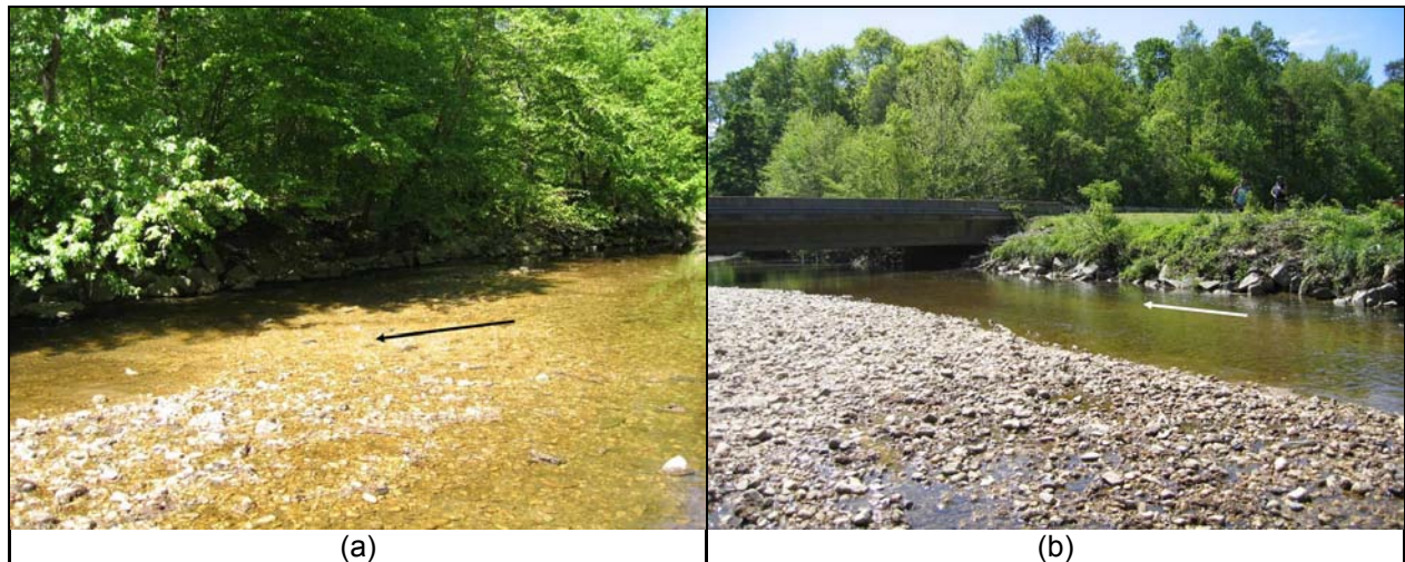
Figure 16. Right descending bank upstream of Panther Bridge, 1 May 2006 (8.75 years after construction). PSTP, mostly hidden, still protecting trees a decade after installation. (a) Looking upstream. (b) Looking downstream.
