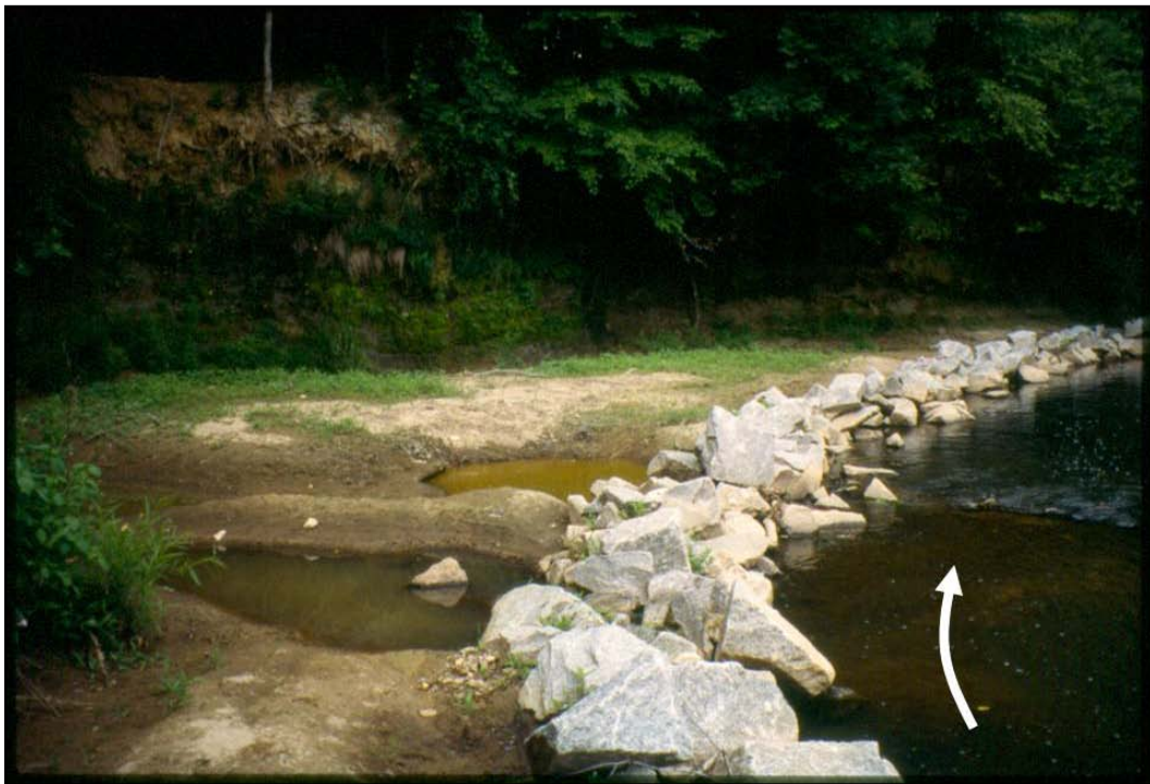
Figure 13. Looking downstream at new deposition landward of LPSTP at weir 3, 8 June 1998 (9 months after construction).
