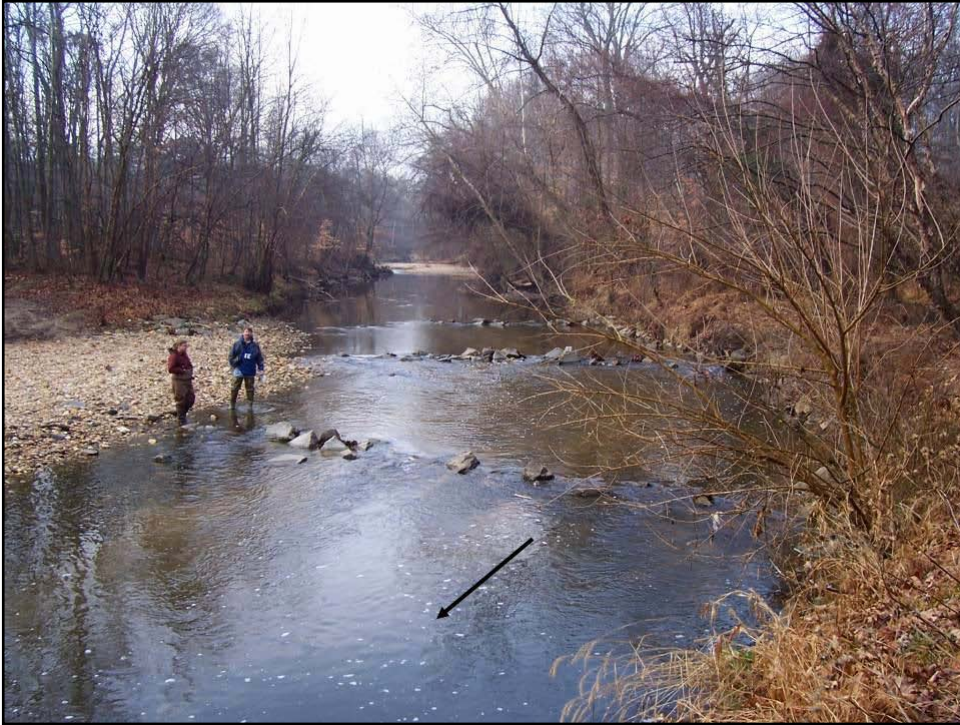
Figure 20. Looking upstream at bendway weirs 1-3 (10 years after project completion, 14 January 2008). Banks are stable.
