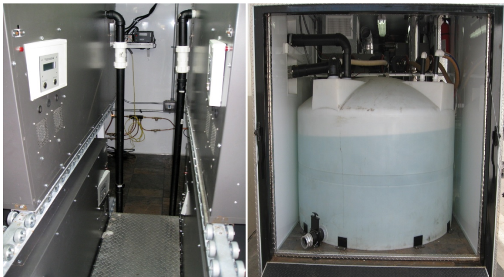
Figure 8. Four burner chambers inside the incinerator and control panels that were upgraded (left) and waste water storage tank with upgraded piping and feed pumps (right).
