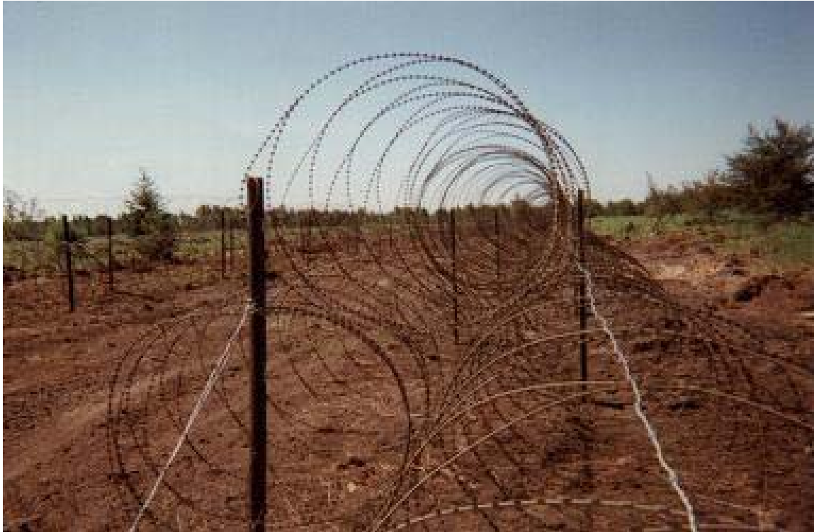
Figure 2-10. Example of Wire Configuration Used for a PoW Camp Perimeter
