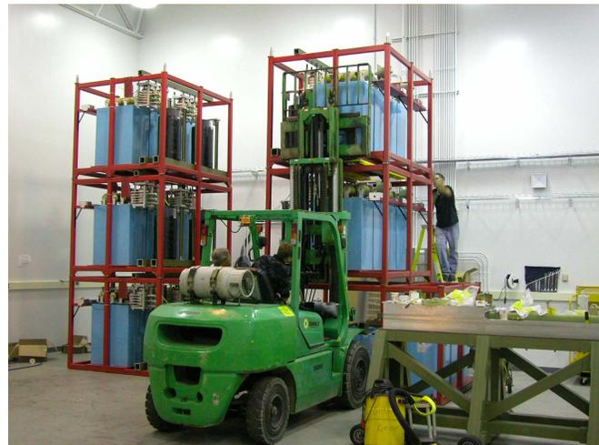
**Figure 4.** Forklift stack top level of bank frames.
