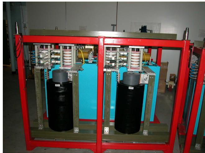
**Figure 3.** Two production banks mounted in their steel frame. The black object is the storage inductor, and the thyristor stack is to the left of the inductor, and the diode stack is to the right.
