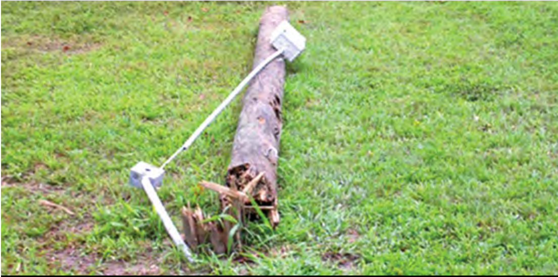
Figure 7. Fallen Pole in the AFRH-W Ponds Source: DoD IG–SPO
