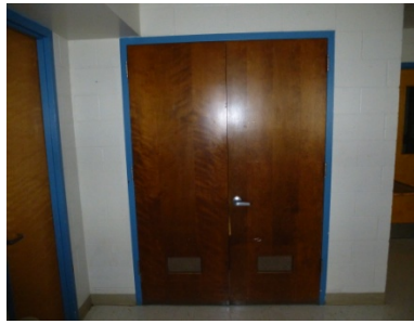
Original wood closet doors.
