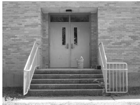
West elevation: 1984 addition drawing on the left compared to photo on right of the current replacement doors and original transom.
