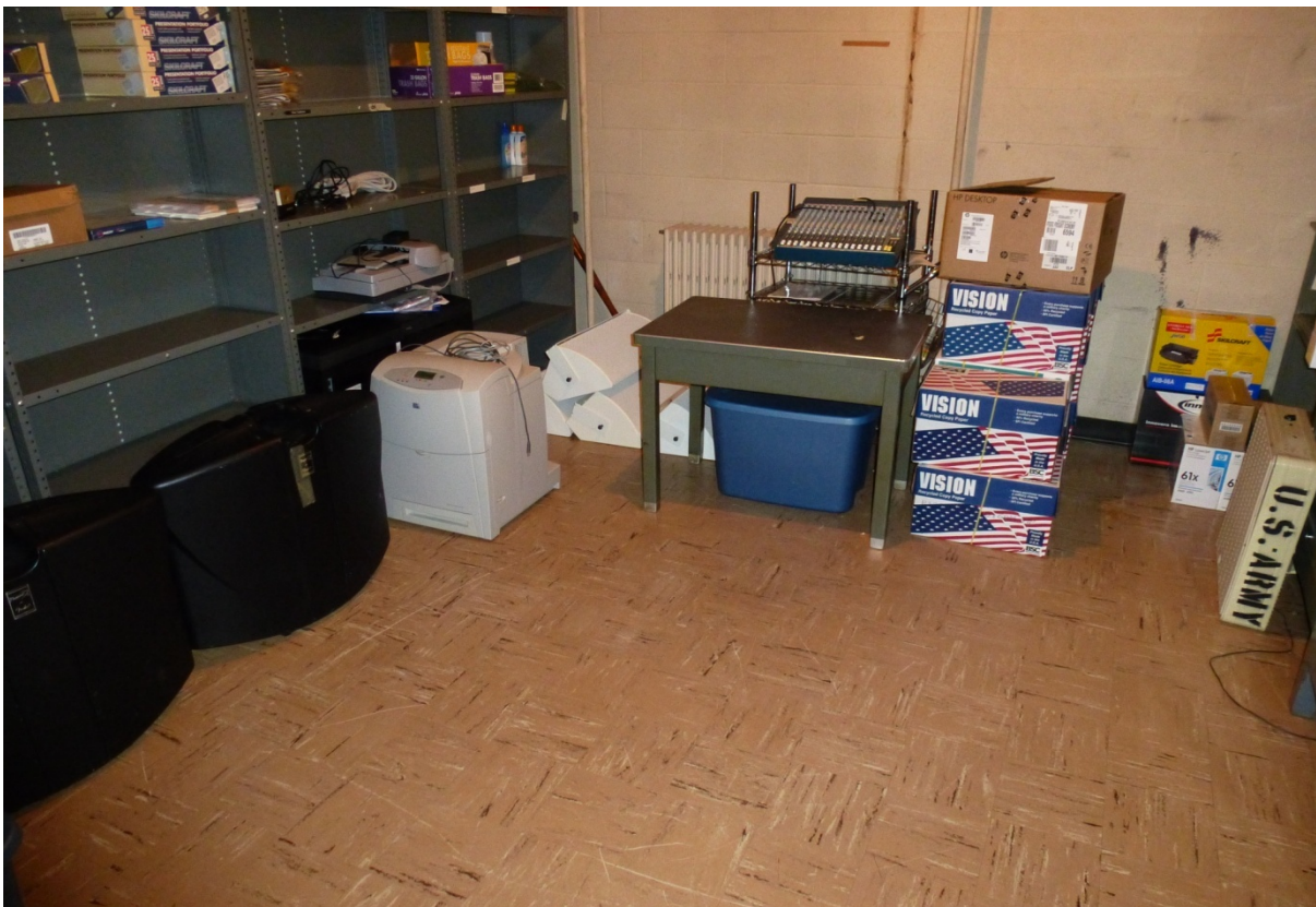
Photo 121. Storage room with original asbestos tile flooring (1957 addition) (ERDC-CERL, 2012).
