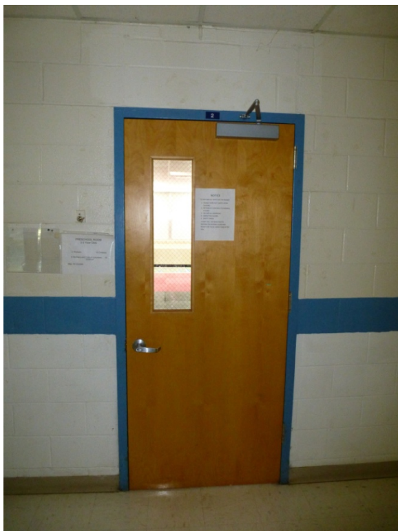
Photo 76. Replacement door into a kindergarten room (original school) (ERDC-CERL, 2012).
