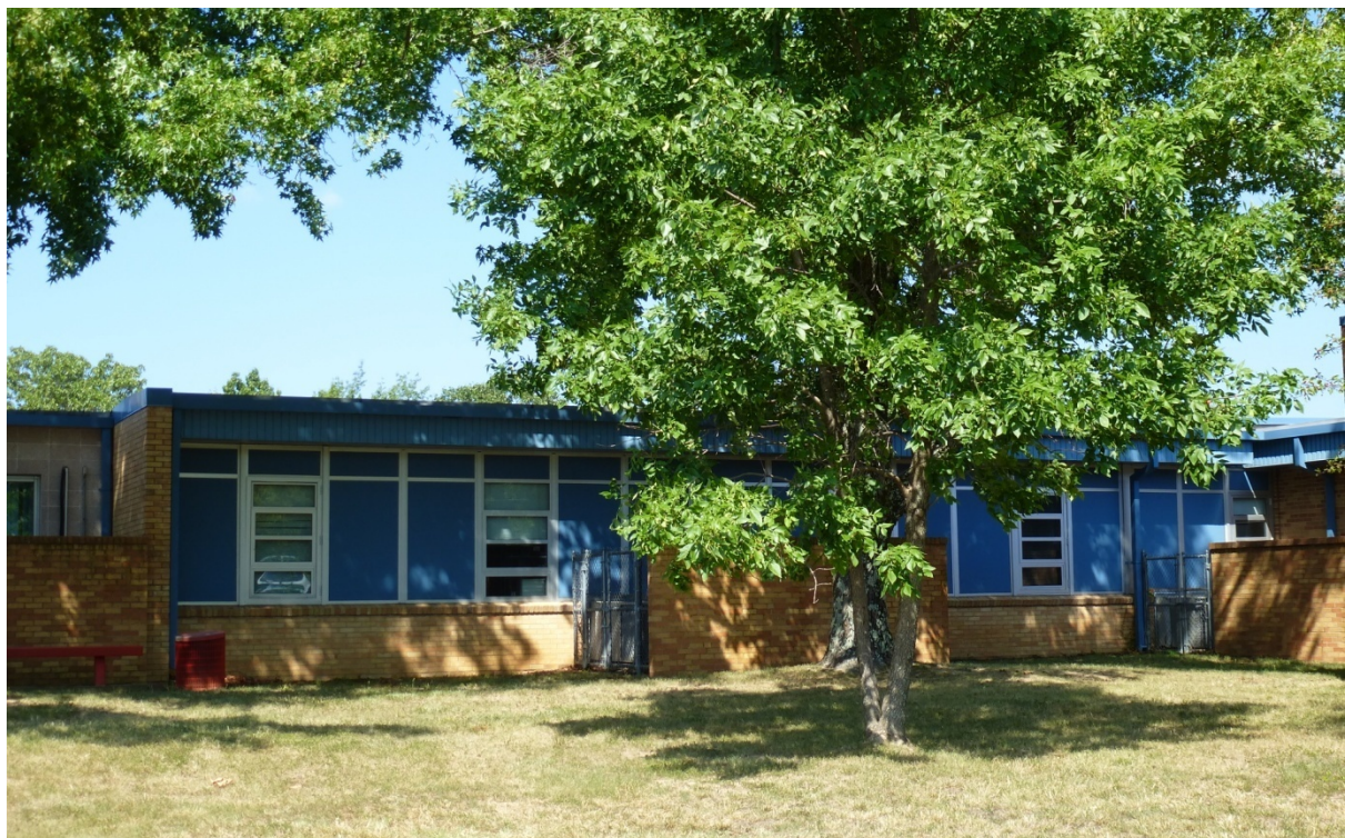
Photo 48. East elevation of the original school building with modified window pattern of replacement bright aluminum windows and panel inserts (ERDC-CERL, 2012).
