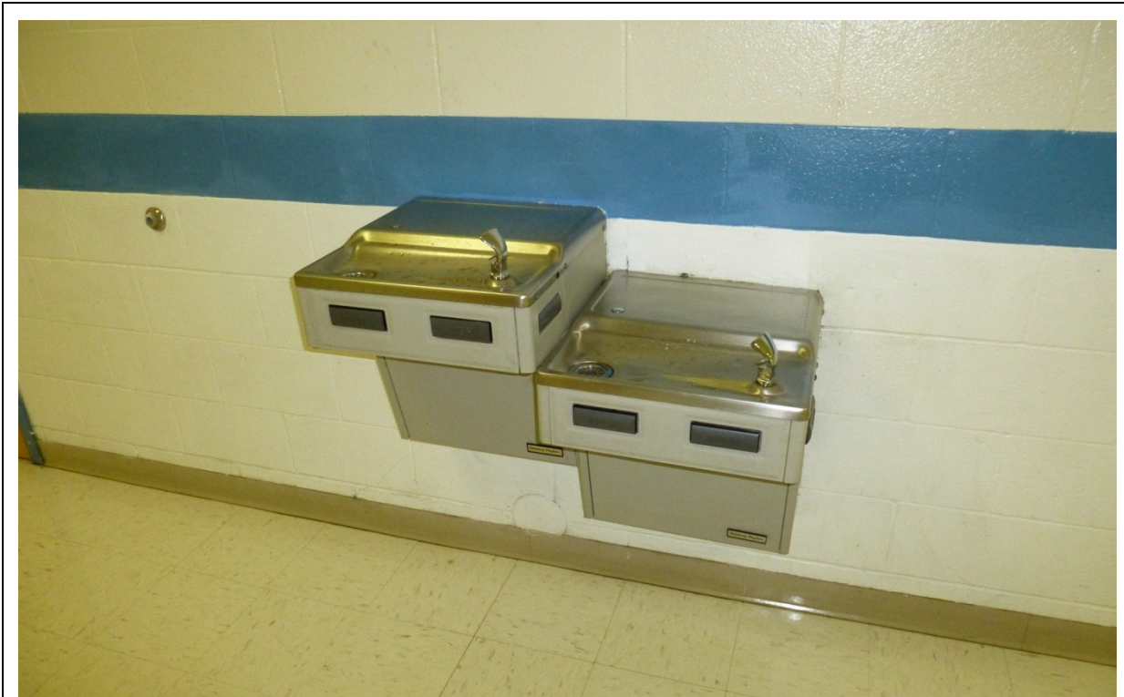
Photo 110. Water fountains in the corridor of 1957 addition (ERDC-CERL, 2012).
