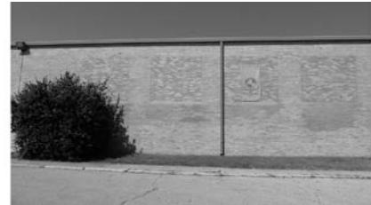
East elevation: Original drawing on the left from 1955 with original multi-pane windows located on the double-height wall of the all-purpose room compared to the current condition of the wall with the removal of the windows and infill brick.
