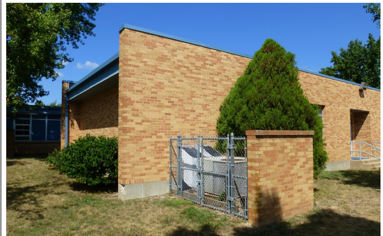
Photo 46. East elevation of 1984 addition (ERDC-CERL, 2012).
