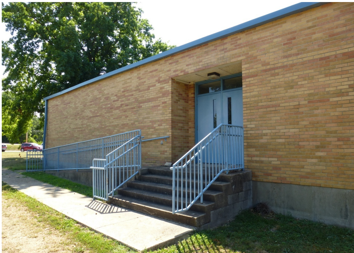
Photo 38. North elevation of 1957 addition with replacement entry doors (ERDC-CERL, 2012).
