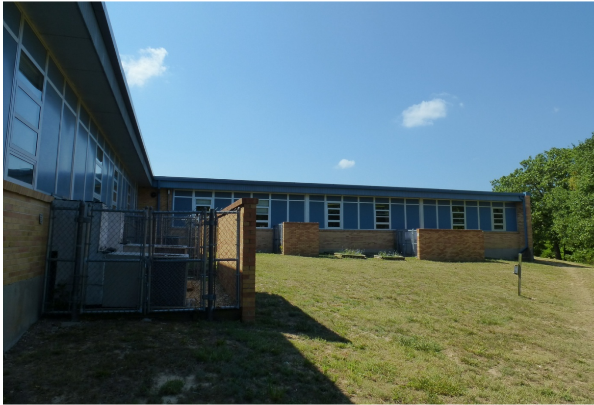
Photo 35. Right side of the north elevation with modified window pattern. Left side is 1957 addition and right side 1984 addition (ERDC-CERL, 2012).
