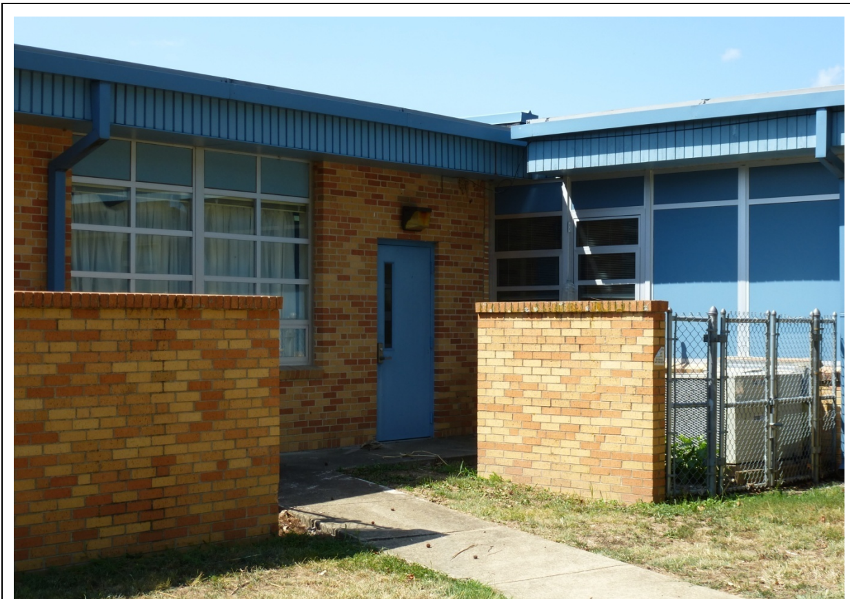
Photo 41. Closeup of connection between the 1957 addition (right side) and 1984 addition (left side) (ERDC-CERL, 2012).
