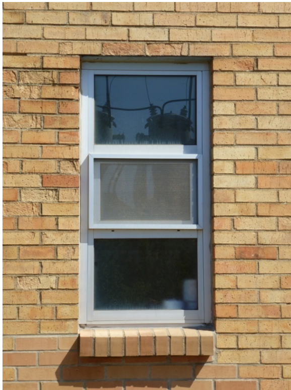
Photo 11. Closeup of replacement bright aluminum three-pane awning window (ERDC-CERL, 2012).
