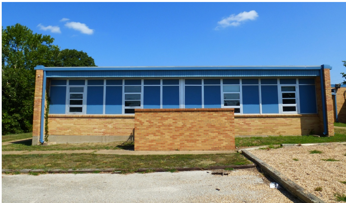
Photo 32. South elevation with modified window pattern with replacement windows and panel inserts. Left side is 1984 addition and right side is 1957 addition (ERDC-CERL, 2012).
