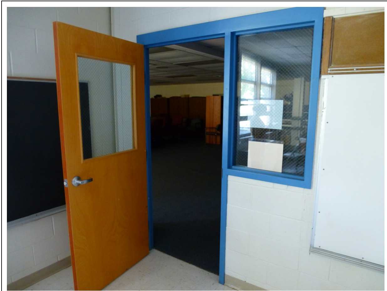
Photo 107. Door located in classroom, looking into media room (ERDC-CERL, 2012).
