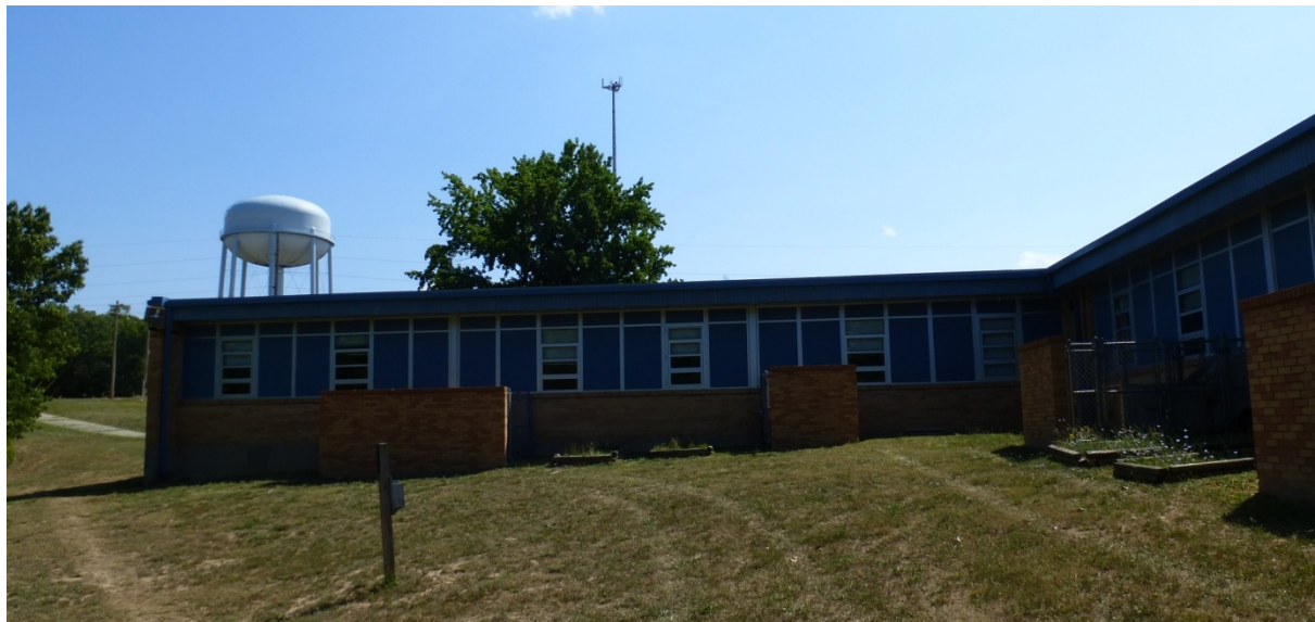
Photo 37. Left side of the west elevation of the 1957 addition with modified window pattern (ERDC-CERL, 2012).
