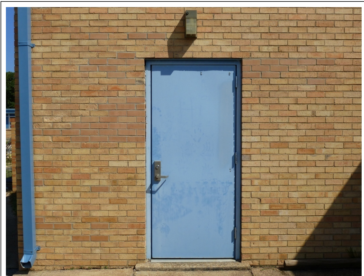
Photo 15. Replacement metal door on the far left side of the south elevation (ERDC-CERL, 2012).
