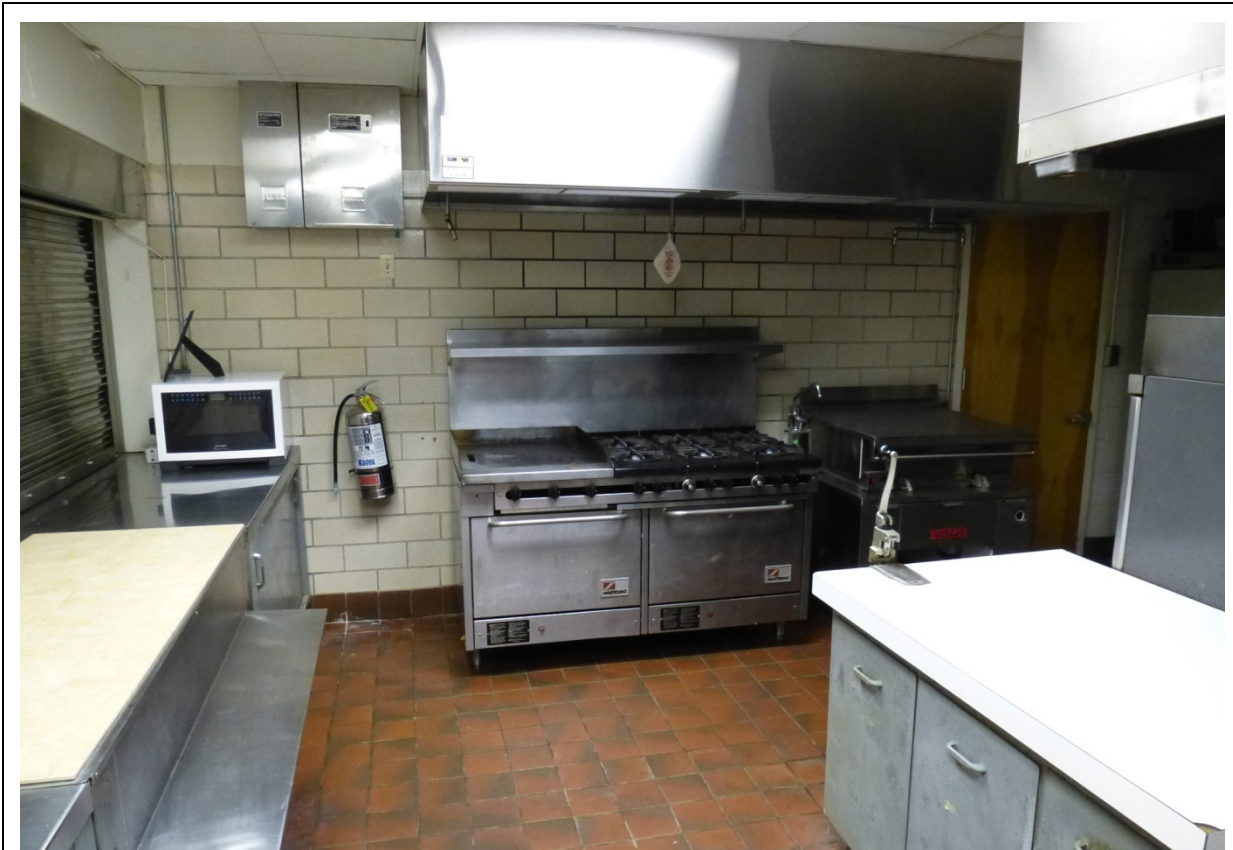
Photo 71. Kitchen with original glazed-tile floor and sanitary tile walls (original school) (ERDC-CERL, 2012).
