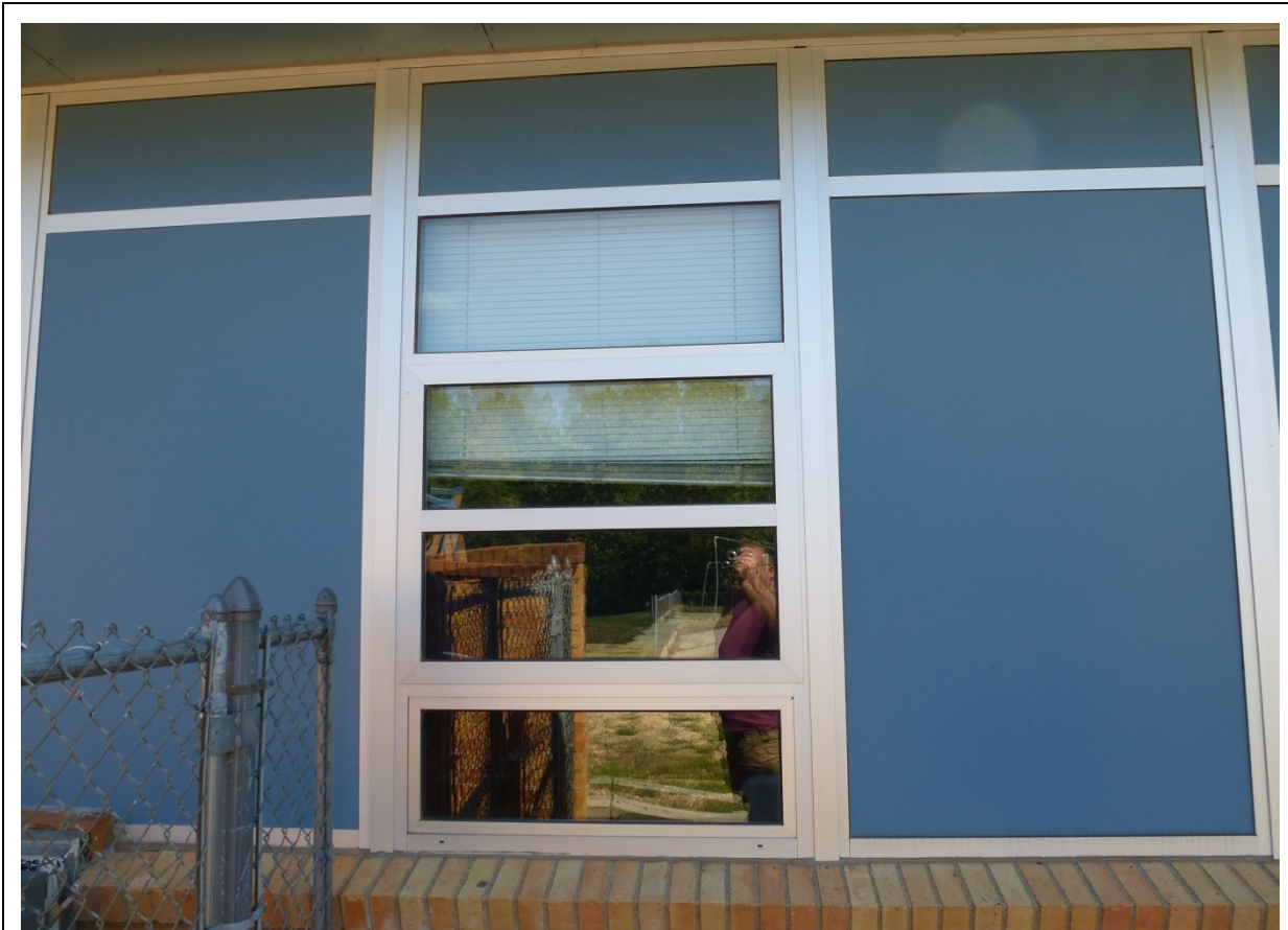
Photo 29. Close-up of replacement window and panel inserts (ERDC-CERL, 2012).
