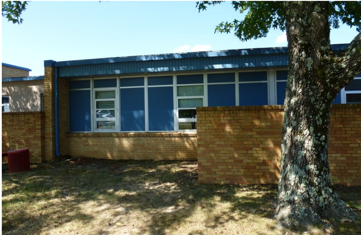
Photo 49. East elevation of the original school building with modified window pattern of replacement bright aluminum windows and panel inserts (ERDC-CERL, 2012).
