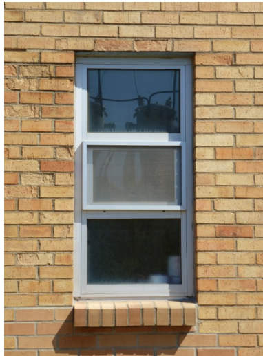
Replacement three-pane bright aluminum hopper window.
