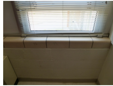
Original glazed-tile windowsill on the interior.
