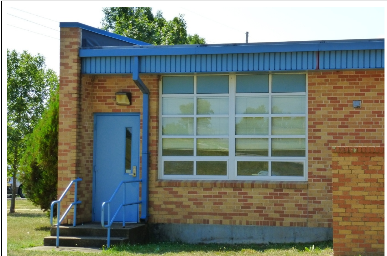
Photo 43. Left side of the north elevation of the 1984 addition with original windows and entry door (ERDC-CERL, 2012).
