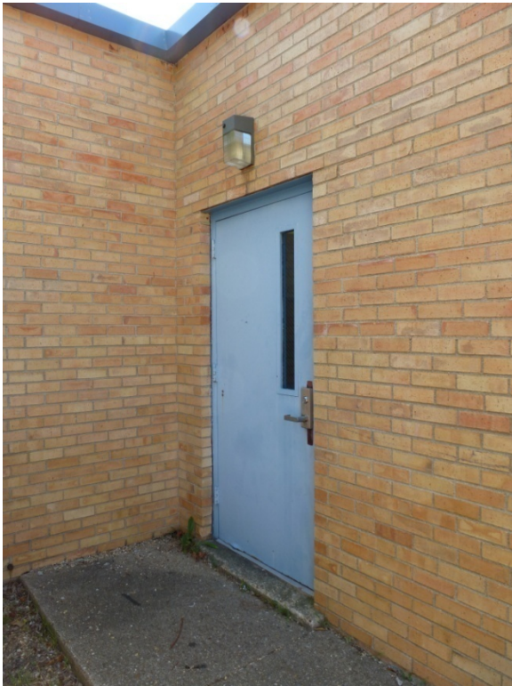
Photo 21. Replacement metal door and replacement light fixture on the west elevation (ERDC-CERL, 2012).
