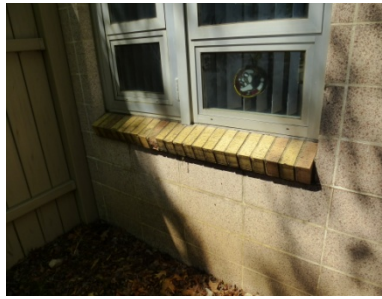
Original brick windowsill on exterior.
