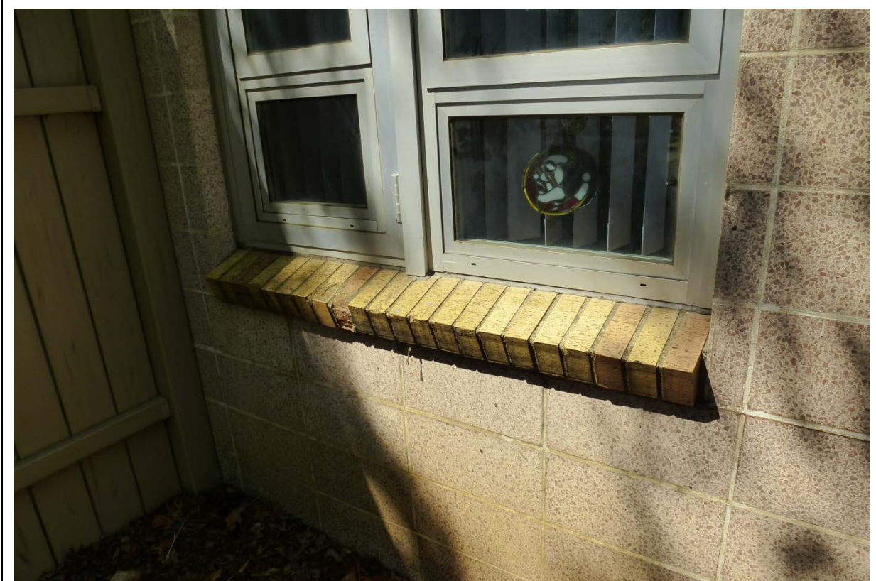
Photo 52. Replacement window with original brick windowsill near the main entry on the east elevation (ERDC-CERL, 2012).
