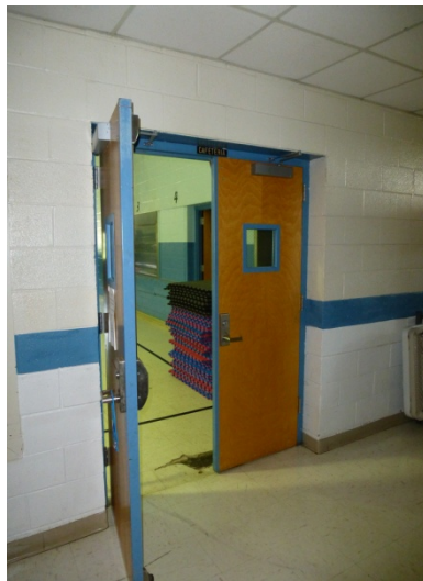
Replacement interior double door.
