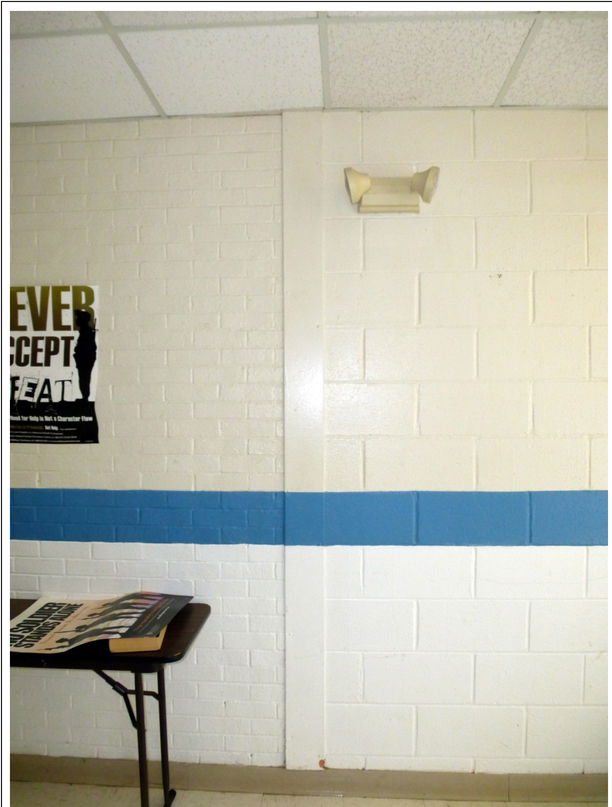
Photo 123. Closeup of the original north exterior wall of original school on left, connected to concrete block wall of the 1957 addition (ERDC-CERL, 2012).
