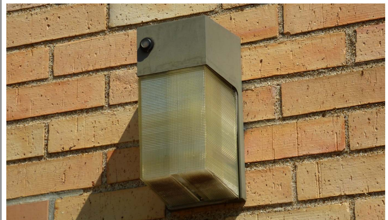
Photo 16. Replacement light fixture above the door on the far left side of the south elevation (ERDC-CERL, 2012).
