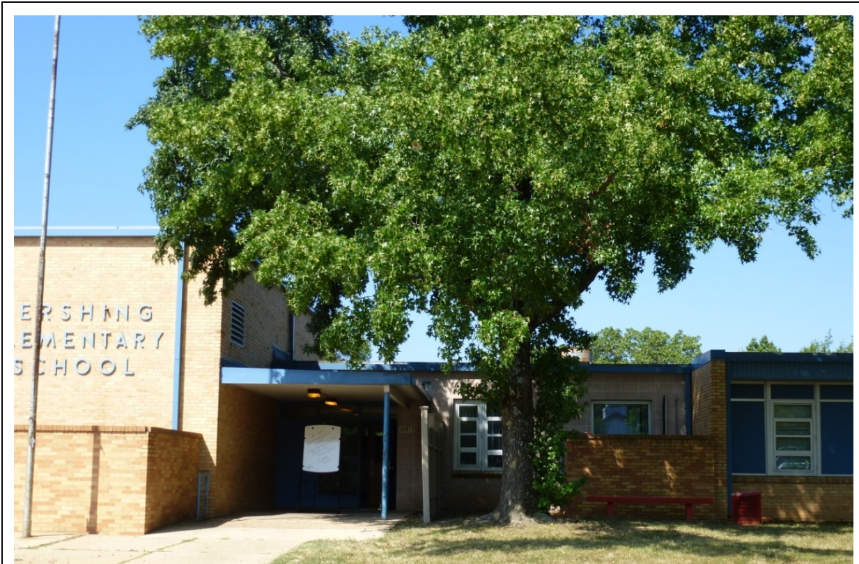
Photo 1. Main entrance on the east elevation (ERDC-CERL, 2012).
