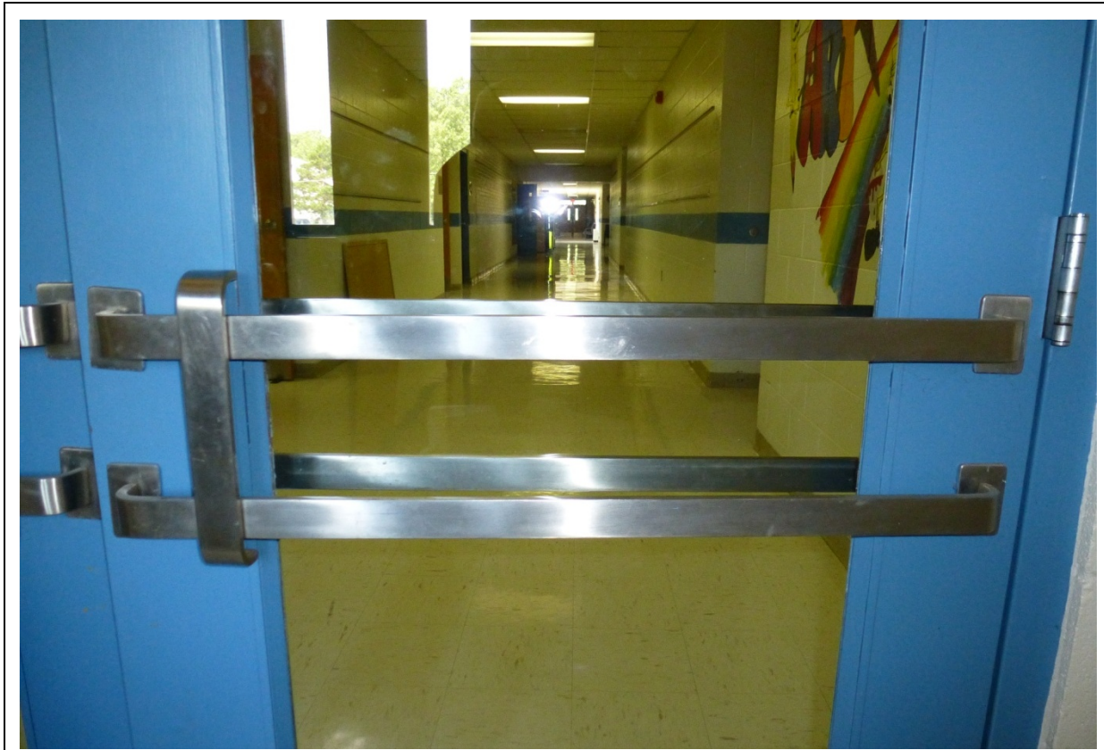
Photo 103. Closeup of older style vestibule door hardware (1984 addition) (ERDC-CERL, 2012).
