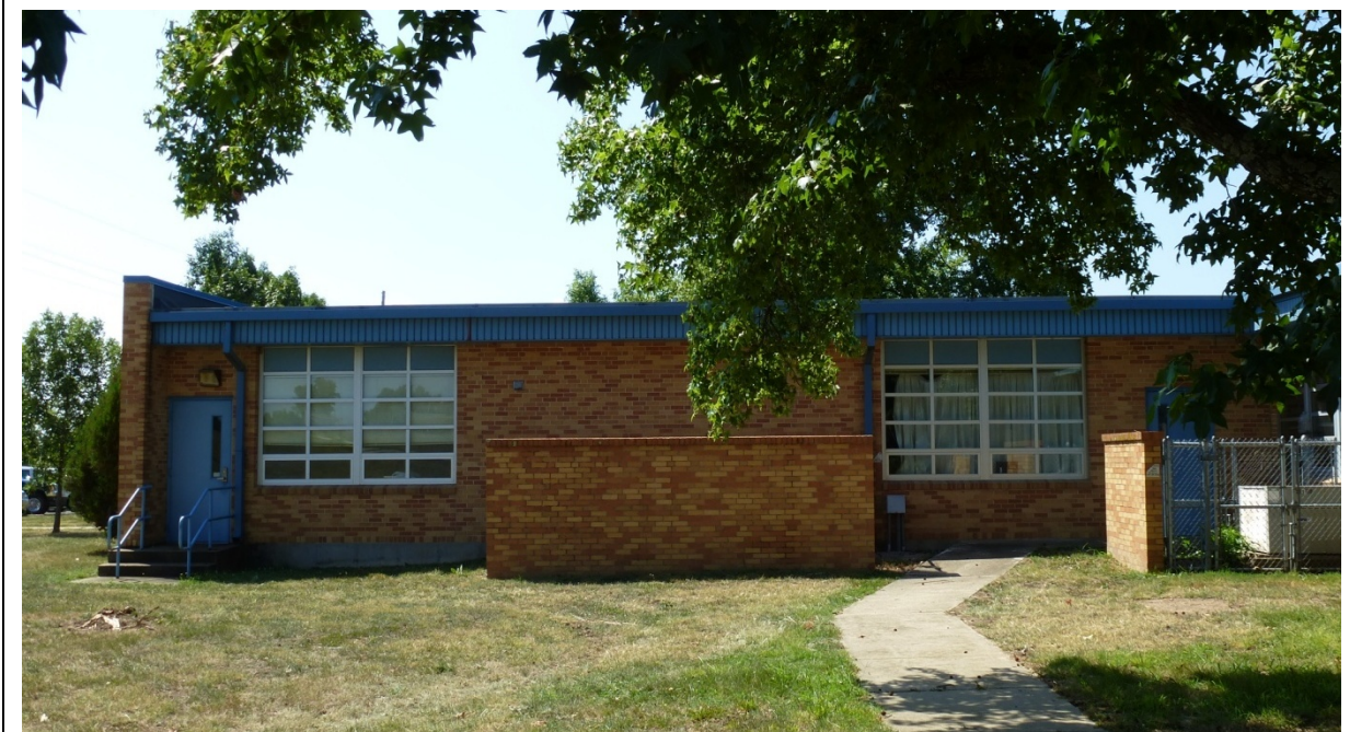
Photo 42. North elevation of 1984 addition (ERDC-CERL, 2012).
