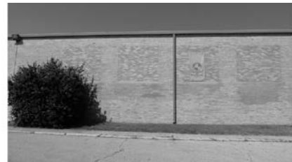
East elevation: Original drawing on the left from 1955 with original multi-pane windows located on the double-height wall of the all-purpose room compared to the current condition of the wall with the removal of the windows and use of infill brick.
