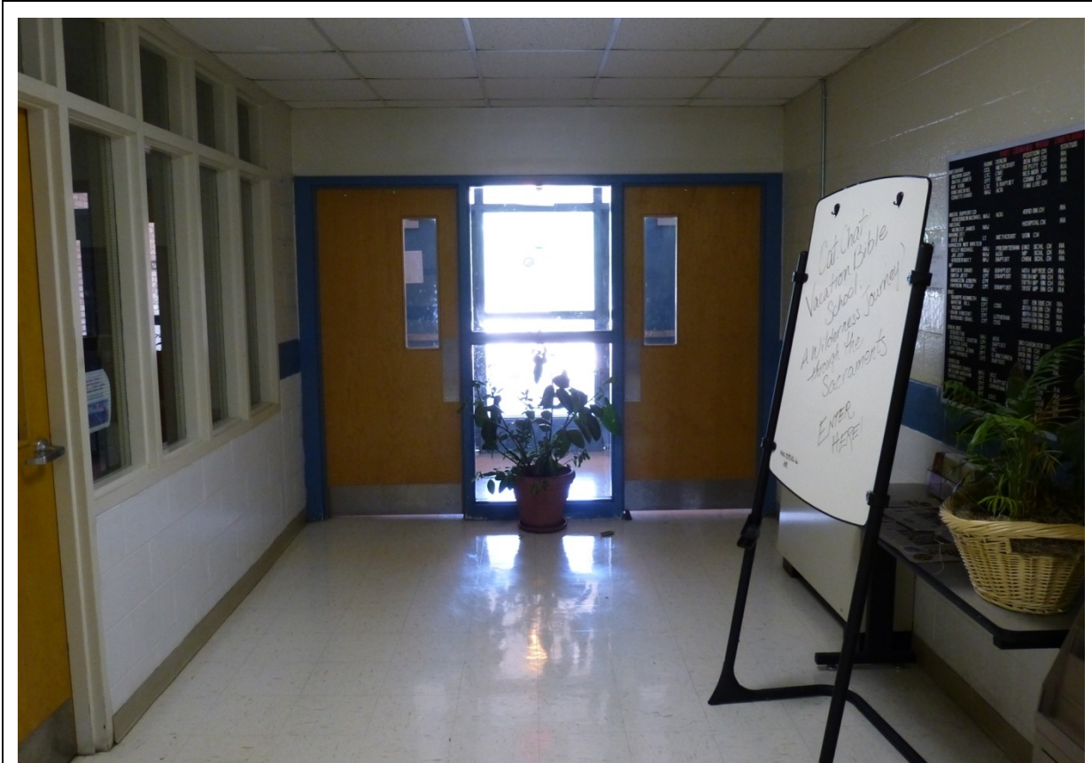
Photo 53. Looking toward the replacement vestibule doors on the east side of the building (original school) (ERDC-CERL, 2012).
