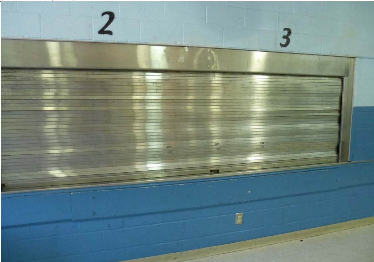
Photo 68. Modified serving line (original school) (ERDC-CERL, 2012).
