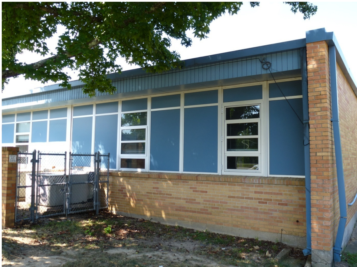
Photo 40. Closeup of bright aluminum replacement windows and panel inserts (ERDC-CERL, 2012).
