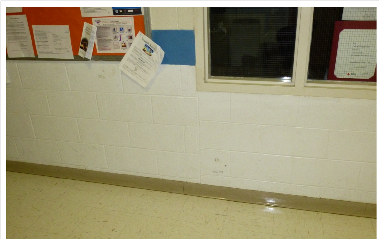
Photo 55. Closeup of the seam between original concrete block interior wall (left) and concrete block infill wall from 1984 remodel of office area (right) (ERDC-CERL, 2012).
