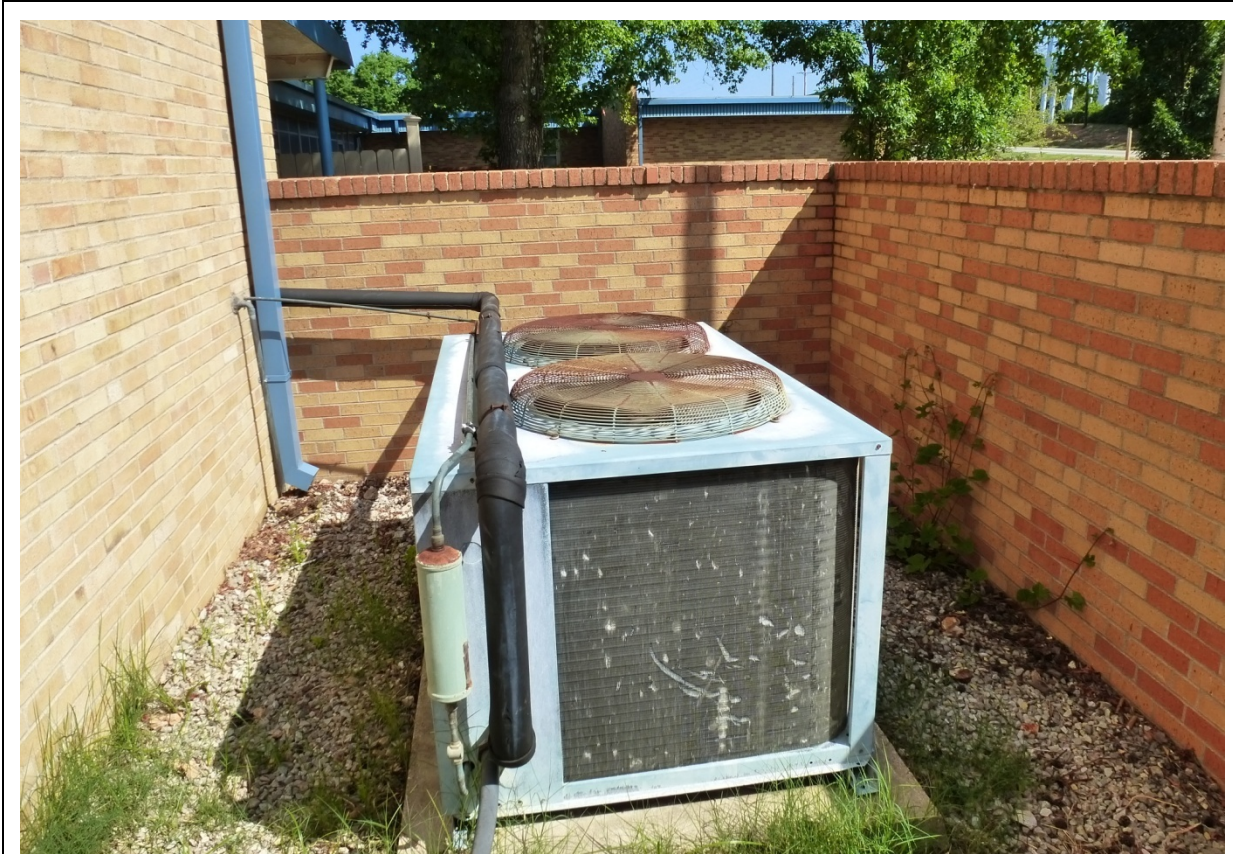
Photo 7. Air-conditioning unit addition with newer brick enclosure walls (ERDC-CERL, 2012).
