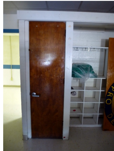
Original wood closet door.
