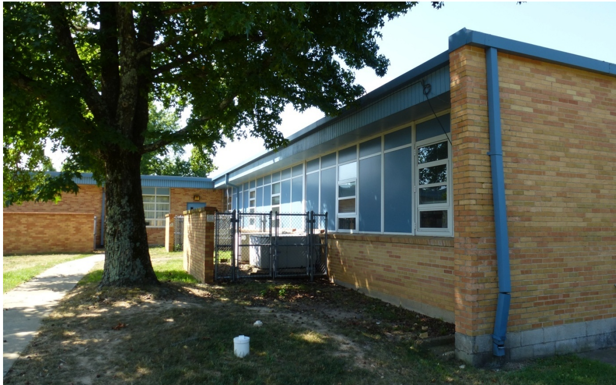
Photo 39. East elevation of 1957 addition with modified window pattern (ERDC-CERL, 2012).
