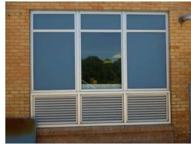
Replacement bright aluminum fixed window with porcelain enamel metal panels and metal louvered vents.
