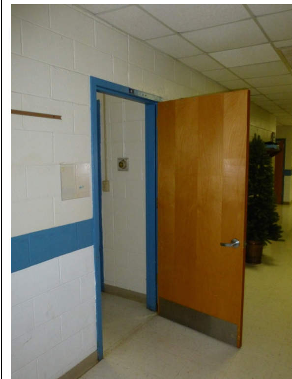
Photo 84. Replacement classroom door (original school) (ERDC-CERL, 2012).
