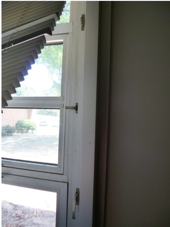
Photo 93. Closeup of replacement window hardware (original school) (ERDC-CERL, 2012).
