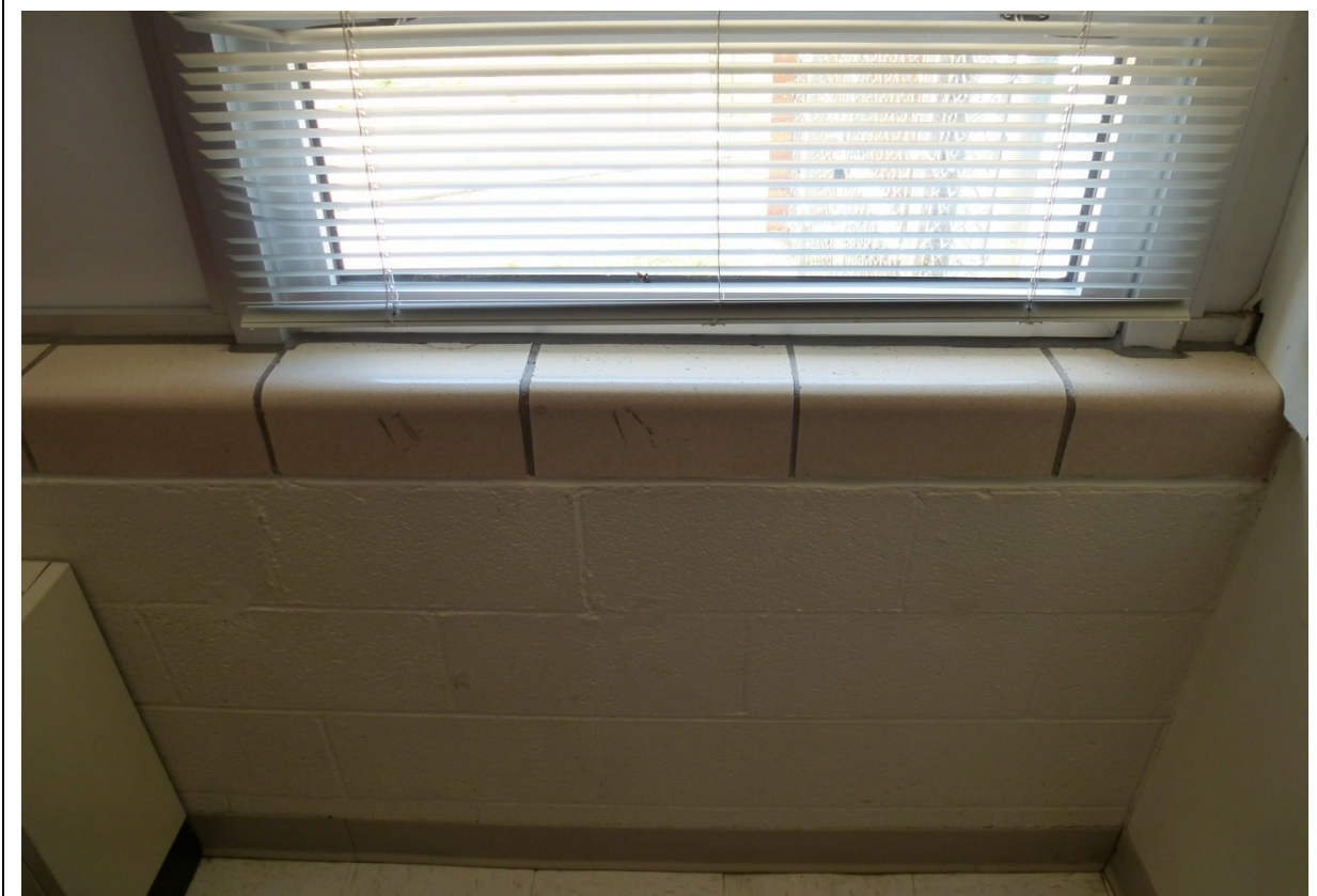
Photo 80. Original windowsill (original school) (ERDC-CERL, 2012).
