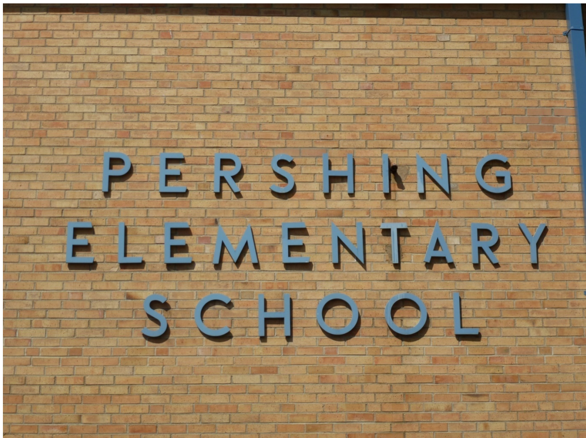
Photo 4. Original signage on the left side of the east elevation (ERDC-CERL, 2012).
