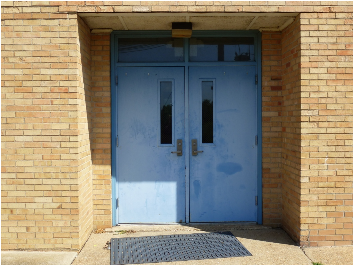
Photo 12. Closeup of replacement entry doors into the north-south corridor (ERDC-CERL, 2012).
