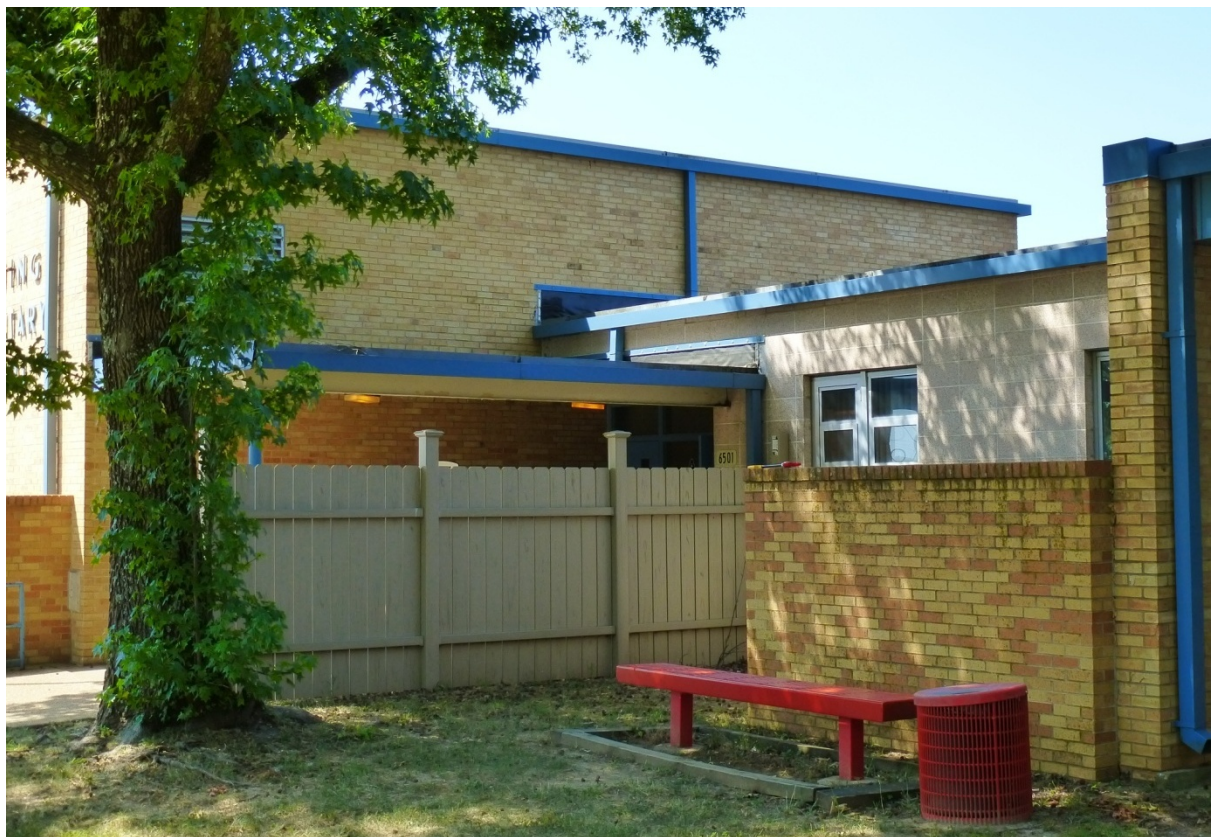
Photo 50. Looking toward the main entry on the east elevation (ERDC-CERL, 2012).
