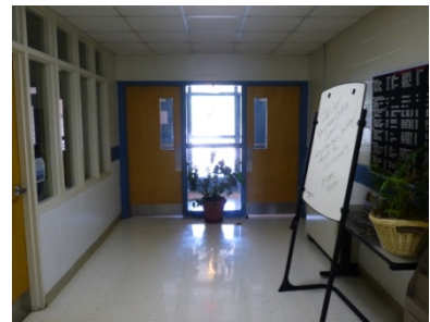
Replacement interior vestibule doors by main entry on east elevation.
