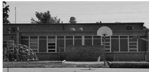
Right side of west elevation: Original 1955 drawing with design of classroom windows compared to the current condition of the elevation with replacement windows and metal panel inserts.
