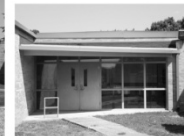
Window comparison: 1957 addition drawing on the left showing multi-pane awning/hopper steel sash windows compared to the current replacement bright aluminum and awning windows with porcelain enamel metal panel inserts. Also, the original doors have been replaced. The image on the right also shows the 1984 classroom addition on the far left.
