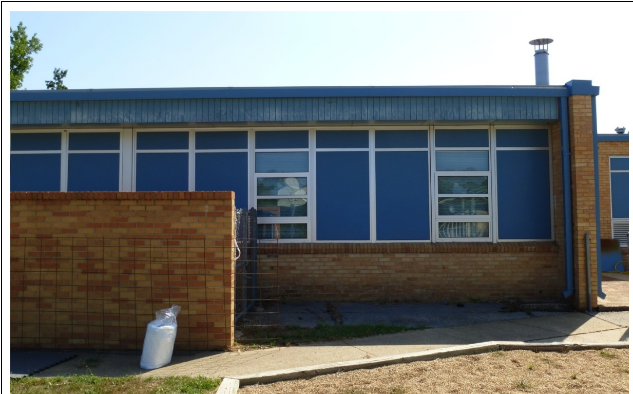
Photo 19. Closeup of replacement windows (ERDC-CERL, 2012).
