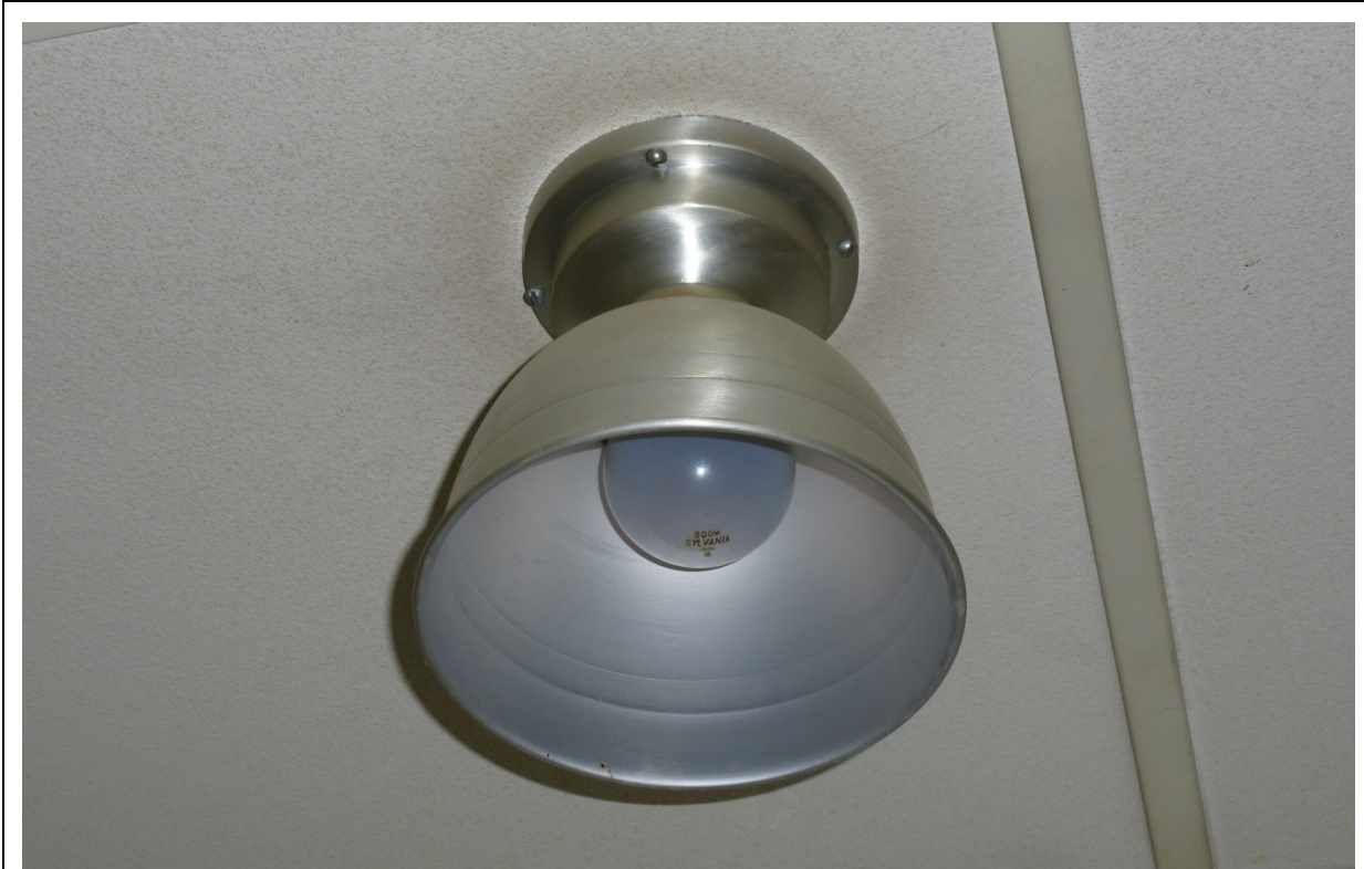
Photo 79. Older style light fixture in a kindergarten room (original school) (ERDC-CERL, 2012).
