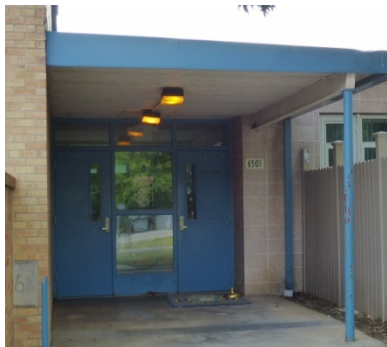
Replacement exterior main entry doors with sidelight.
