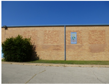
Removed original windows and openings filled with brick.
