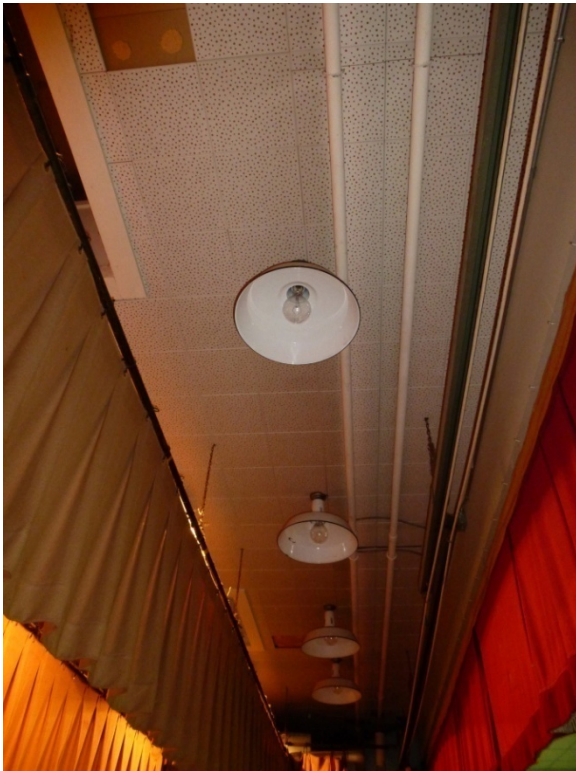
Photo 63. Original light fixtures above stage (original school) (ERDC-CERL, 2012).
