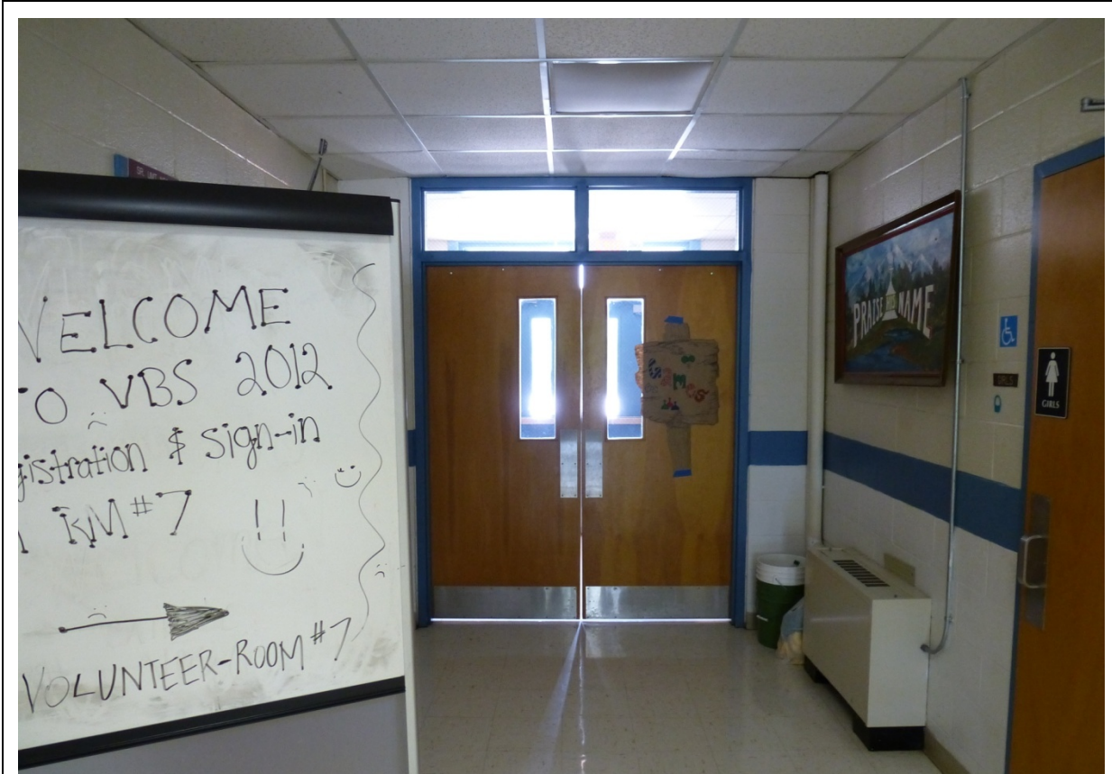
Photo 57. Looking toward replacement vestibule doors on the west side of the building (original school) (ERDC-CERL, 2012).
