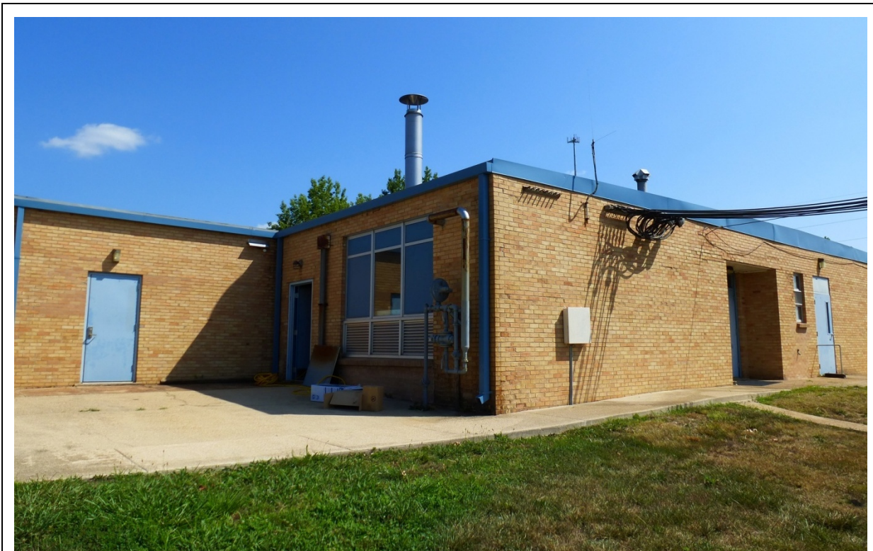
Photo 13. Looking at the exterior of the boiler room on the south elevation (ERDC-CERL, 2012).
