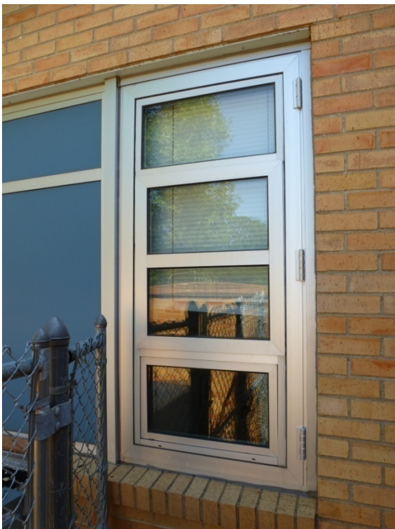
Photo 22. Closeup of replacement bright aluminum egress window (ERDC-CERL, 2012).
