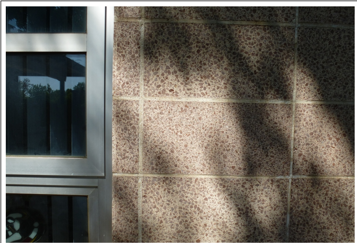
Photo 51. Original terrazzo faced block near the main entry on the east elevation (ERDC-CERL, 2012).
