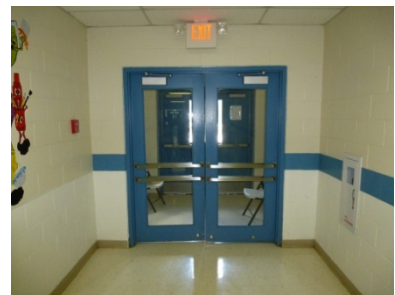
Replacement interior double door (1950s metal doors with original hardware).
