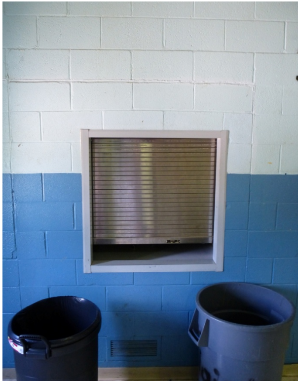
Photo 67. Original door opening filled in with concrete block and small window opening (original school) (ERDC-CERL, 2012).
