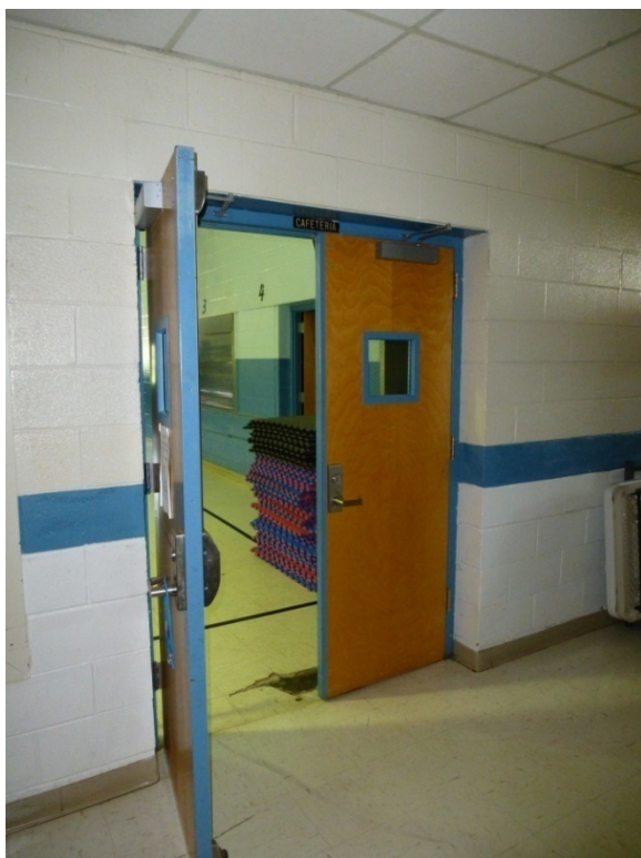
Photo 60. Replacement wood doors into the multi-purpose room (original school) (ERDC-CERL, 2012).
