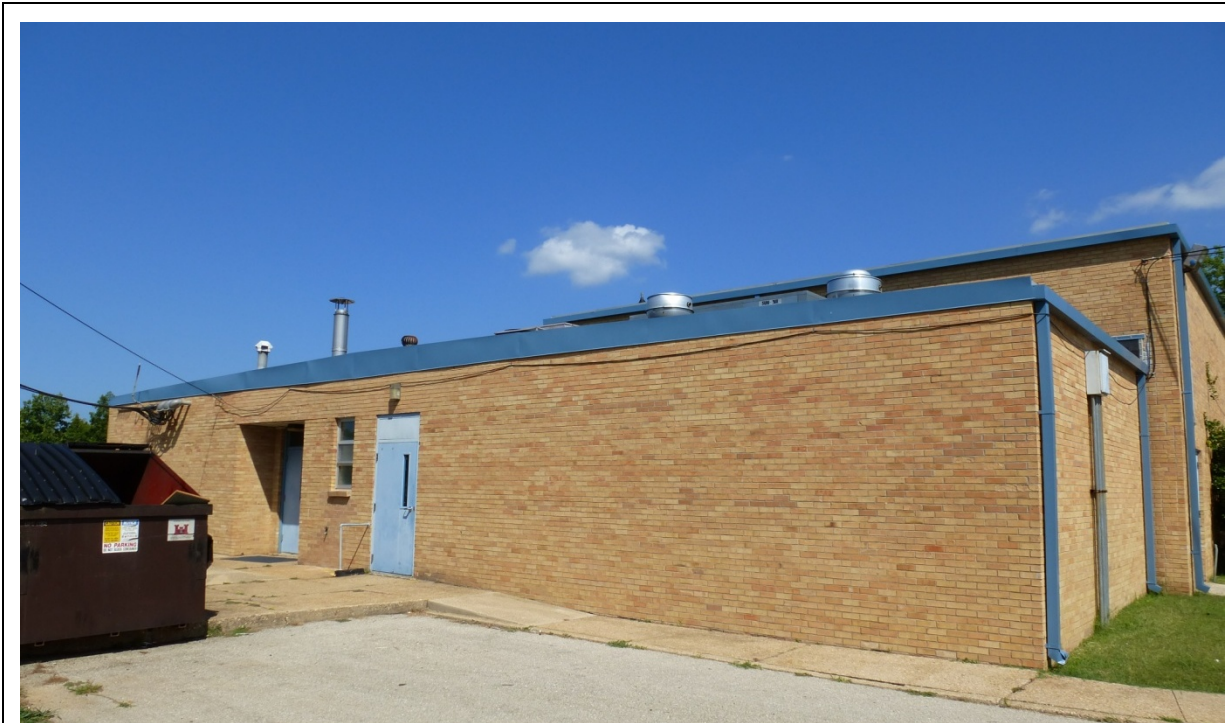
Photo 9. Southeast corner of original school (ERDC-CERL, 2012).
