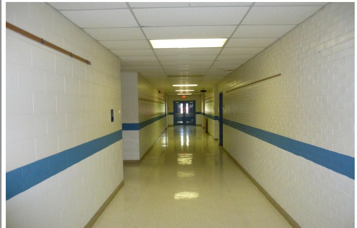
Photo 100. Looking north down corridor of 1984 addition (ERDC-CERL, 2012).
