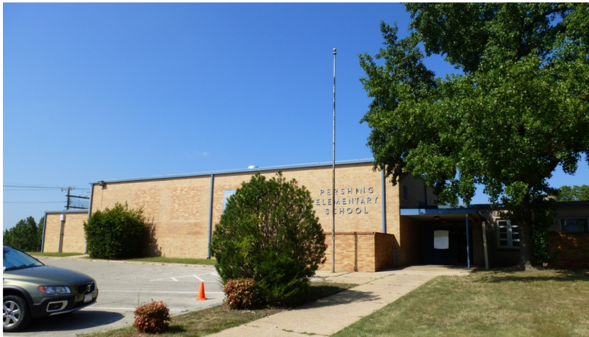
Photo 3. Left side of the east elevation (ERDC-CERL, 2012).
