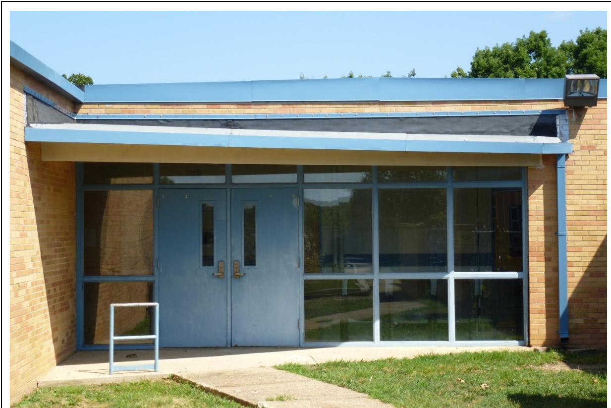
Photo 31. Entry on the south side of the 1957 addition. The windows and angled canopy structure are original to the 1957 design and construction, while the entry doors are replacement (ERDC-CERL, 2012).
