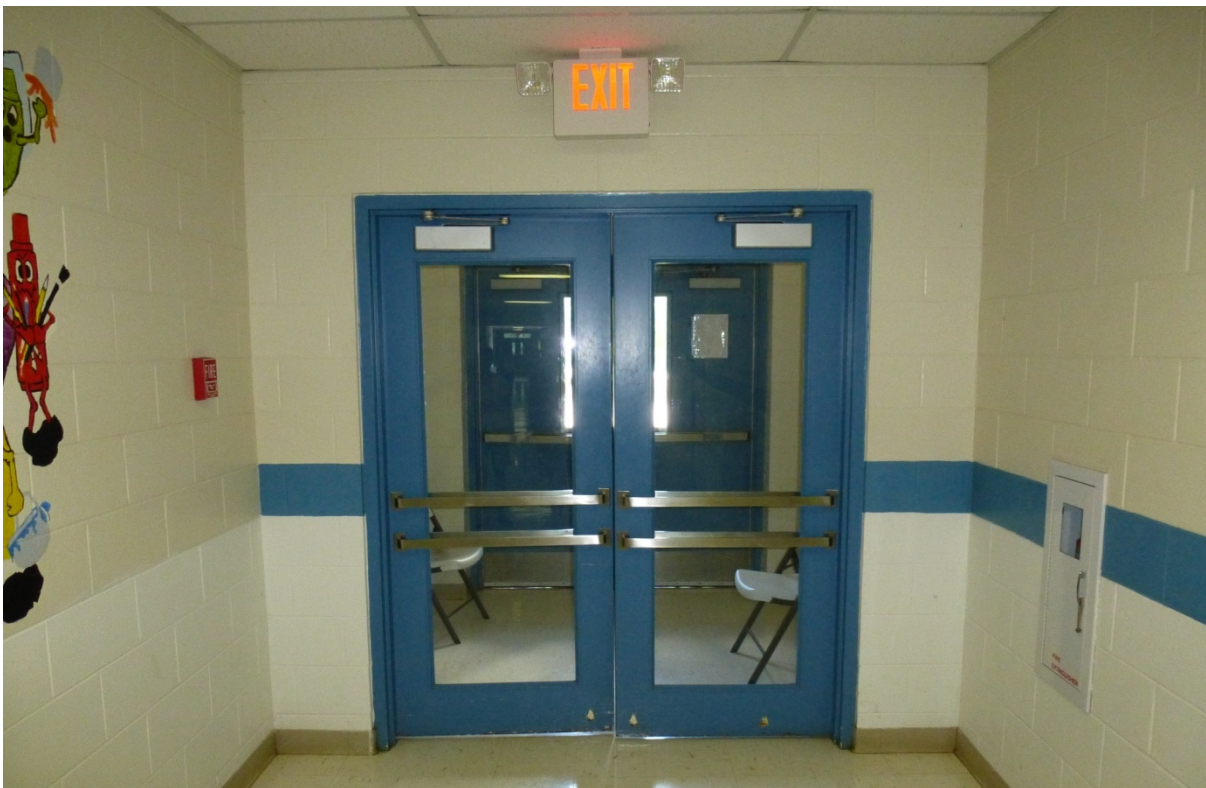
Photo 102. Older style vestibule doors located on the east end of the 1984 addition corridor (ERDC-CERL, 2012).
