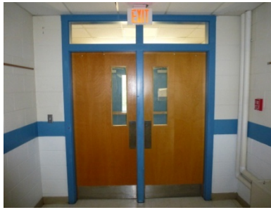
Replacement interior vestibule doors.
