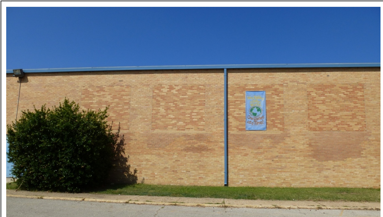
Photo 5. Modified window openings on the left side of the east elevation (ERDC-CERL, 2012).
