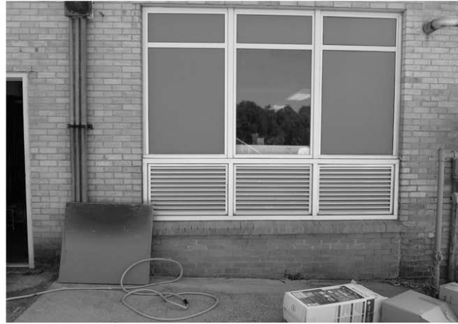
Window comparison: Original drawing on the left from 1955 showing two original multi-pane awning steel sash windows with two metal louvered vents compared to the current replacement bright aluminum and awning windows with porcelain enamel metal panel inserts and new metal louvered vents.
