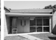
Window comparison: 1957 addition drawing on the left showing multi-pane awning/hopper steel sash windows compared to the current replacement bright aluminum and awning windows with porcelain enamel metal panel inserts. Also, the original doors have been replaced. The image on the right also shows the 1984 classroom addition.
