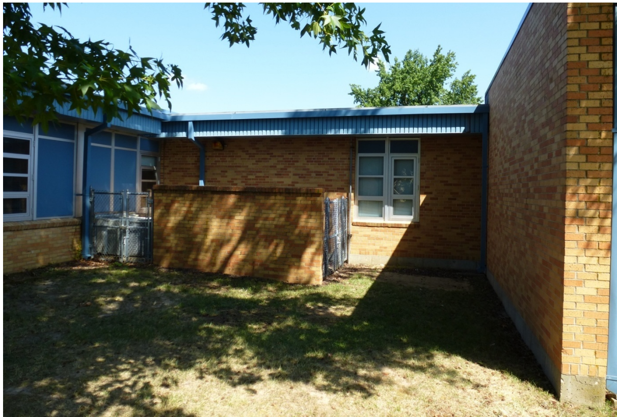
Photo 47. South elevation of the 1984 addition (ERDC-CERL, 2012).
