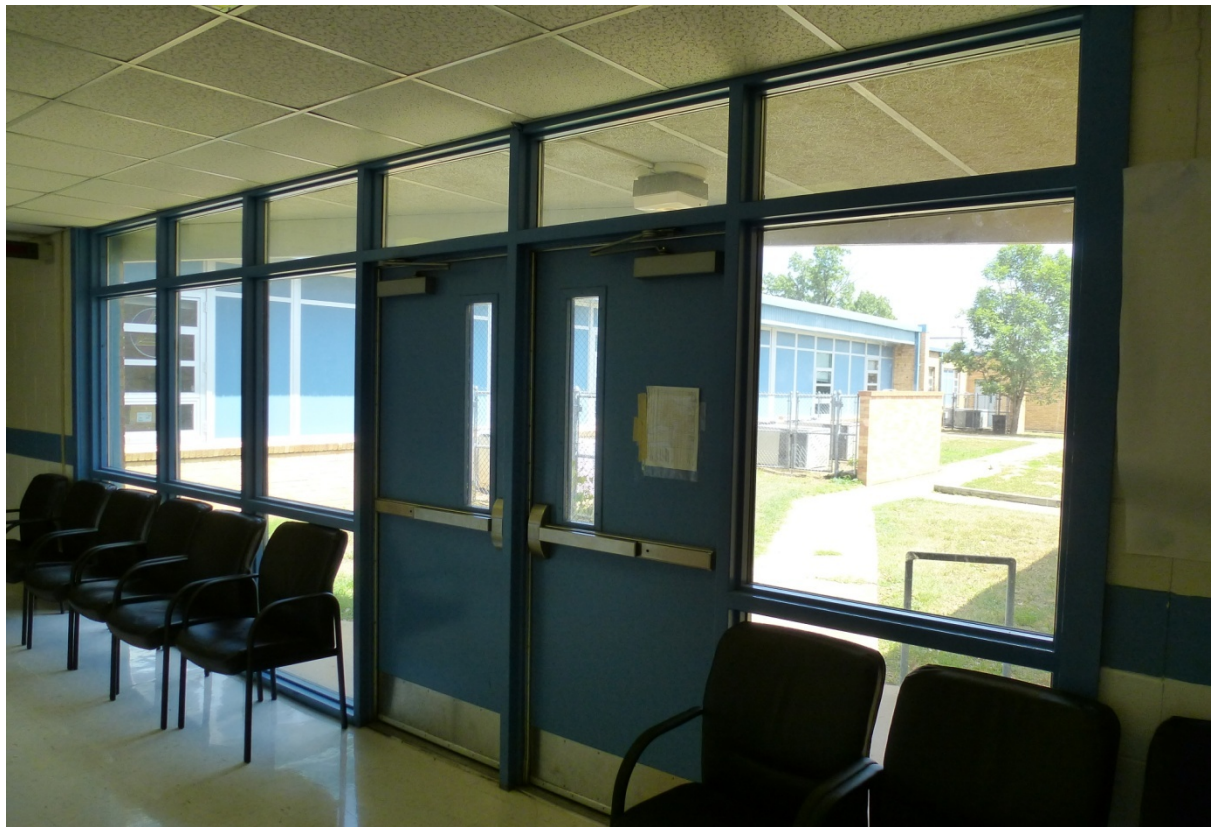
Photo 124. Original 1957 curtain wall with replacement entry doors on the south side of the 1957 west wing addition (ERDC-CERL, 2012).
