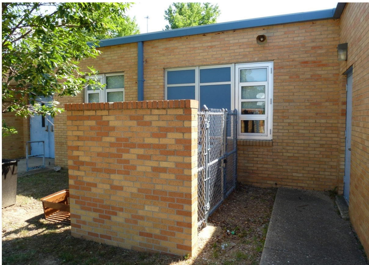
Photo 20. Replacement windows and air conditioning unit addition on the west elevation of the original school (ERDC-CERL, 2012).
