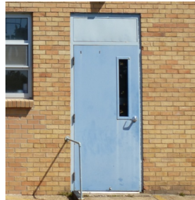
Replacement exterior metal door with narrow pane.
