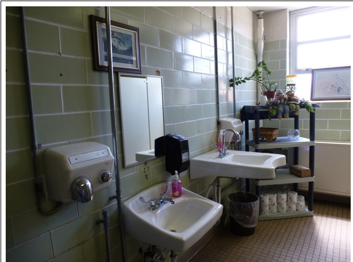
Photo 87. Girls' restroom with replacement sinks (original school) (ERDC-CERL, 2012).
