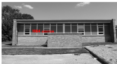
Window comparison: 1957 addition drawing on the left showing multi-pane awning/hopper steel sash windows compared to the current replacement bright aluminum and awning windows with porcelain enamel metal panel inserts. Also, the original doors have been replaced. The image on the right also shows the 1984 classroom addition.
