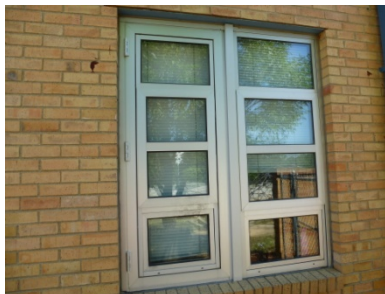
Replacement paired bright aluminum awning windows.
