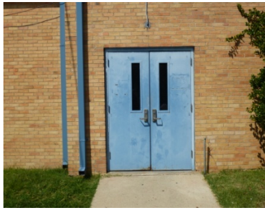
Replacement exterior doors.
