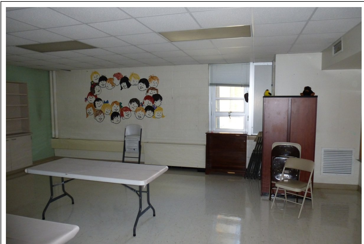
Photo 97. Classroom with replacement windows, floor, and ceiling (original school) (ERDC-CERL, 2012).
