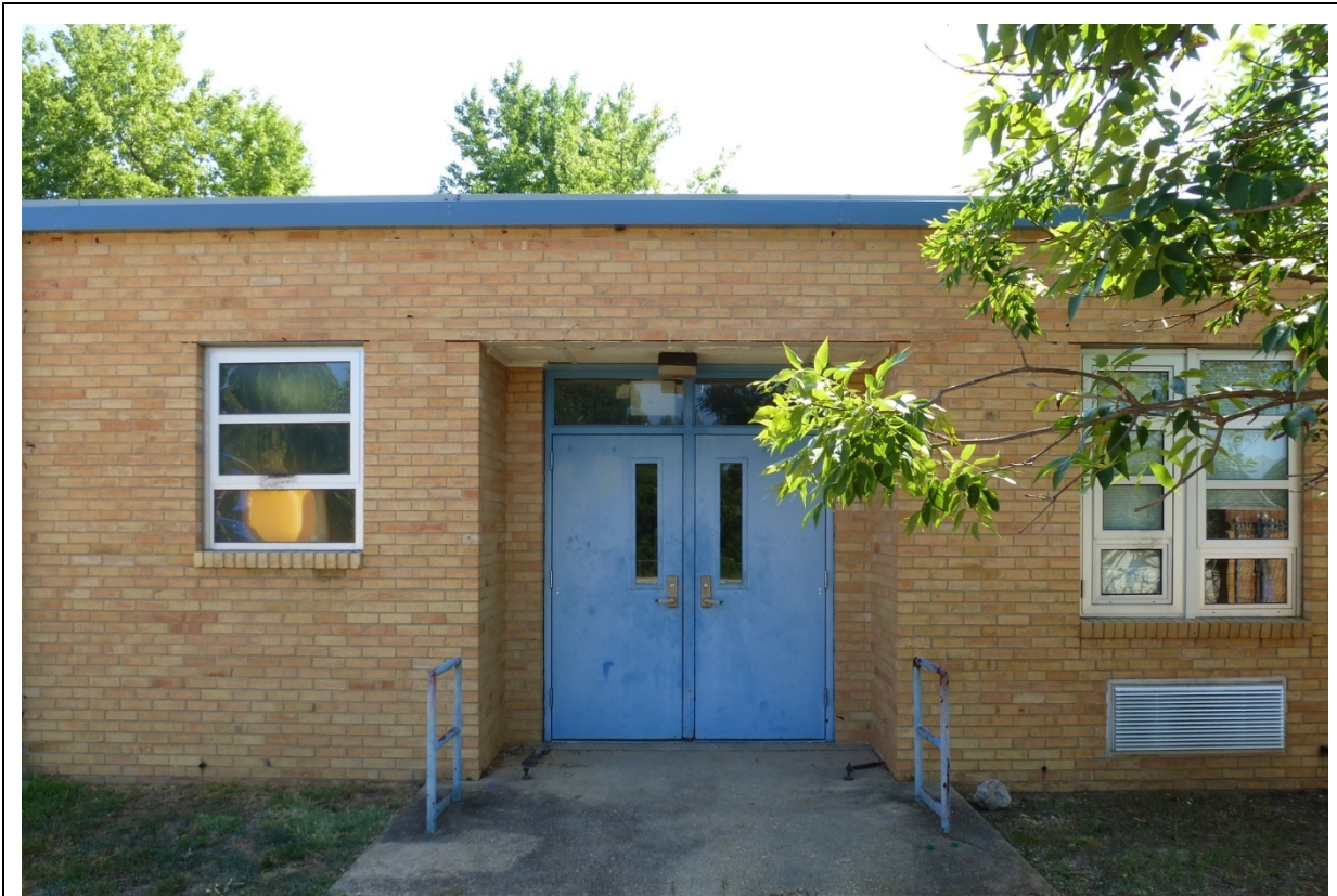
Photo 23. Replacement metal entry doors leading into the east-west corridor of the original school (ERDC-CERL, 2012).
