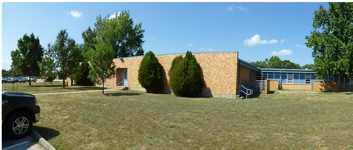
Photo 44. East elevation (left side is 1984 addition while the right side is the 1957 addition) (ERDC-CERL, 2012).
