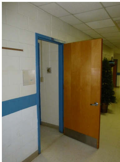
Replacement interior wood door.
