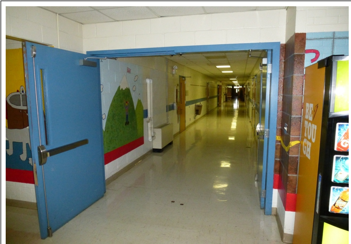
Photo 99. Intersection of corridors where 1957 addition is connected to the original school. Looking south down original corridor (ERDC-CERL, 2012).
