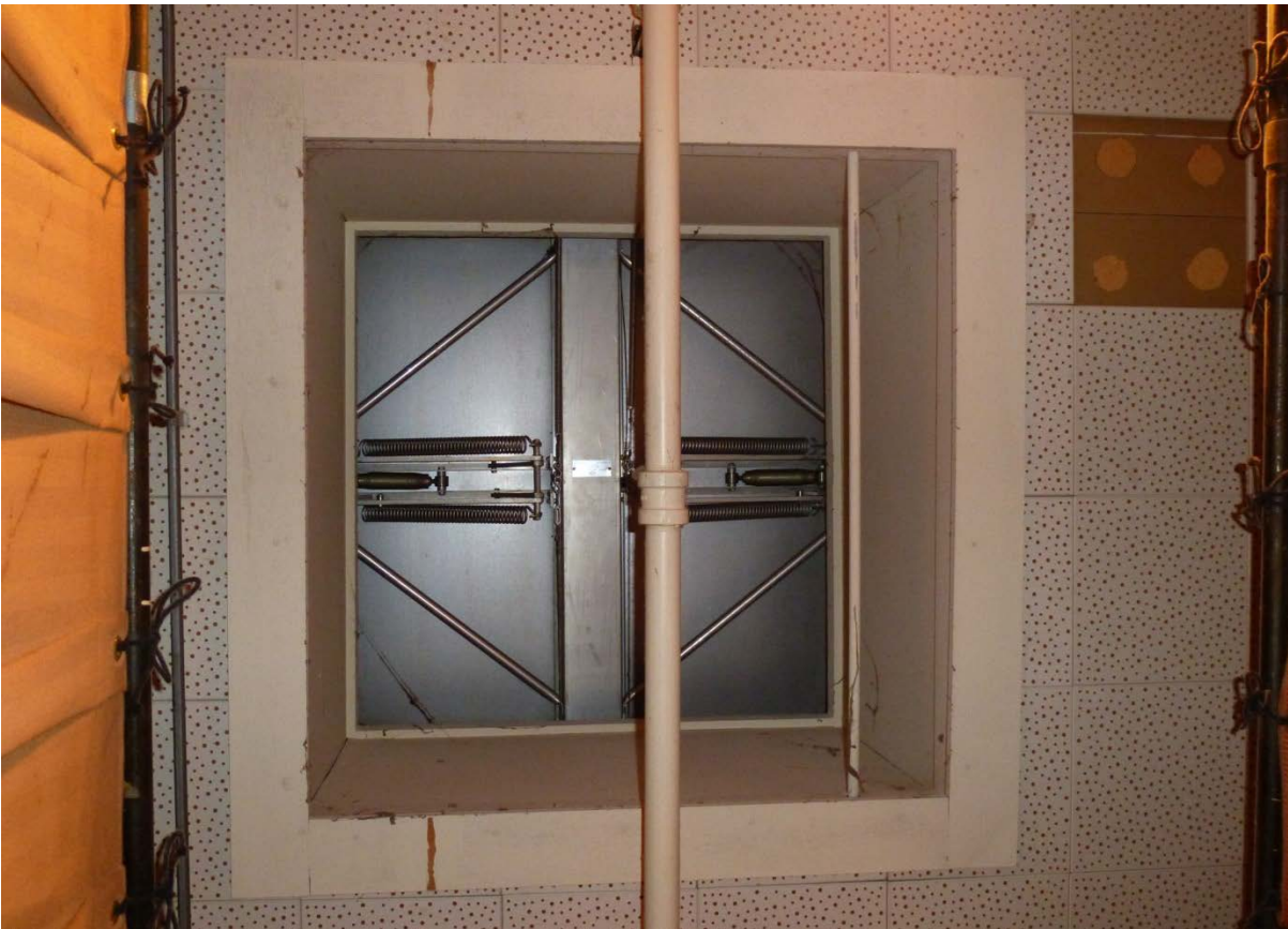
Photo 64. Looking up at original light dome located above the stage (original school) (ERDC-CERL, 2012).
