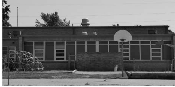
Right side of west elevation: Original 1955 drawing with design of classroom windows compared to the current condition of the elevation with replacement windows and metal panel inserts.
