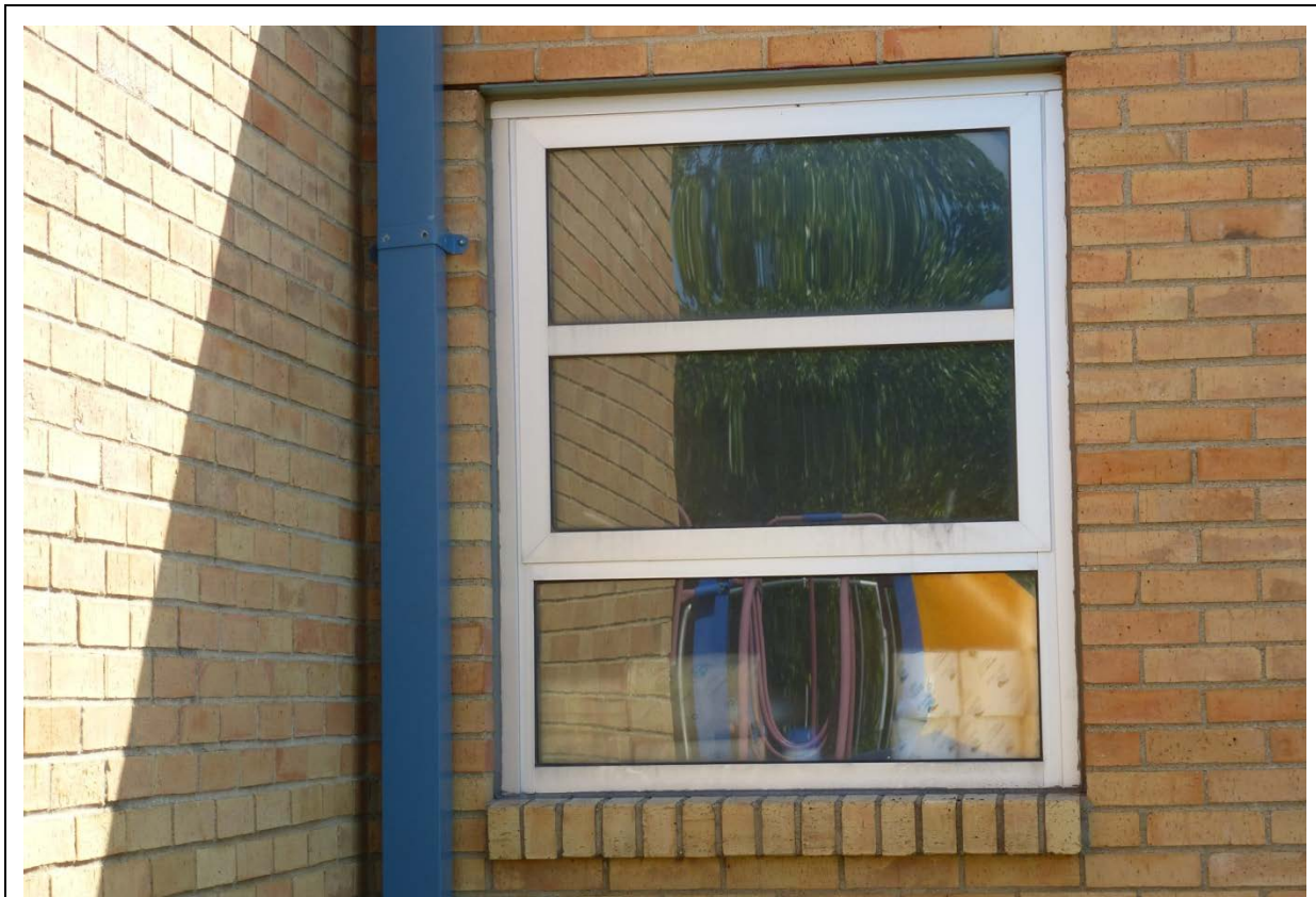
Photo 26. Replacement bright aluminum three-pane awning window (ERDC-CERL, 2012).
