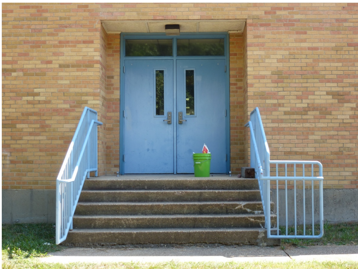
Photo 34. Replacement entry doors on the west elevation of 1984 addition with original metal handrails (ERDC-CERL, 2012).
