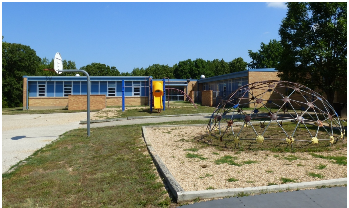
Photo 27. Looking north toward both the 1957 (left) and 1984 (right) additions (ERDC-CERL, 2012).
