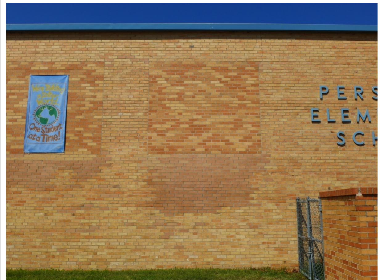
Photo 6. Closeup of the modified window openings on the left side of the east elevation (ERDC-CERL, 2012).
