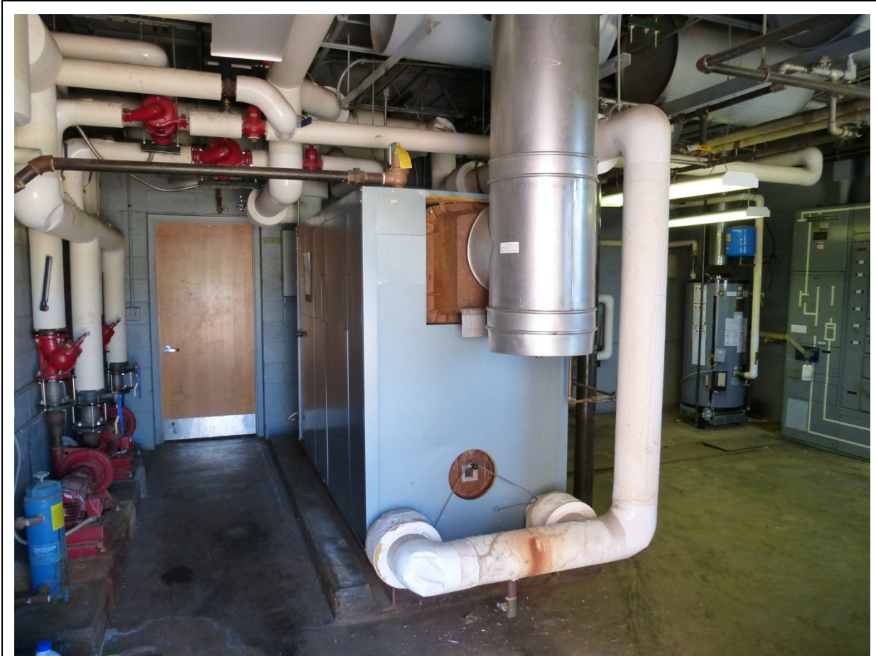
Photo 75. Boiler room (original school) (ERDC-CERL, 2012).
