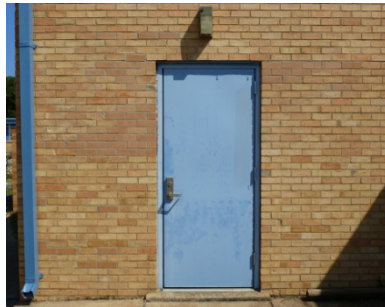
Replacement exterior metal door.
