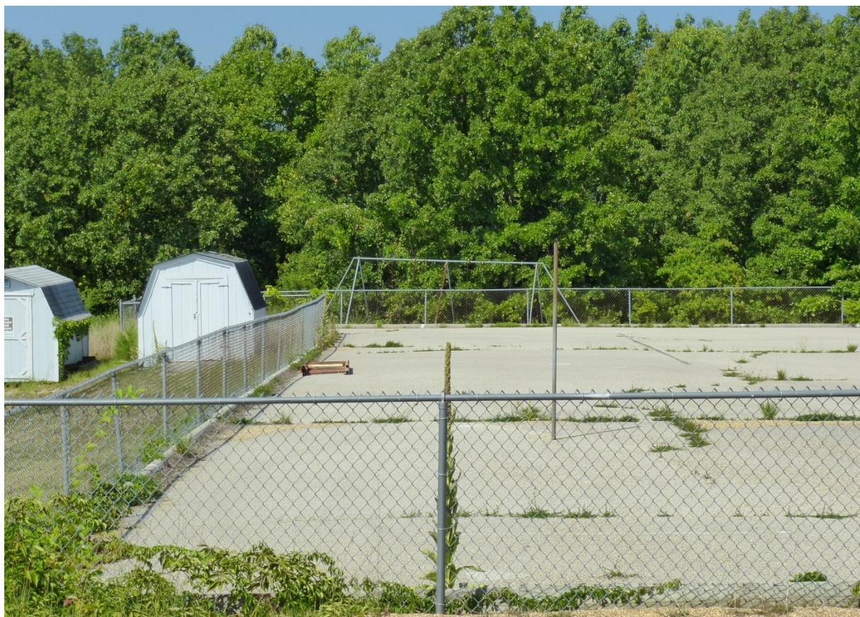
Photo 135. Paved playground on the west side of the school (ERDC-CERL, 2012).
