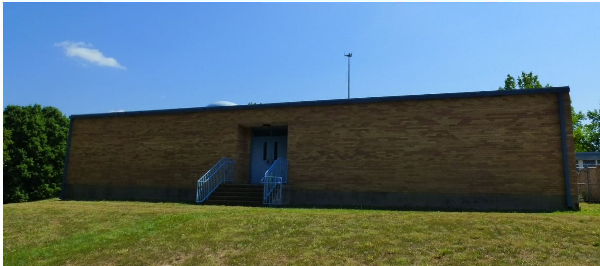
Photo 33. West elevation of 1984 addition (ERDC-CERL, 2012).
