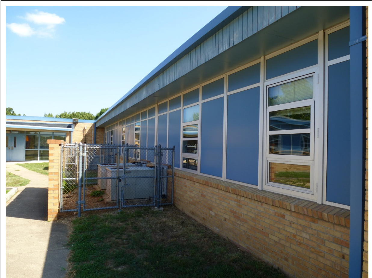
Photo 28. Modified window pattern on the far left side of original west elevation (ERDC-CERL, 2012).
