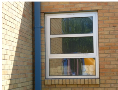
Replacement three-pane bright aluminum awning window.
