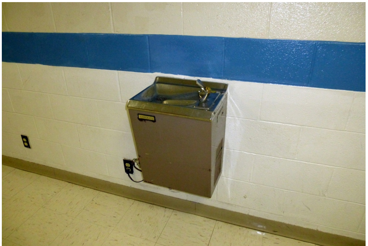
Photo 96. Replacement water fountain in original corridor (original school) (ERDC-CERL, 2012).
