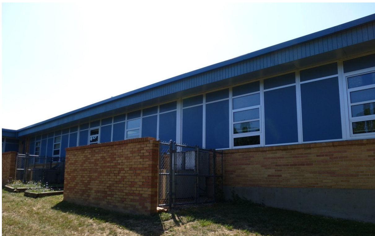
Photo 36. Right side of the north elevation with modified window pattern. Left side is 1957 addition and right side 1984 addition (ERDC-CERL, 2012).
