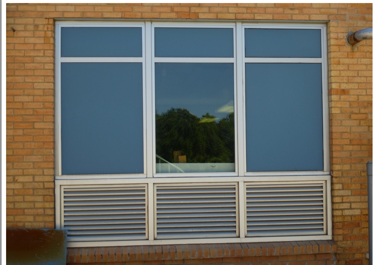
Photo 14. Closeup of replacement bright aluminum windows with metal louvered vents and panel inserts on the west elevation of the boiler room (ERDC-CERL, 2012).
