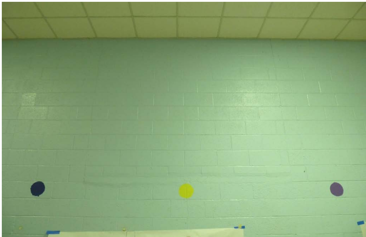
Photo 66. Looking toward east wall in multi-purpose room where the original windows were removed and the openings filled with concrete block (original school) (ERDC-CERL, 2012).
