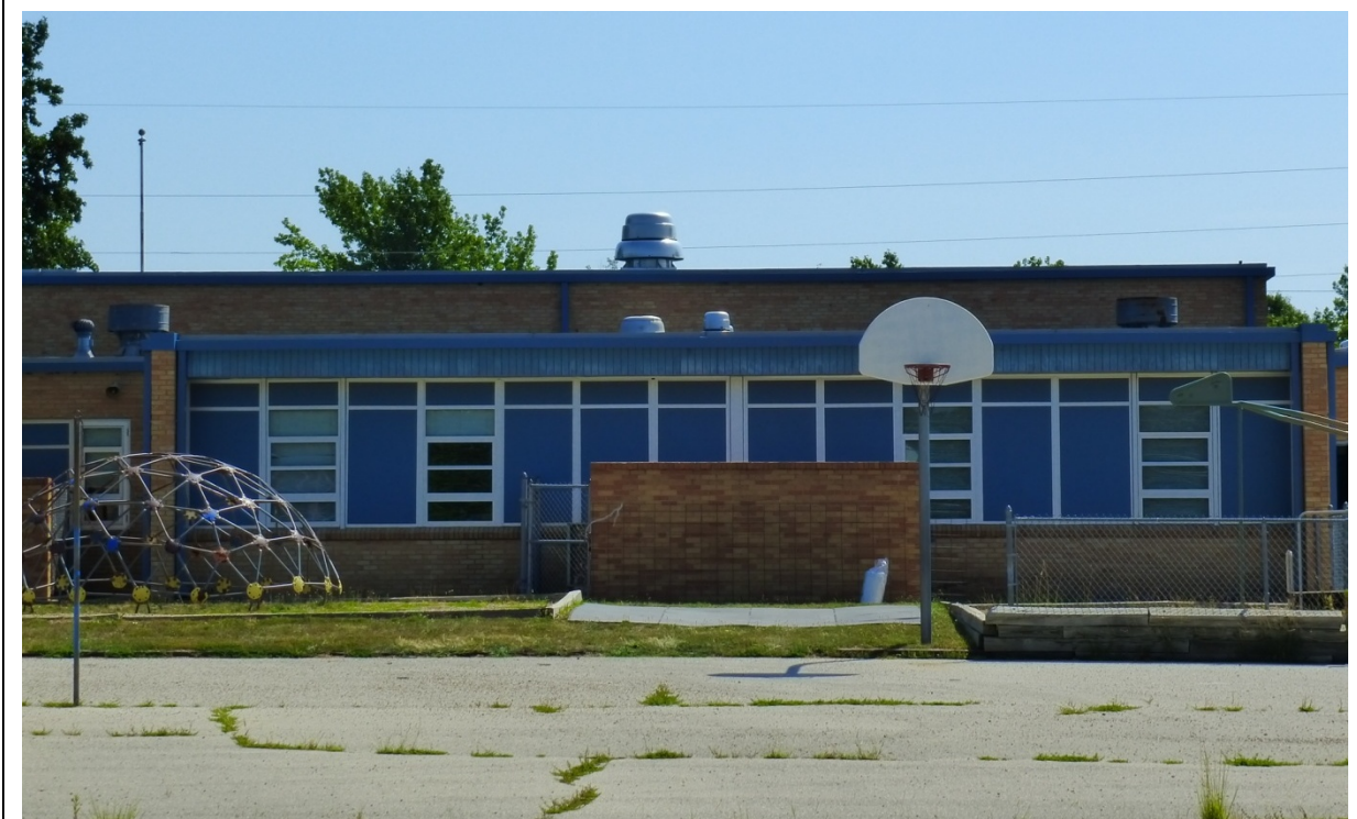
Photo 18. Modified window pattern with replacement bright aluminum windows and panel inserts on the right side of the west elevation of the original school portion (ERDC-CERL, 2012).
