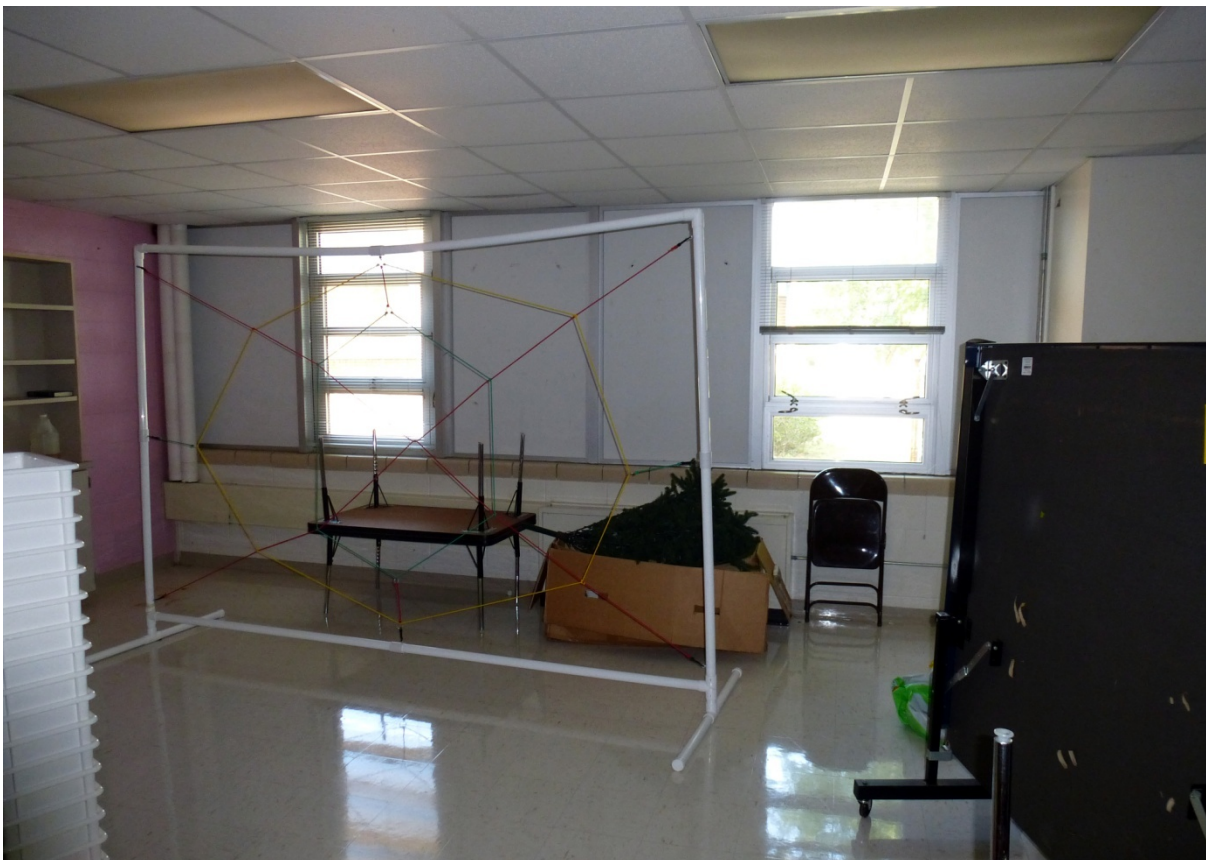
Photo 94. Interior of classroom looking at replacement windows, floors, and ceiling (original school) (ERDC-CERL, 2012).
