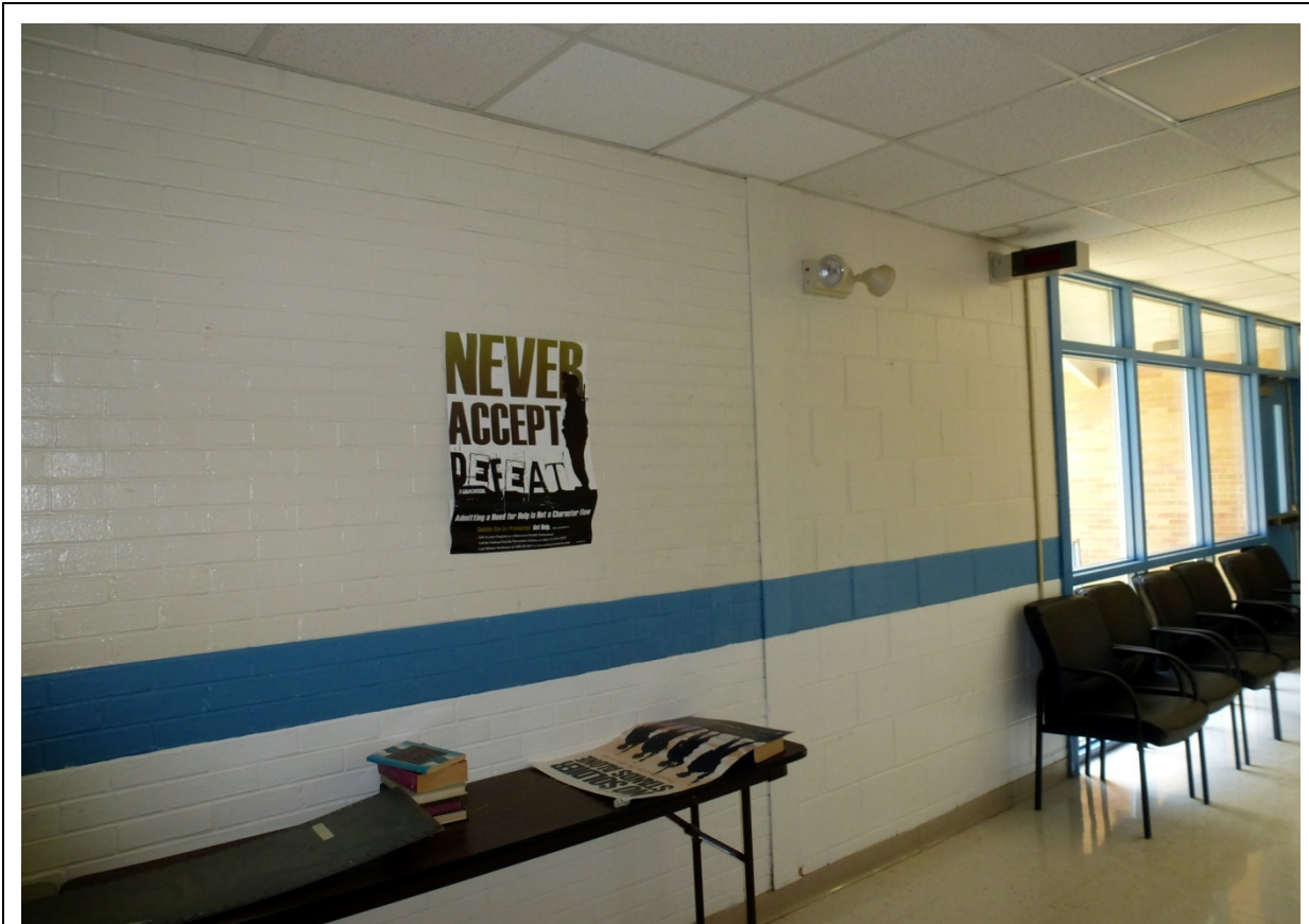
Photo 122. Looking at the original north exterior wall of original school on left connected to concrete block wall of the 1957 addition (ERDC-CERL, 2012).
