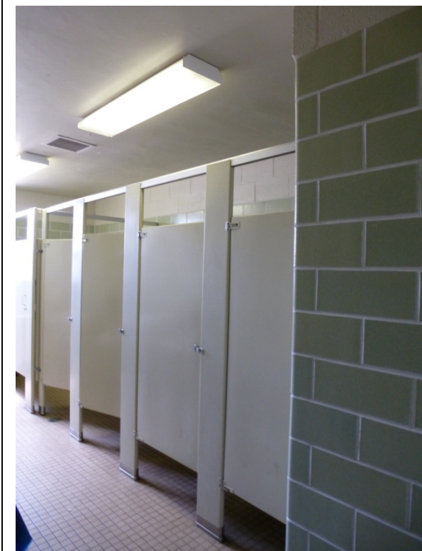
Photo 86. Girls' restroom with original glazed-tile walls (original school) (ERDC-CERL, 2012).
