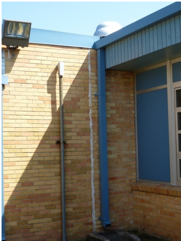
Photo 30. Close-up of connection between the original exterior wall on the west elevation (right side) and the brick wall of the 1957 addition (on the left) (ERDC-CERL, 2012).
