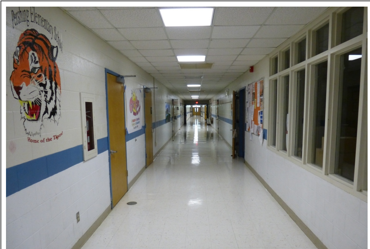
Photo 59. Looking north down original corridor toward addition (ERDC-CERL, 2012).
