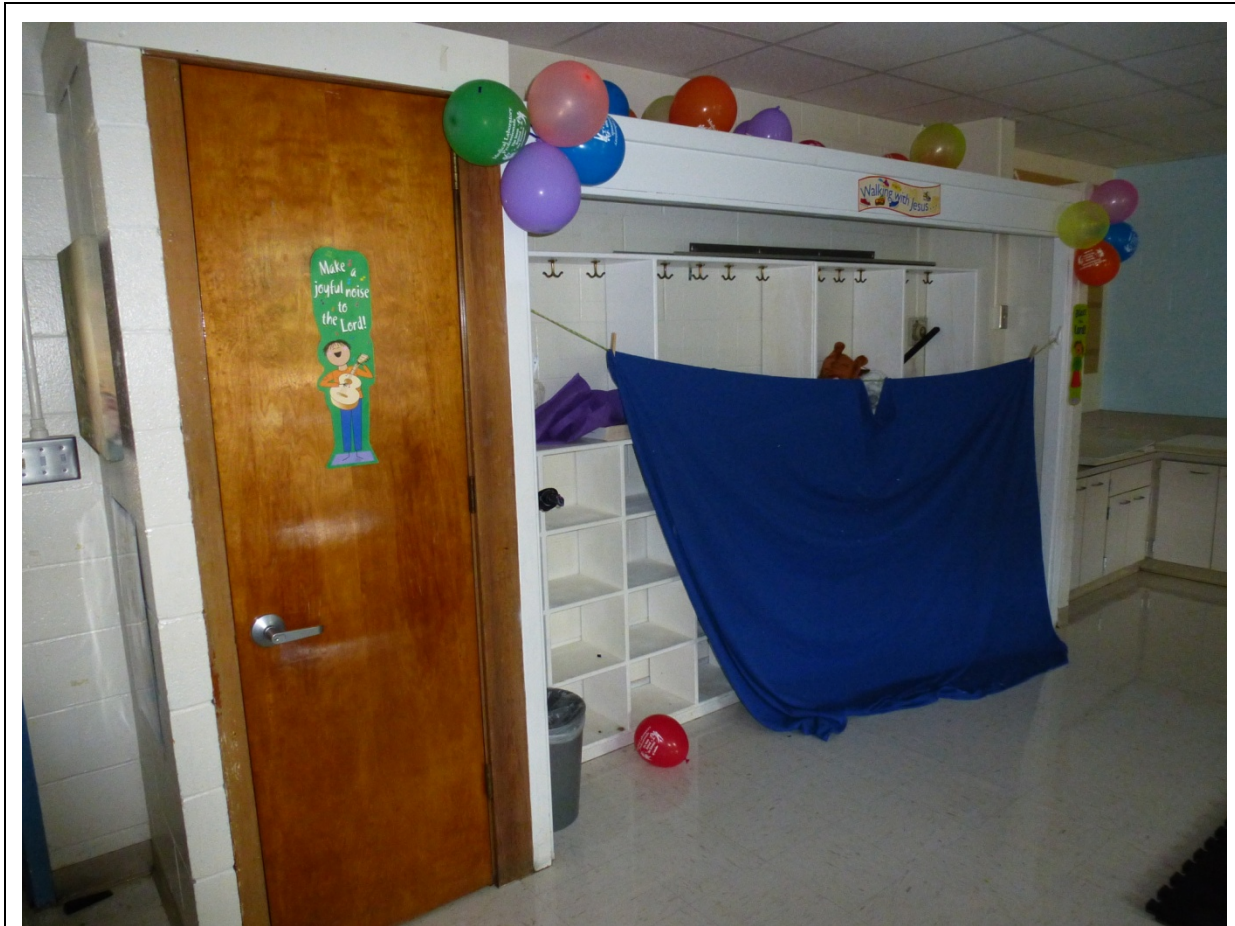
Photo 126. Wardrobe in classroom (1957 addition) (ERDC-CERL, 2012).
