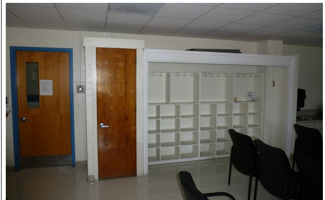
Photo 128. Wardrobe and closet door with replacement hardware in 1957 addition (ERDC-CERL, 2012).
