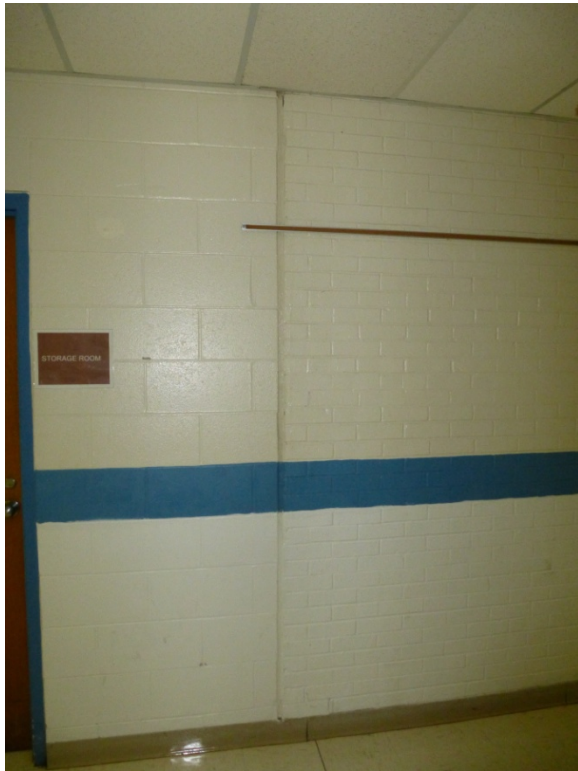
Photo 101. Closeup of connection between the original brick exterior wall and concrete block wall (1984 addition) (ERDC-CERL, 2012).
