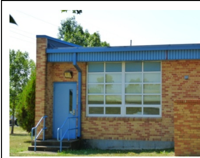
Original 1984 windows on addition.
