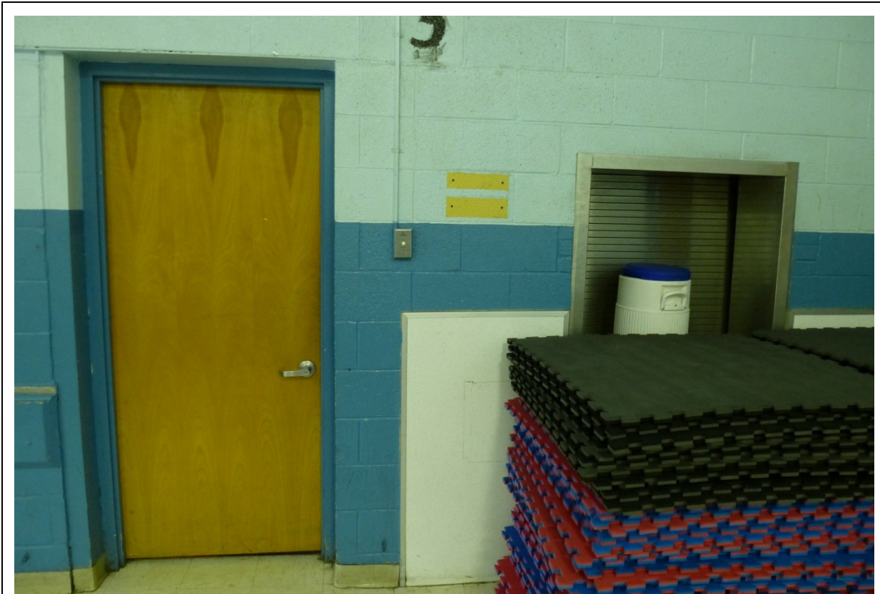
Photo 69. Replacement door leading into the kitchen (original school) (ERDC-CERL, 2012).
