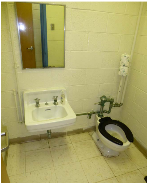
Photo 82. Original toilet room in between the two kindergarten rooms (original school) (ERDC-CERL, 2012).
