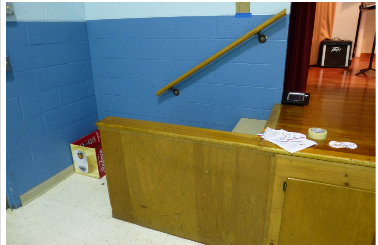
Photo 62. Stage steps (original school) (ERDC-CERL, 2012).
