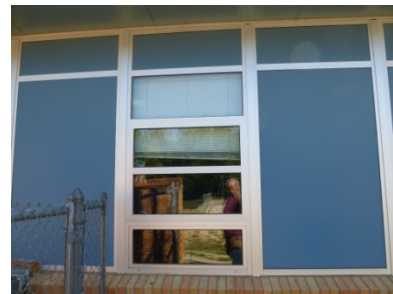
Replacement bright aluminum awning window with porcelain enamel metal panel.
