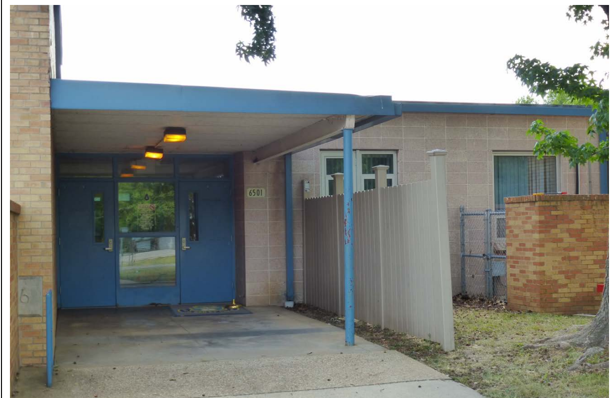
Photo 2. Replacement entry doors and sidelight of the main entry on the east elevation (ERDC-CERL, 2012).
