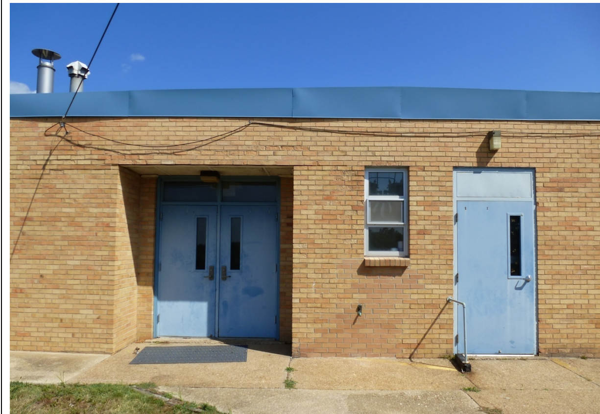
Photo 10. Replacement entry doors and replacement window on the south elevation (ERDC-CERL, 2012).
