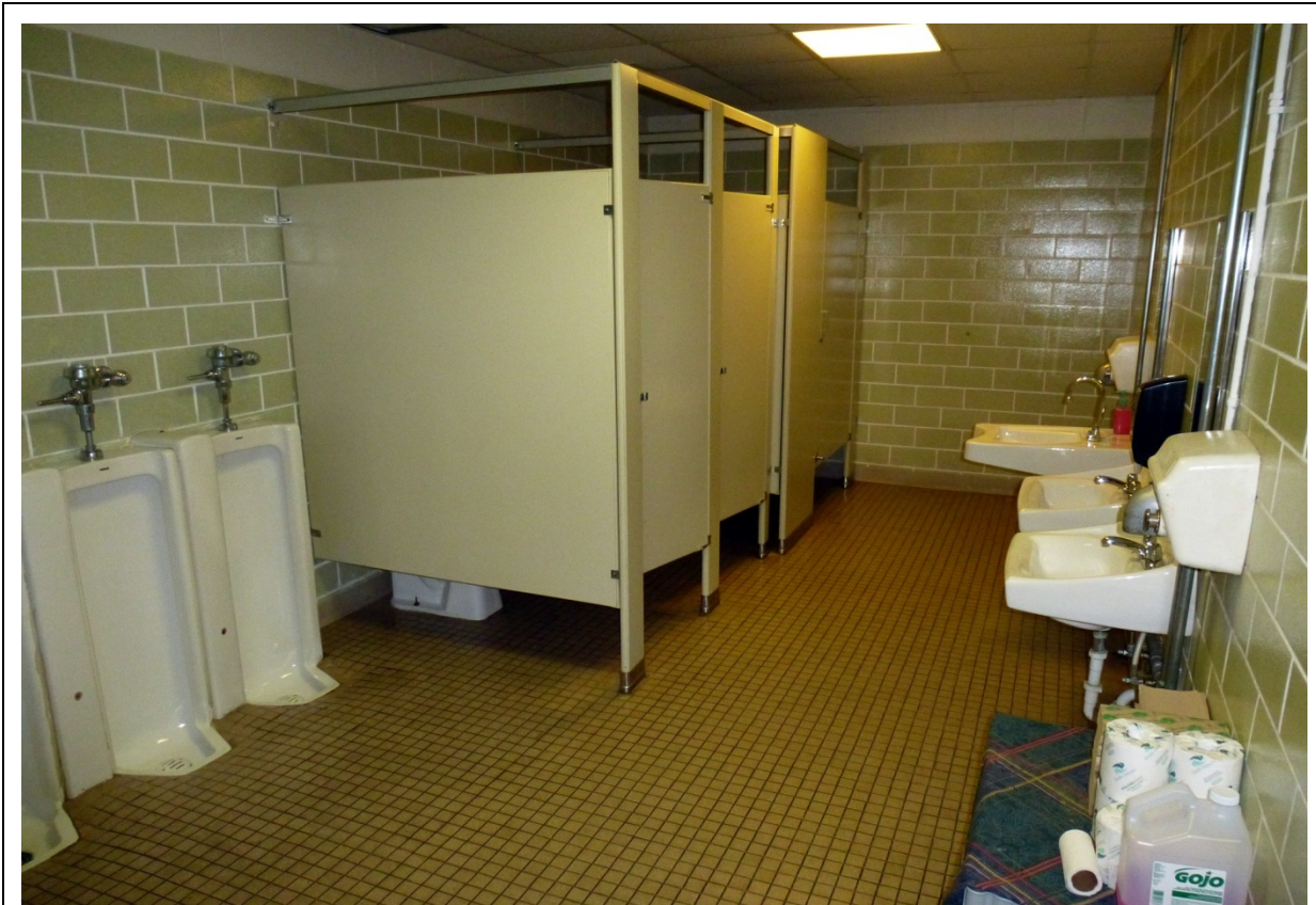
Photo 118. Boys' restroom with original urinals and glazed-tile walls (1957 addition) (ERDC-CERL, 2012).
