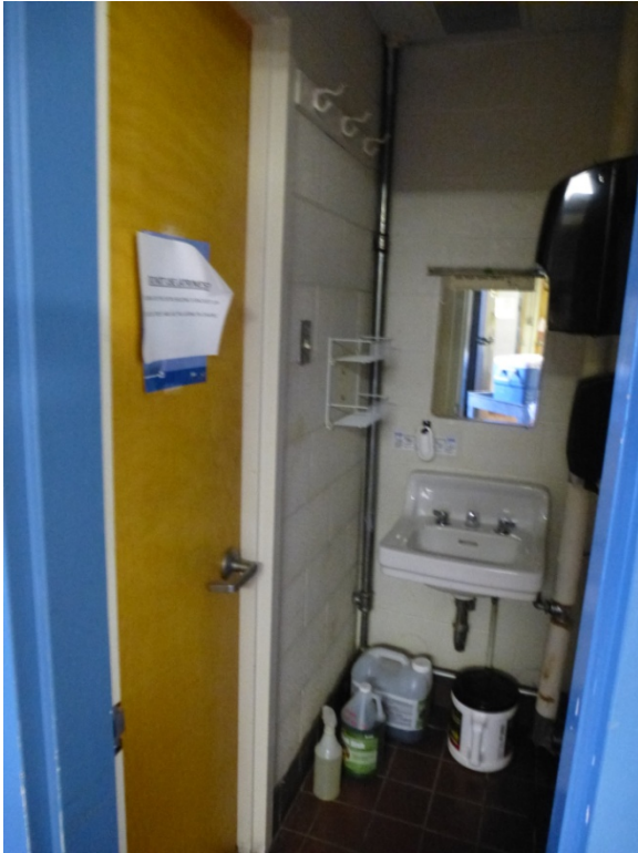
Photo 73. Original toilet room off of kitchen with replacement sink (original school) (ERDC-CERL, 2012).
