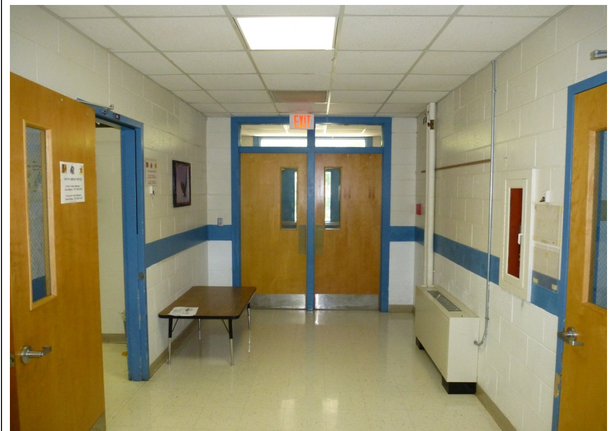
Photo 111. Replacement vestibule doors at the north end of the 1984 addition (ERDC-CERL, 2012).
