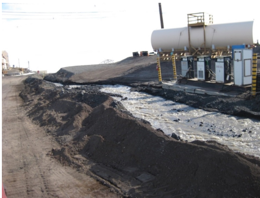
Figure 3. Along the Gasoline Alley drainage channel adjacent to the fuelling station (photo by Lynette Barna, CRREL, 19 December 2010).
