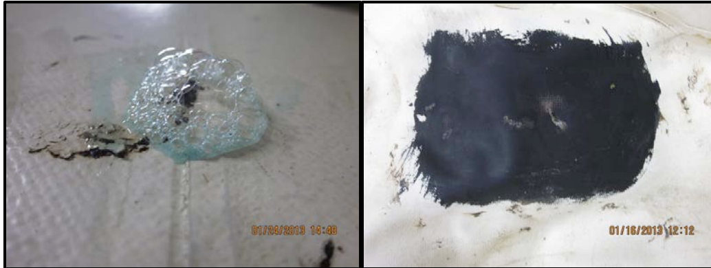
Figure 6. Bubbles forming above a small leak in a thumbnail-sized arc (left), and 2 large gouges at the center of a section prepared for patching (right). The gouges on the right are each approximately the size of a quarter, and the entire prepared area is approximately 8 × 6 in.
